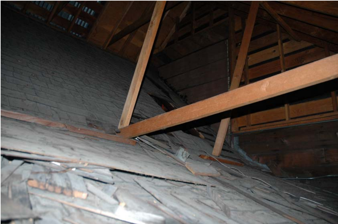
Original roof, single story portion
