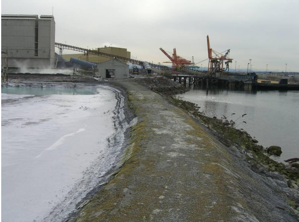
Photo 3: Waterfront at Edge of Secondary Settling Pond – from the northwest
