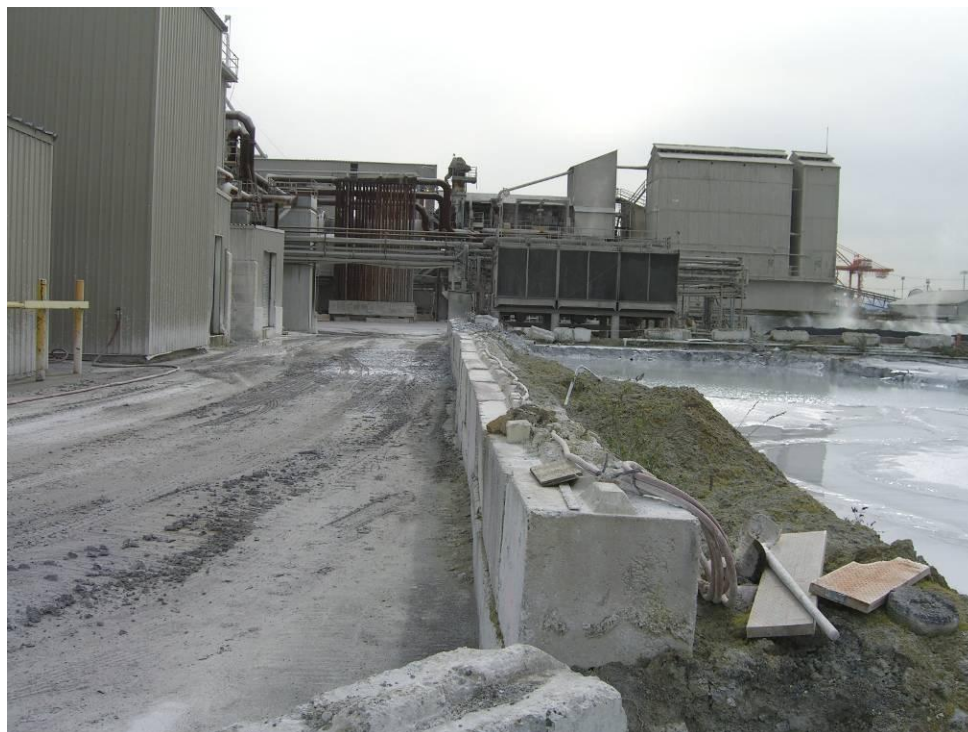
Photo 2: Original Restrictive Covenant Area – from the northwest
