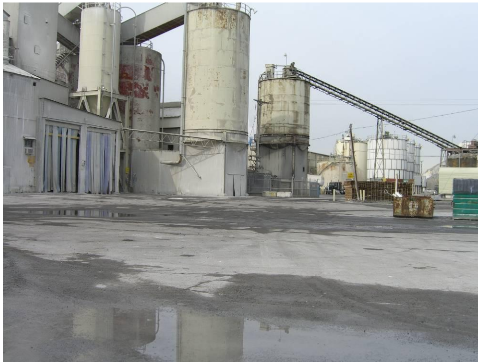
Photo 1: Main Plant – from the east
