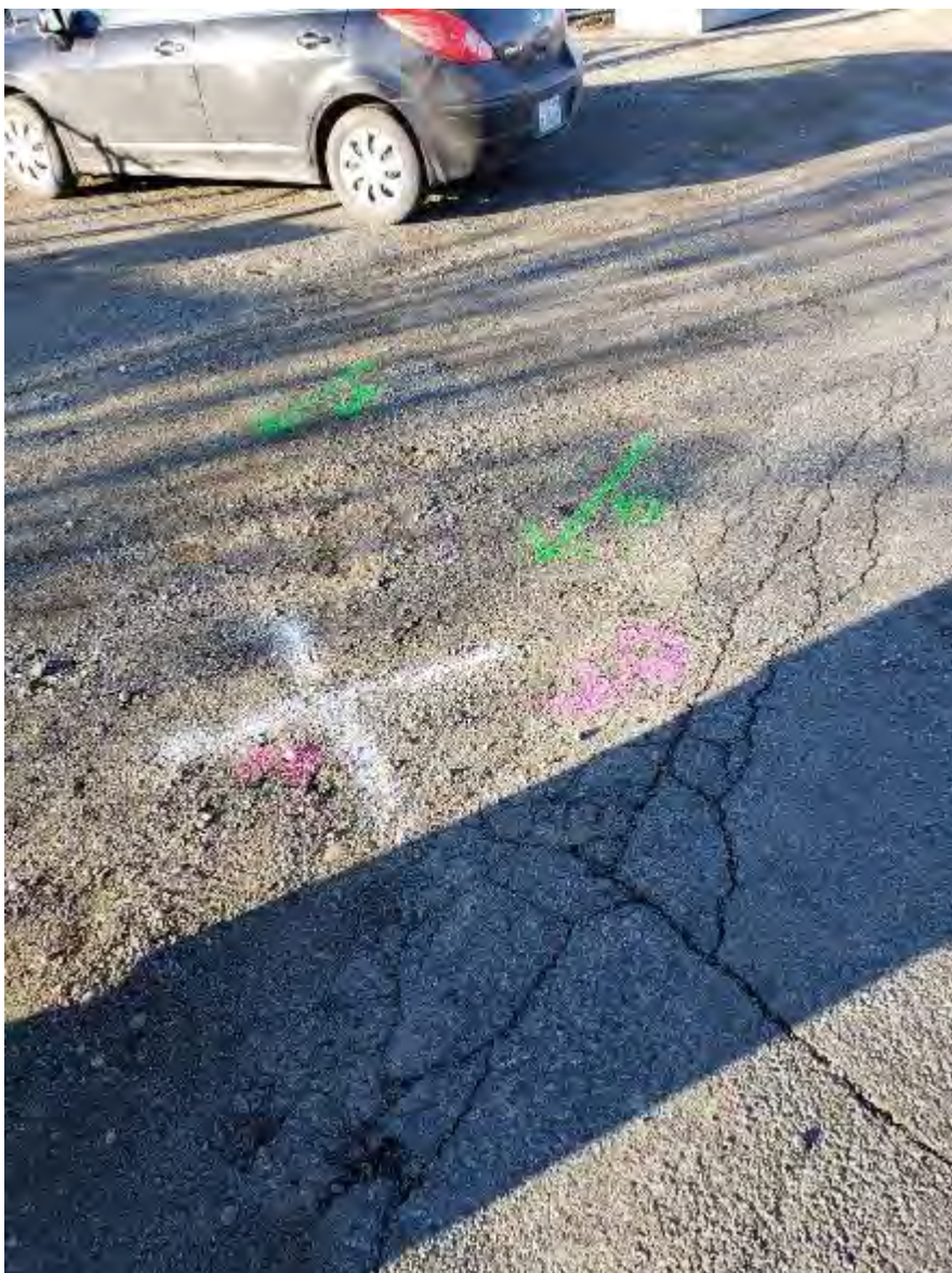
Photo 15. Initial location for BH2-16 with utilities marked.
