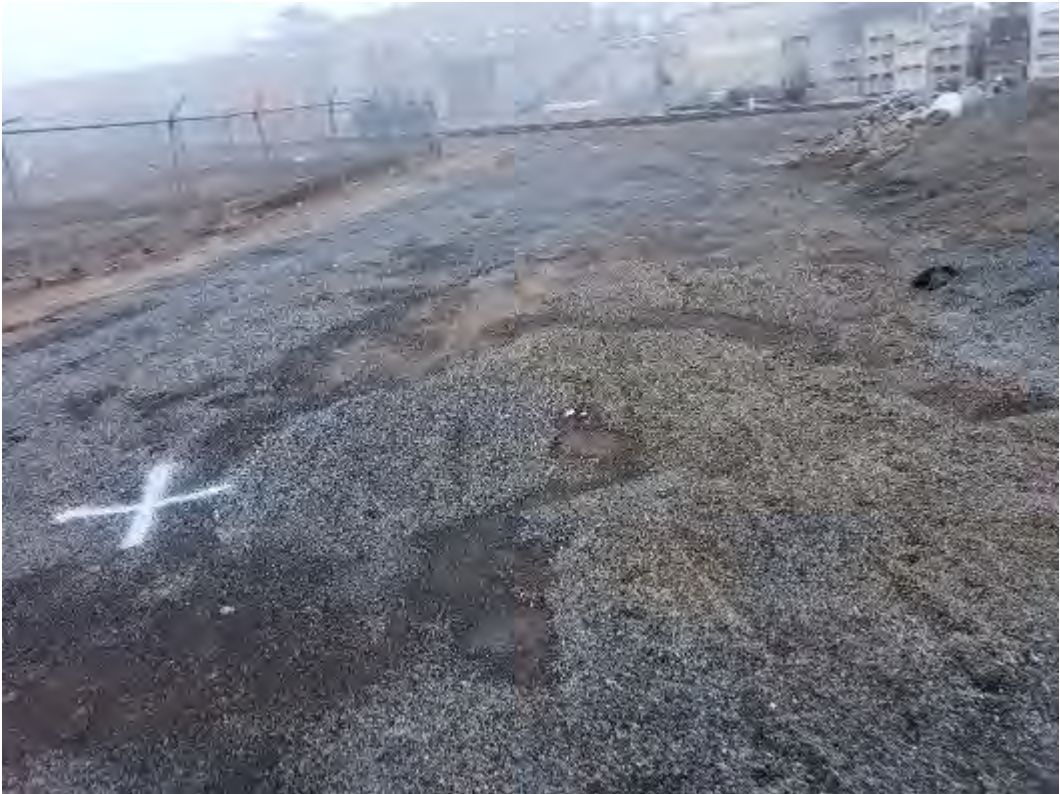
Photo 14. New locations for BH2-12 and BH2-13.
