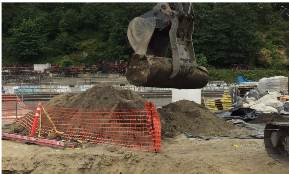
Photograph 5 Removal of UST.
