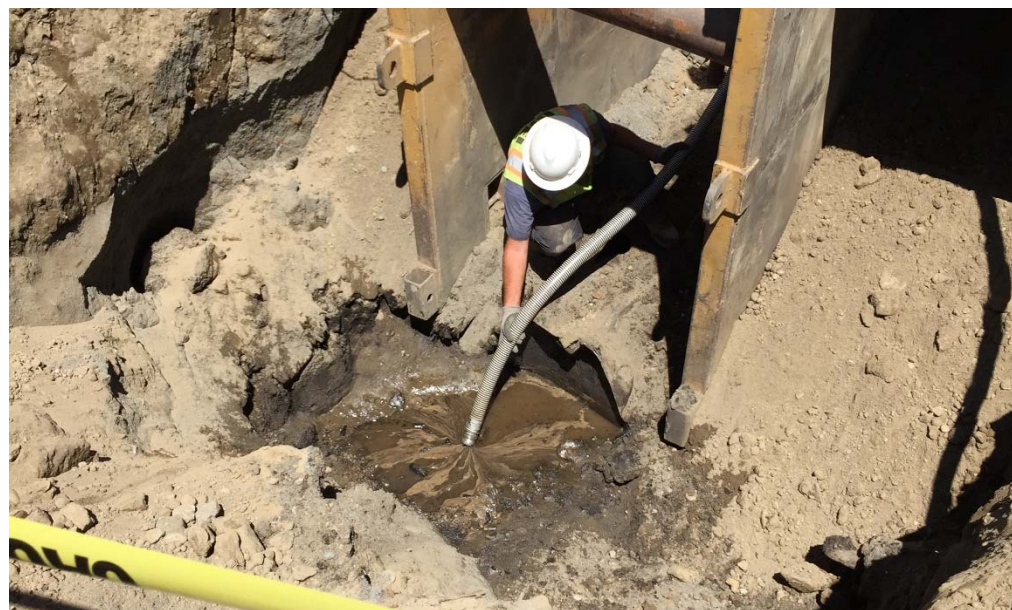
Photograph 2 Removal of fluid from inside and around the tank.
