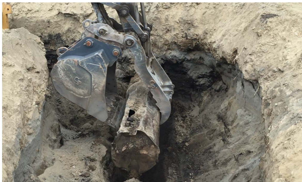
Photograph 4 UST being removed from trenching excavation area.
