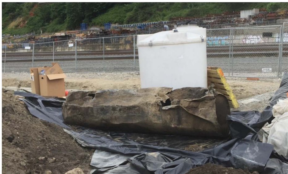
Photograph 6 UST placed on plastic for storage until removal from site.
