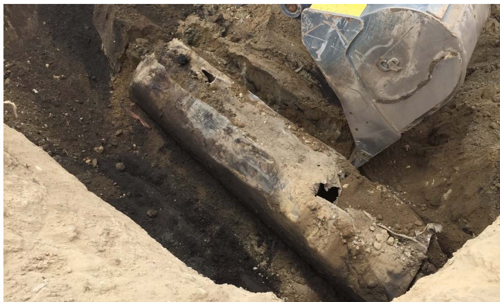
Photograph 3 Removing soils around UST to allow for extraction.
