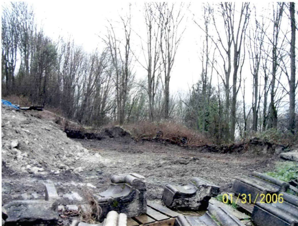
Photograph #11 – Completed removal of the east half of the pile.
