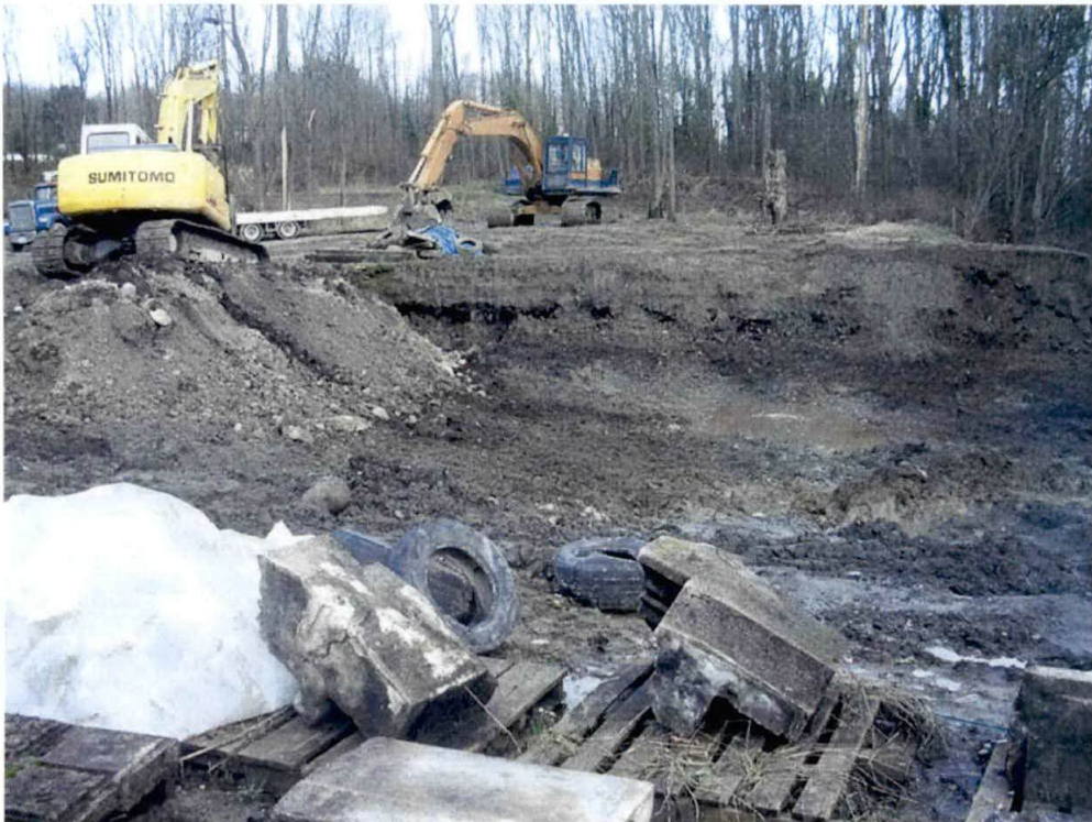
Photograph #18 - 2/2/2006- View of the north and south boundaries of excavation pit.
