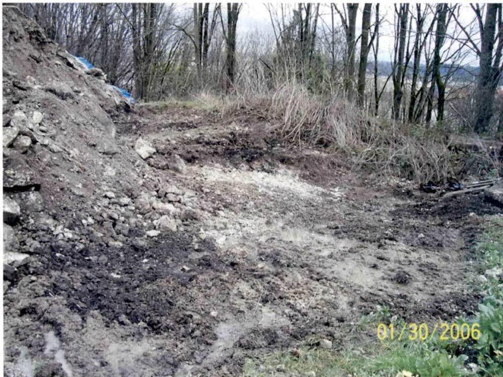
Photograph #8 – Removal of the east side of the pile.
