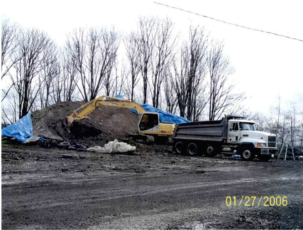
Photograph #5 – Further removal of pile.
