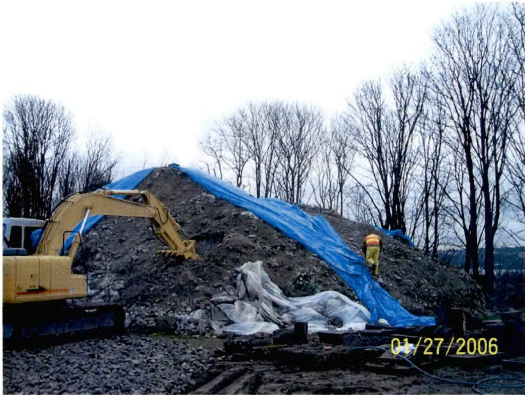
Photograph #3 – Taking tarp off pile for access.
