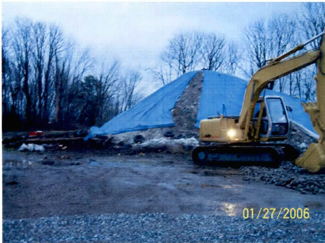
Photograph #2 – Initial pile during removal of unrelated debris pile.
