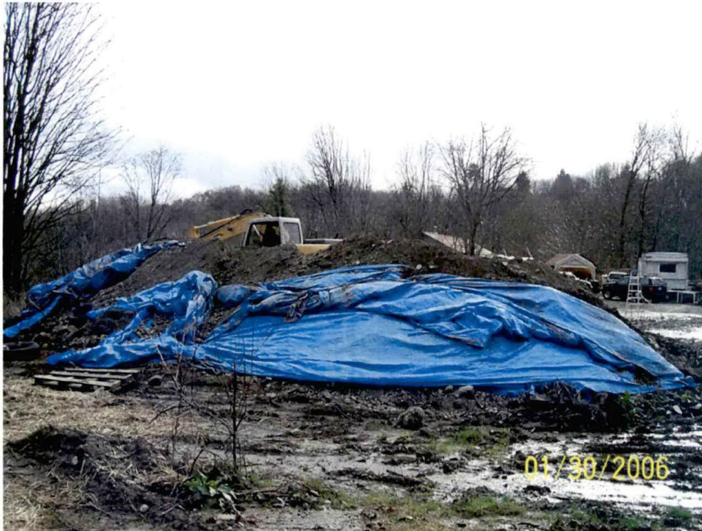
Photograph #7 – Side view of pile
