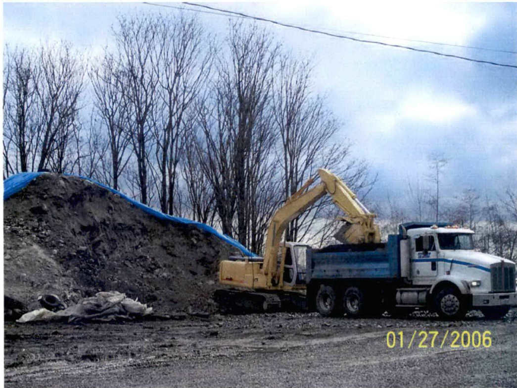
Photograph #4 – View of dump trucks and excavator and removal of pile.
