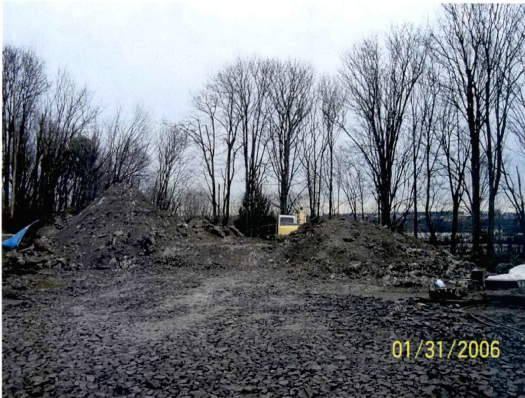
Photograph # 9 – Further removal.
