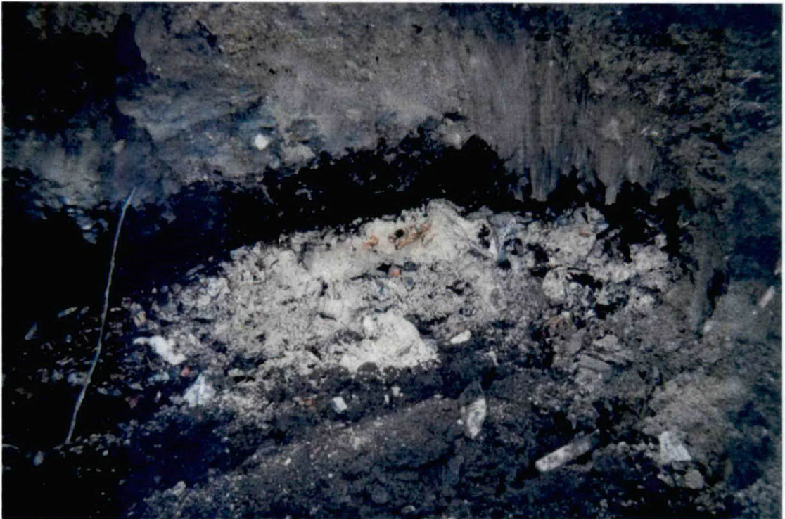
Photograph #10 – Further removal of material.
