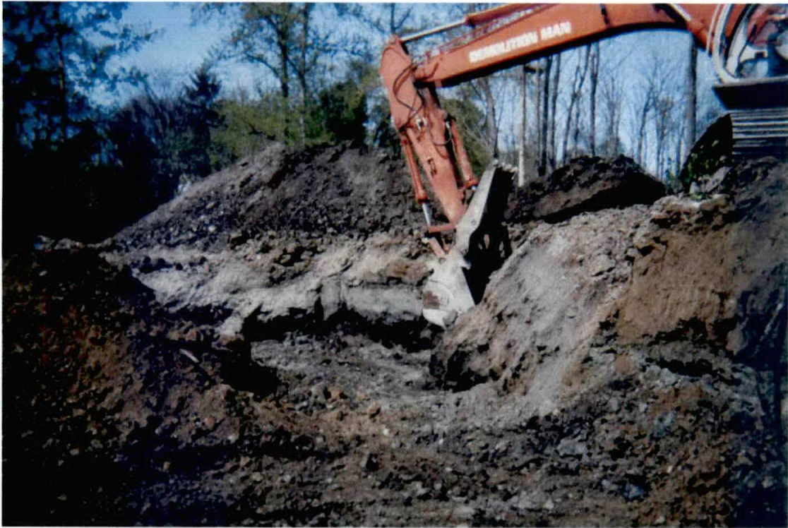
Photograph #9 – View during excavation of battery casing material.
