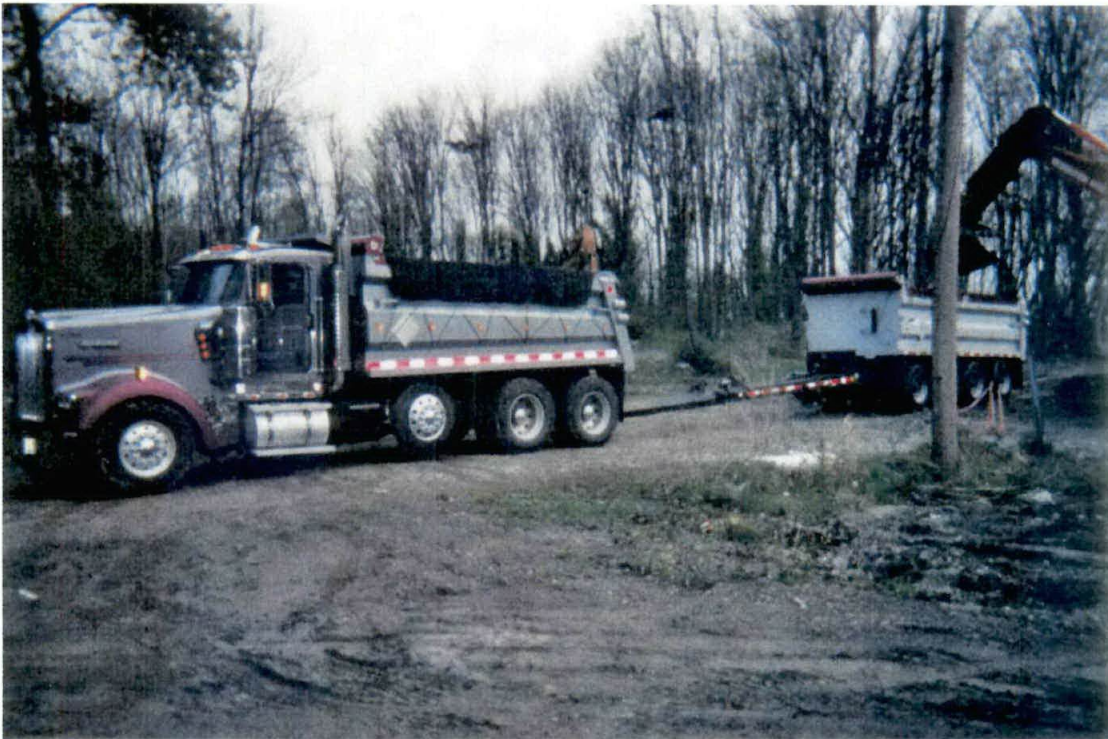
Photograph #12 – Trucks used to haul excavated battery casing material.
