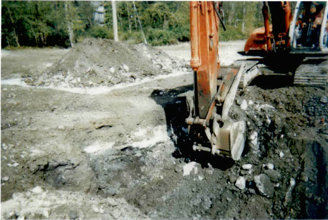
Photograph #9 – Further removal.
