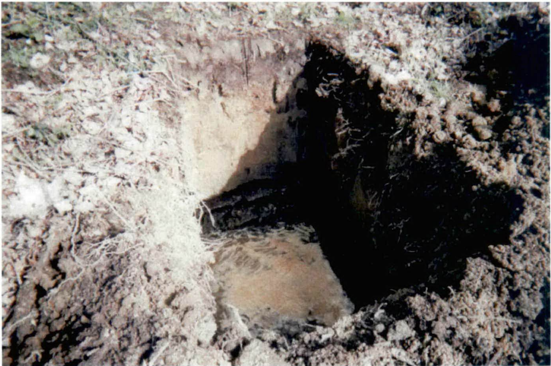
Photograph #4 – View of TP-8 showing groundwater encountered.
