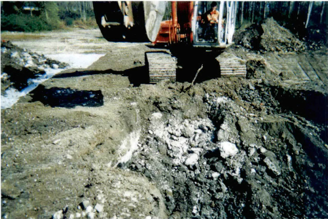
Photograph #8 – Further removal of CKD material.
