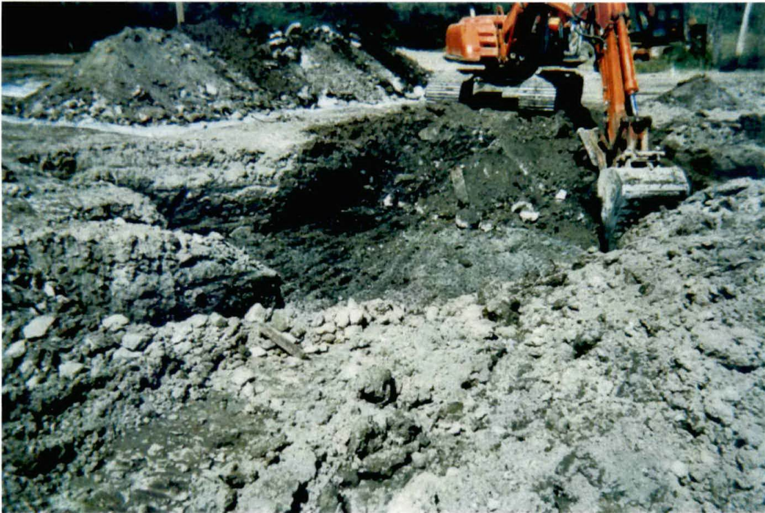
Photograph #10 – View of CKD excavation nearly completed.
