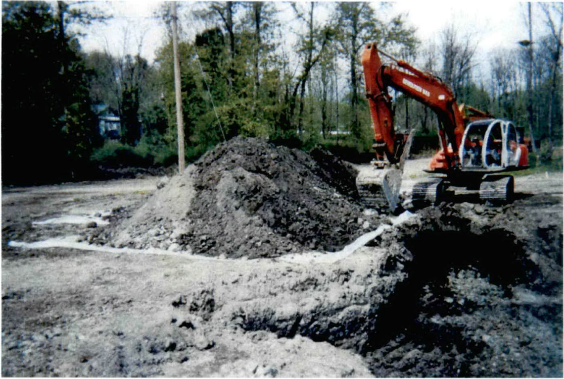
Photograph #11 – Excavation completed of the CKD material.
