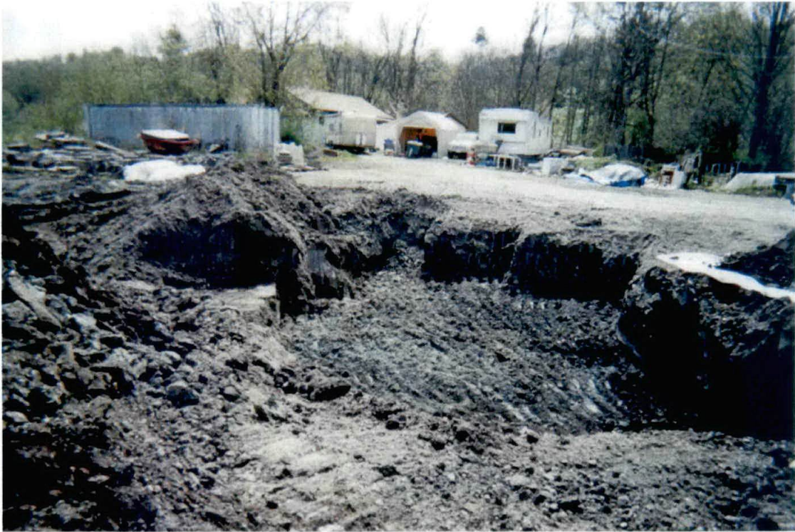
Photograph #15 – View of excavation area looking south.
