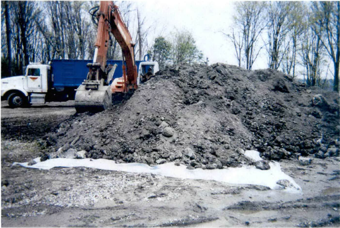
Photograph #17 – View of excavated CKD material being removed.
