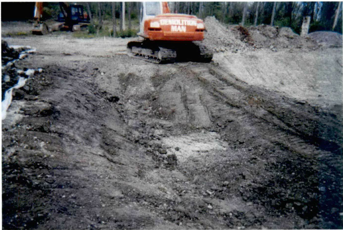
Photograph #16 – View excavated area after grading to reduce erosion.
