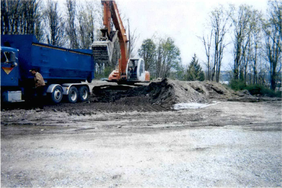
Photograph #19 – Further removal.
