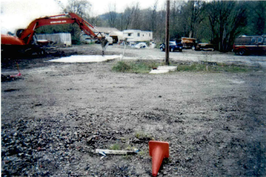
Photograph #6 – View during excavation of CKD material onto plastic sheeting.
