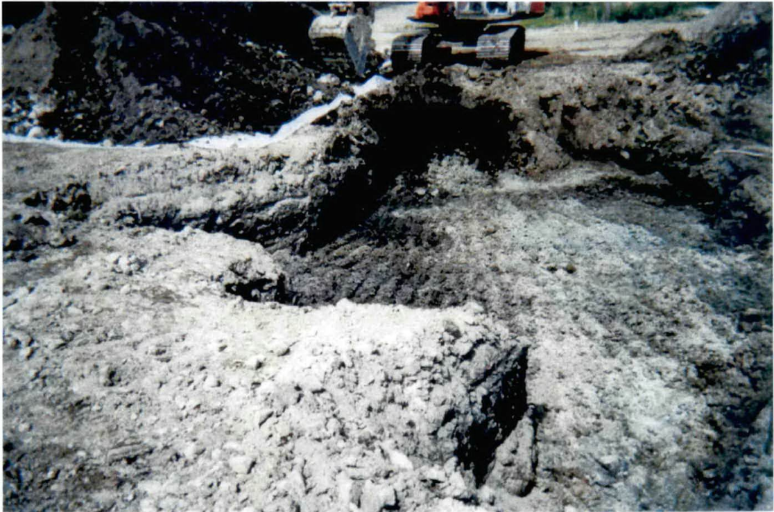
Photograph #14 – View of excavation area looking north.
