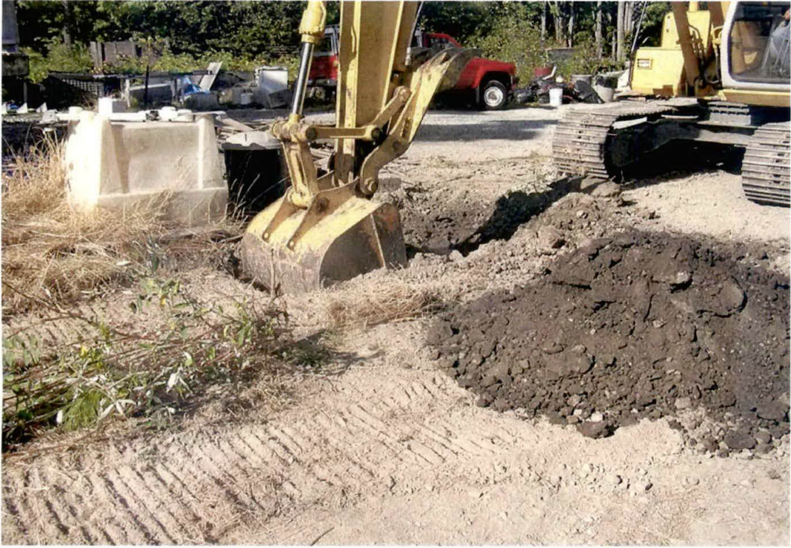
View of the digging of test pit TP-20
