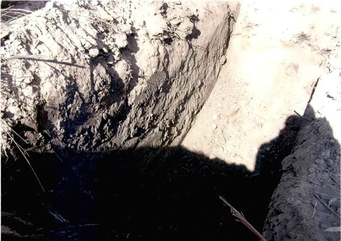
View of inside of test pit TP-20
