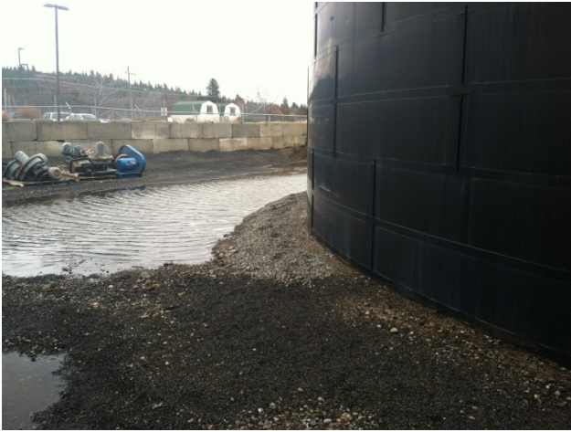
Photo 5 – North of Sample Location No. 2, View Looking Southeast
