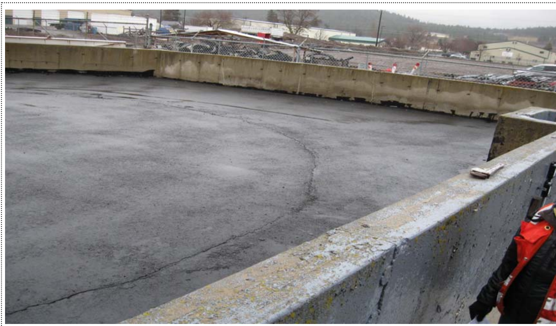
Photograph 2 – View of Northeast Tank Farm looking toward East Wall (February 2011).
