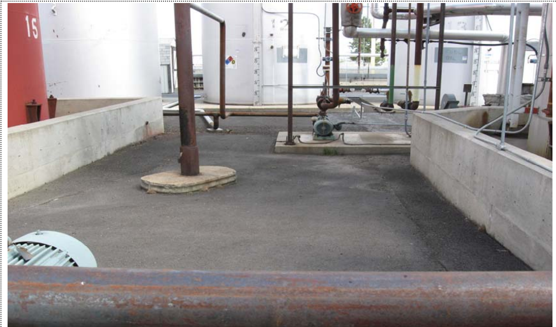
Photograph 4 – View of Northeast Tank Farm Interior (May 2011).
