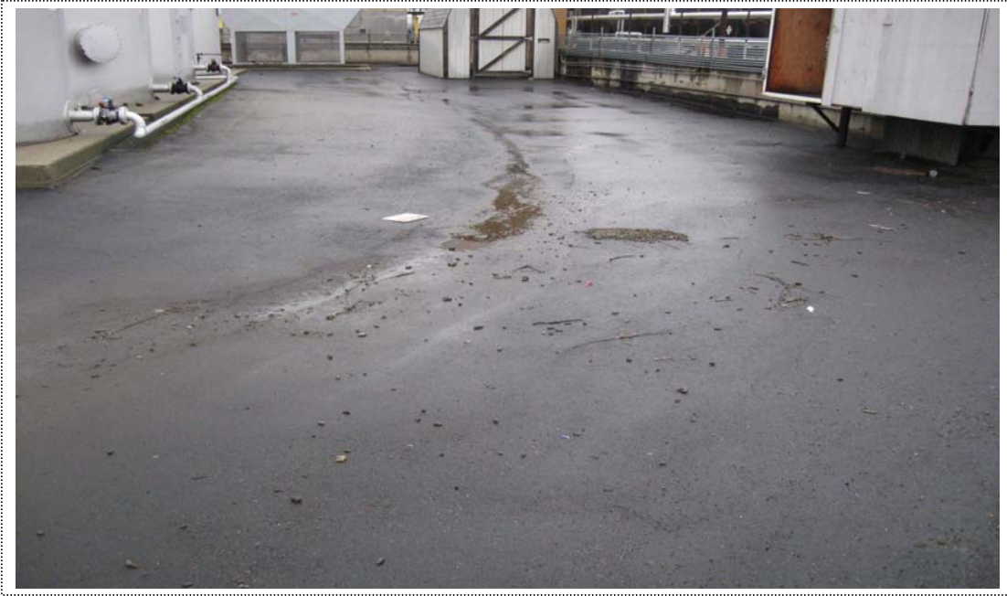
Photograph 3 – View of Northeast Tank Farm Interior (February 2011).
