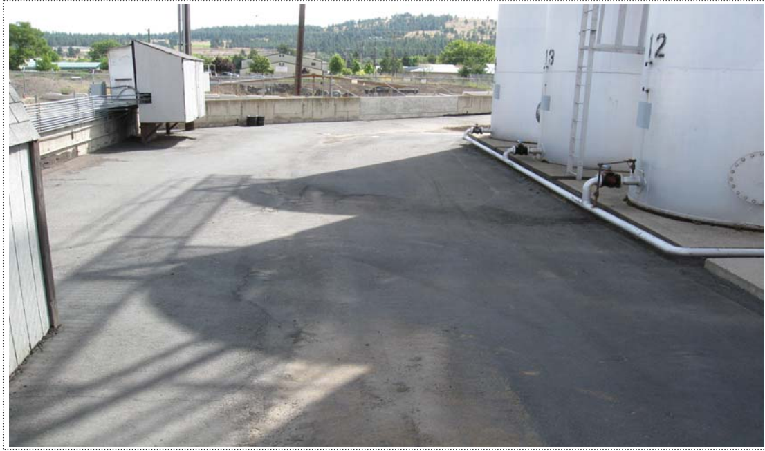
Photograph 5 – View of Northeast Tank Farm towards Northeast Wall (May 2011).
