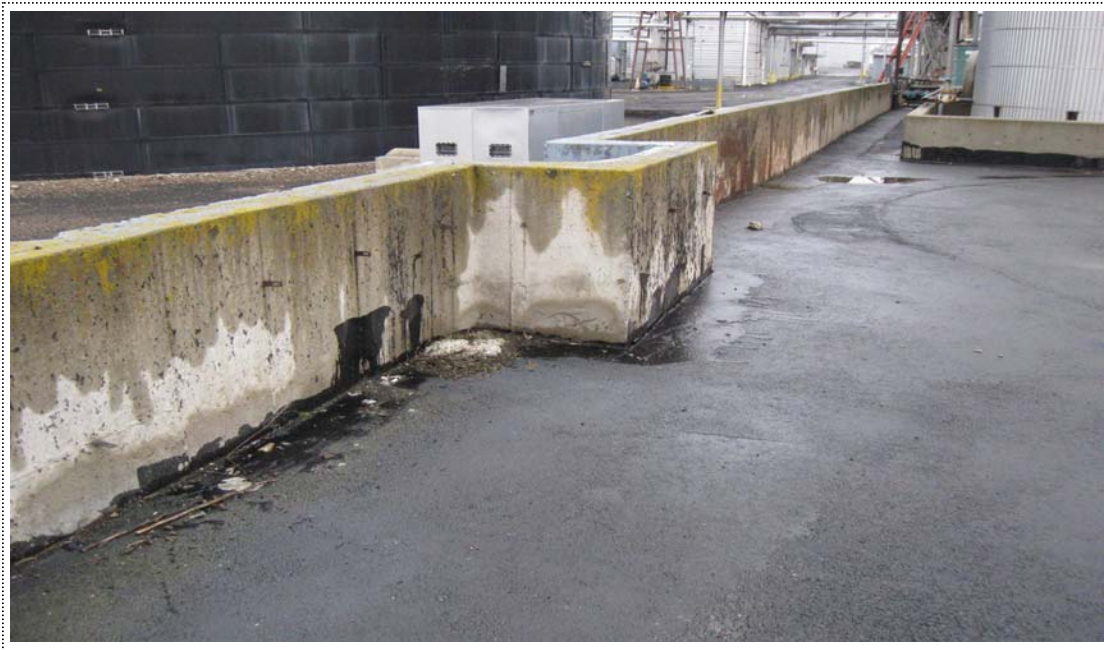
Photograph 1 – View of Northeast Tank Farm along South Exterior Wall (February 2011).
