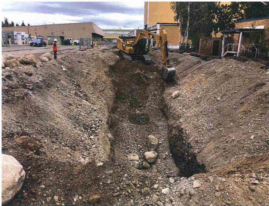
Photograph 10. SES excavates PCS from beneath Bay-3 and Bay-4 areas, looking North.
