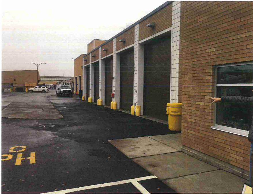
Photograph 1. Outside Avista Spokane Service Center pre-demo, looking north.
