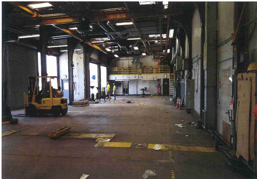
Photograph 2. Inside Avista Spokane Service Center pre-demo, looking north.
