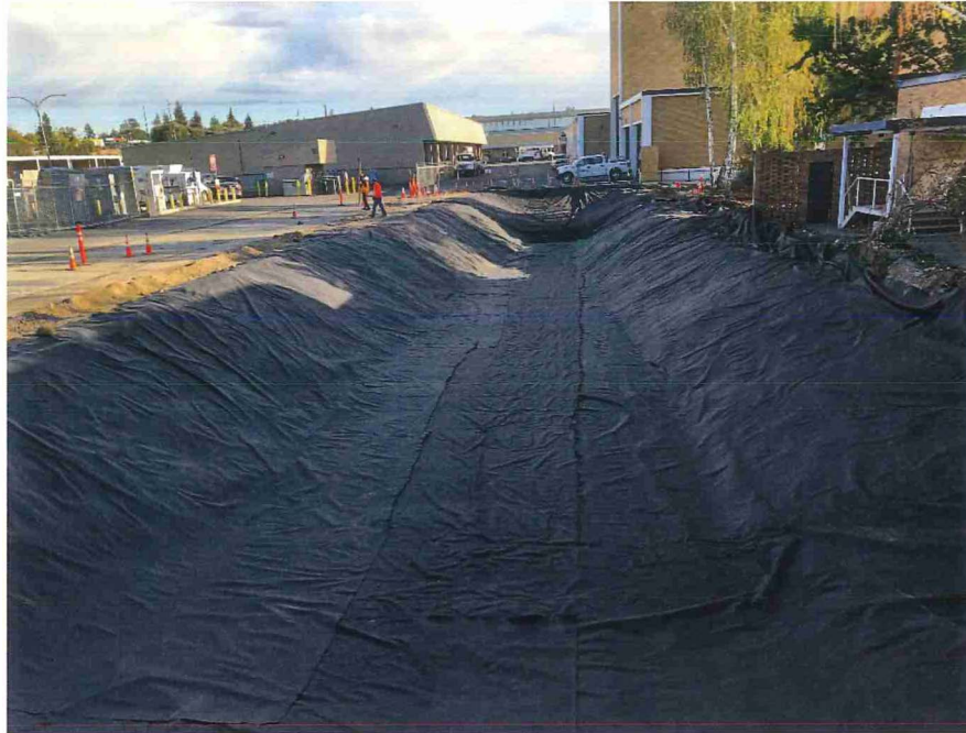
Photograph 17. SES places geotextile fabric over bedding sand in excavation, looking North.
