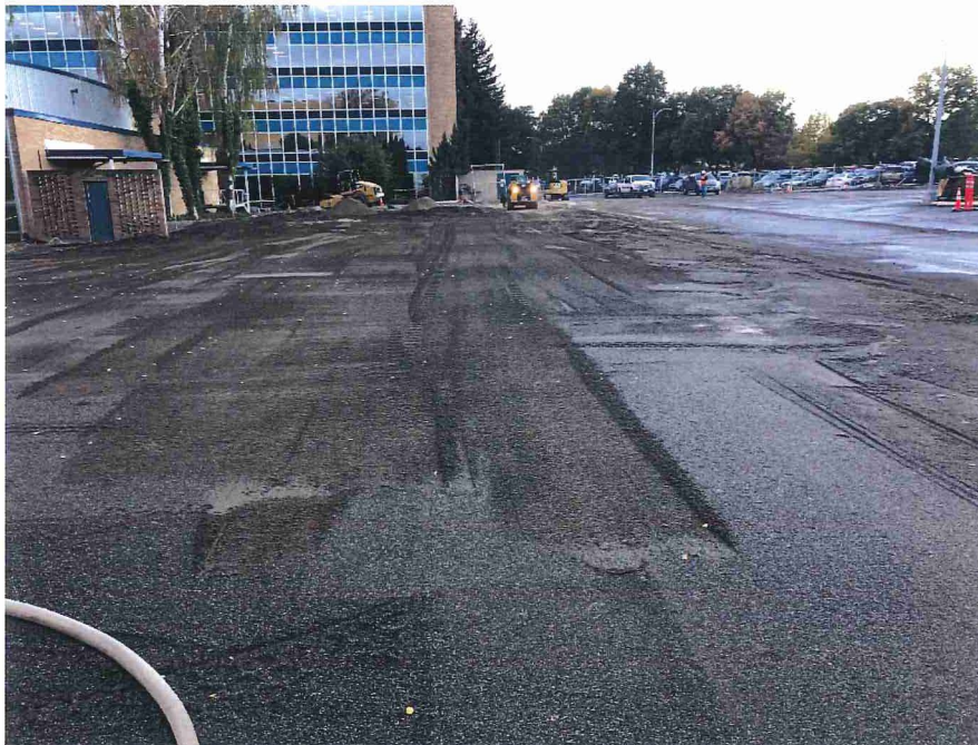
Photograph 28. Excavation backfilled and compacted, looking South.
