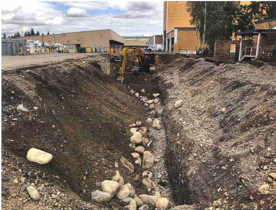
Photograph 14. SES shapes the west sidewall of the excavation, looking North.
