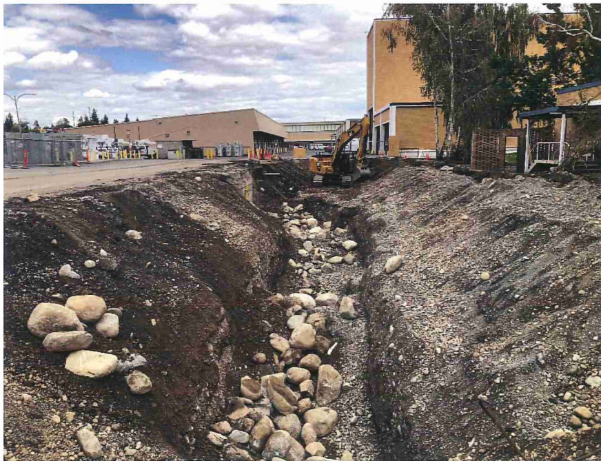
Photograph 12. SES places boulders from excavation into base of excavation.
