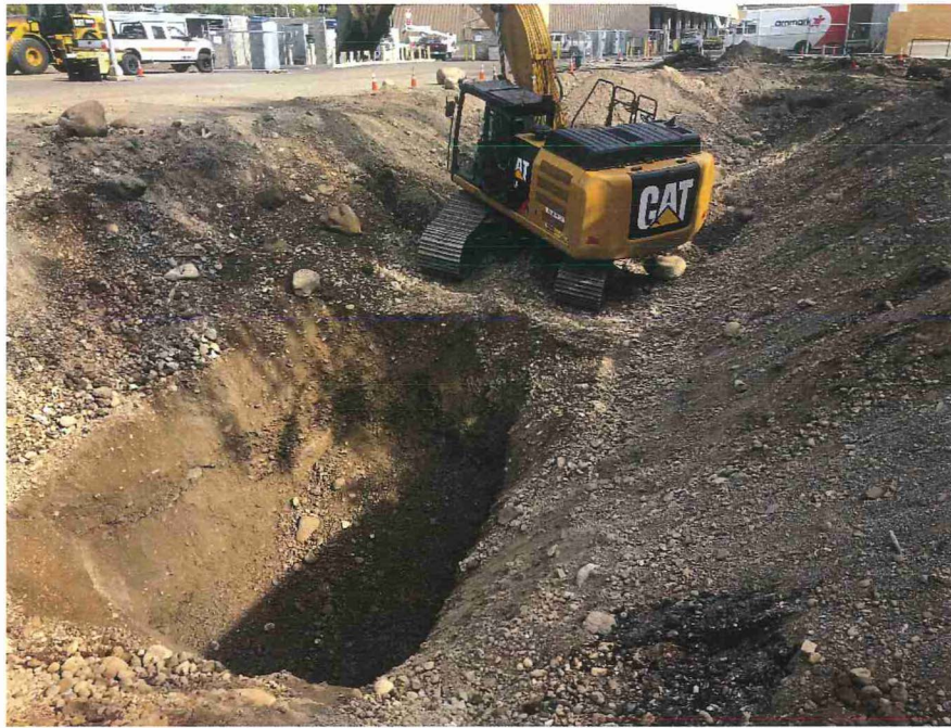
Photograph 9. SES excavates PCS from beneath Bay-1 and Bay-2 areas, looking North.
