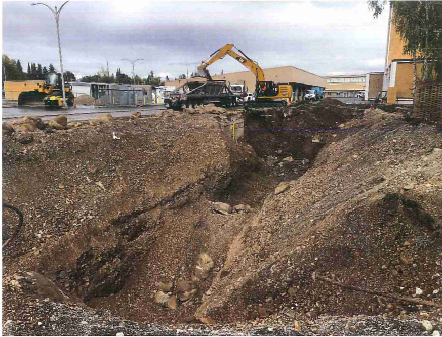
Photograph 11. SES excavates PCS from beneath Bay-5 area, looking North.
