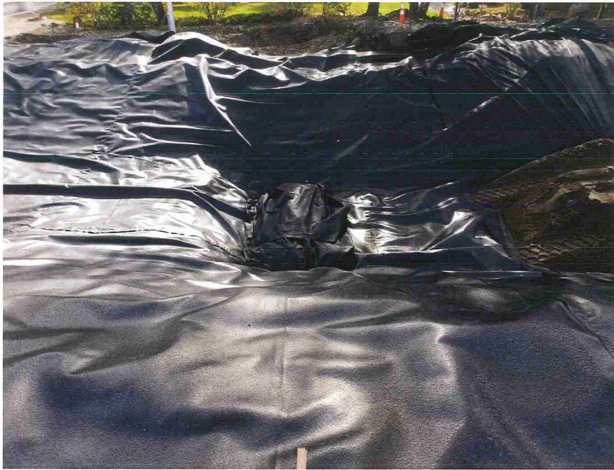
Photograph 25. Completed liner drain wrapped in geotextile fabric, looking East.
