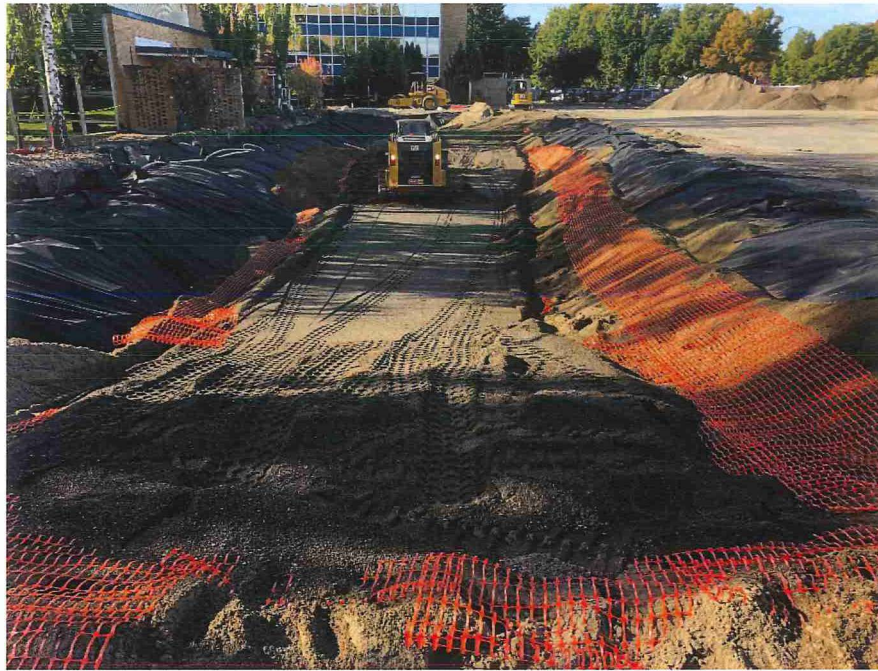
Photograph 27. Excavation backfill, looking South.
