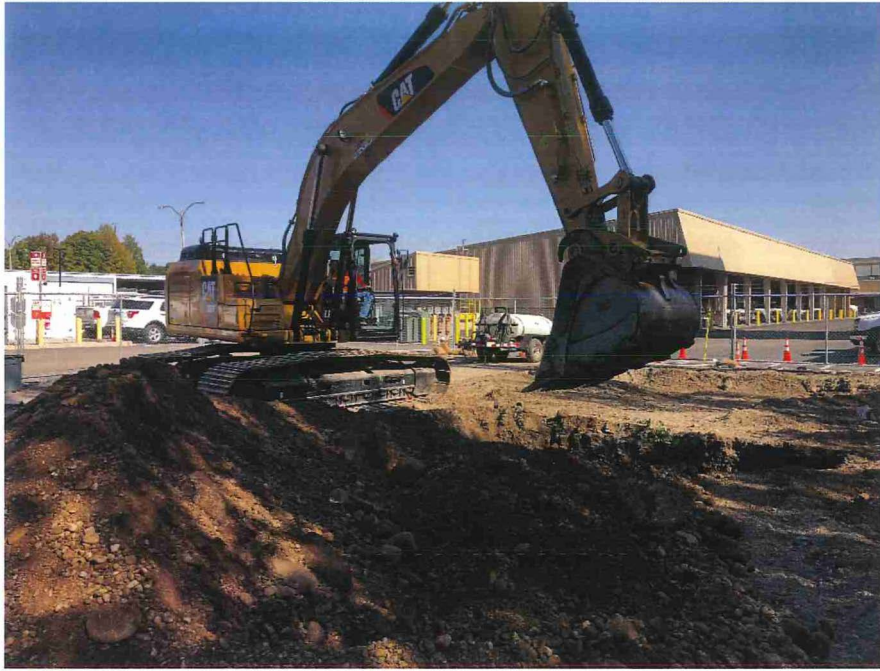
Photograph 5. SES excavates test pit TP-1 in highbay area, looking northwest.
