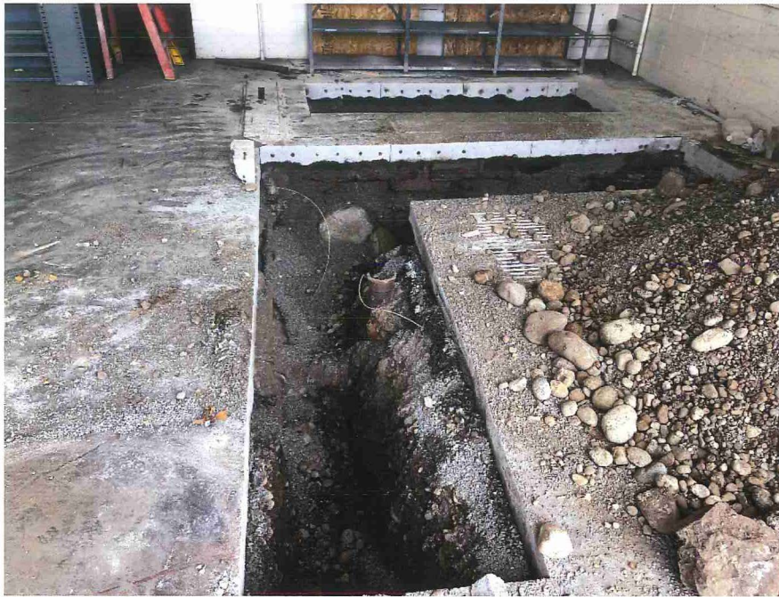
Photograph 3. Sawcut test pit in Bay-7. Looking East.
