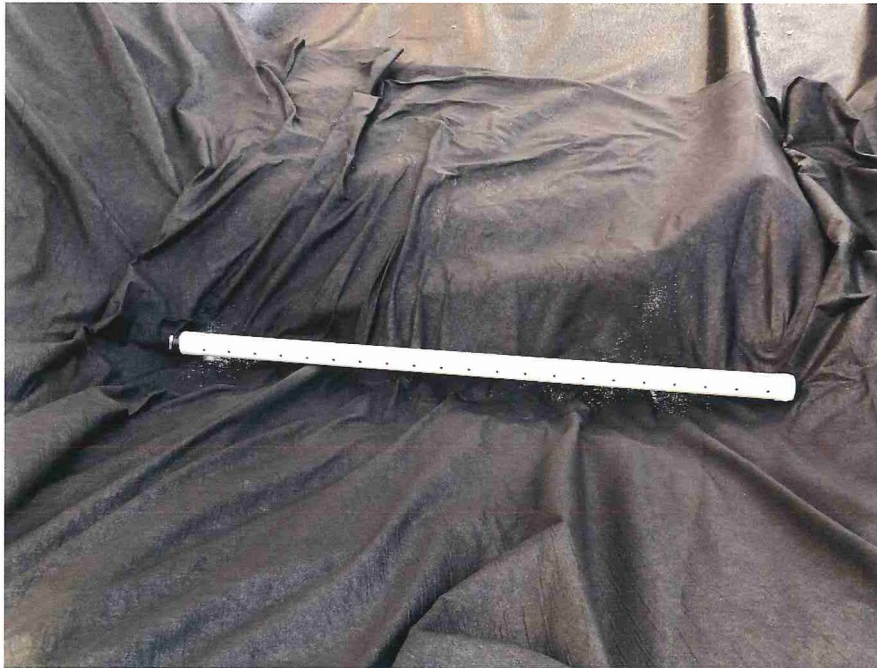
Photograph 22. Perforated drain pipe connected to stub from stormwater manhole, looking South.
