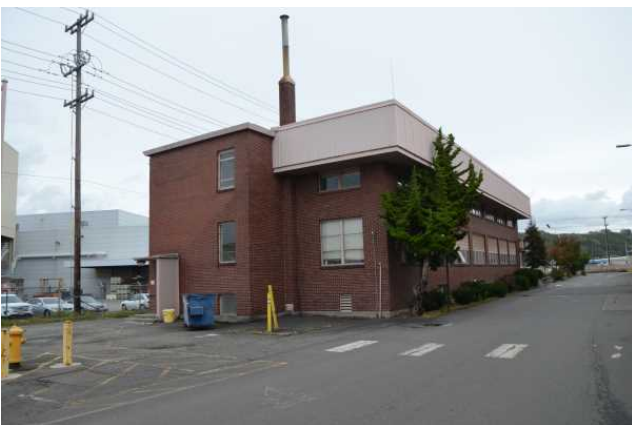
Southwest corner of building, view to the northeast.
