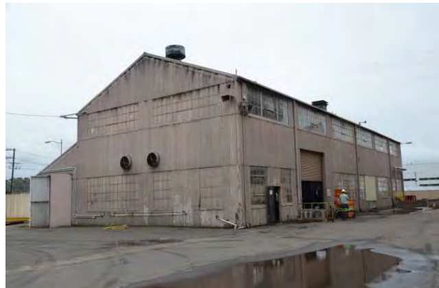
Northwest corner of building, view to the southeast.
