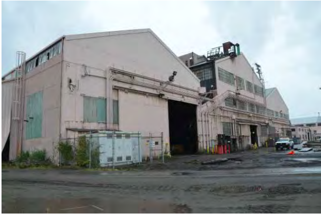
East end of Billet Yard, Forge Shop and Heat Treat (left to right), view to the northwest.
