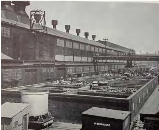
South side of Plant Two following construction of Melt Shop in 1943 (scrap metal storage in foreground) (Isaacson Iron Works 1943)
