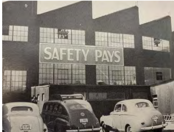
East side of the Machine Shop (Isaacson Iron Works 1943)
