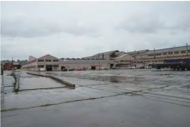
North end of Plant Number Two: (left to right) Erection Shop (Hollowbore), Machine Shop, Heat Treat, Melt Shop. View to the southeast.
