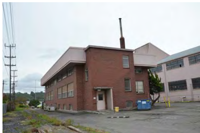
West end of building, view to the southeast.
