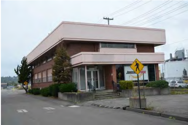
Office headquarters, view to the northwest.
