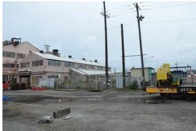
Power House with power lines and electrical equipment to right and Plant Number Two to left, view to the northwest.
