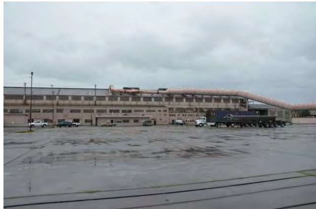
West half of Plant Number Two: Melt Shop and Melt Shop Warehouse (far right).
