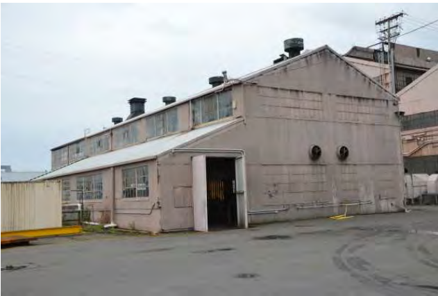
Northeast corner of building, view to the southwest.
