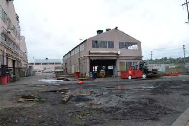
South end of building (Plant Number Two to left), view to the north.
