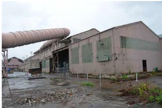
northwest corner of Melt Shop Warehouse, with Melt Shop in background, view to the southeast.
