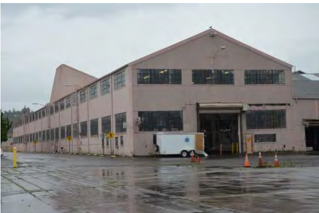
West end of Erection Shop (Hollowbore)
