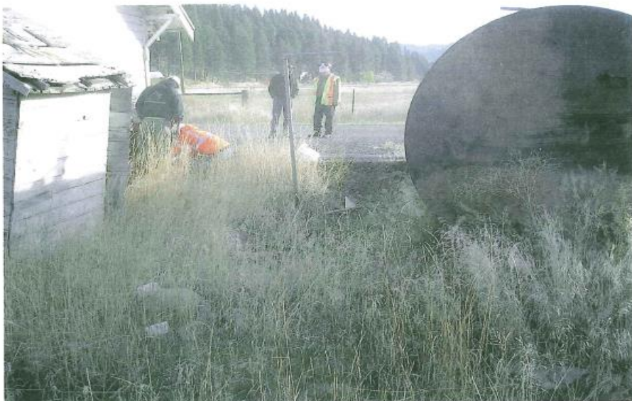
This picture shows the site when ACT first arrived & removed the dispenser. This picture was collected looking in a northeasterly direction.
