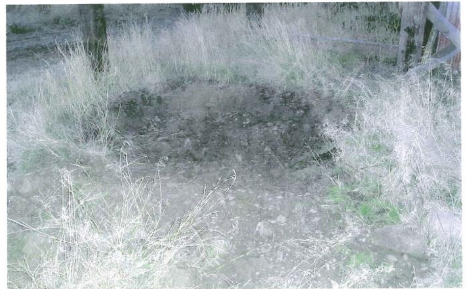
This picture shows the excavation at stained area #2. This picture was collected looking in a northeasterly direction.
