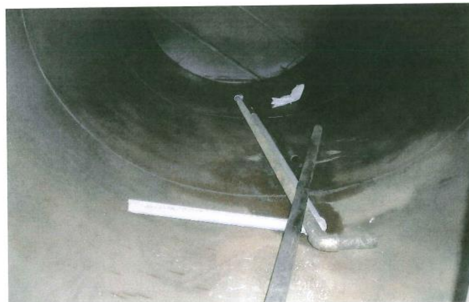
This picture shows the inside of the cleaned UST.
