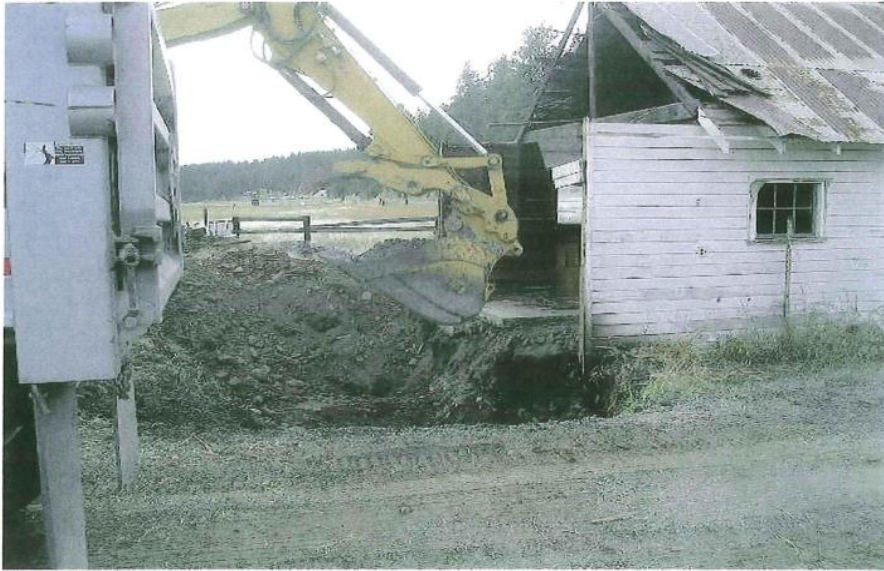
This picture shows the continued removal of the contaminated soils from around the dispenser. This picture was collected looking in a westerly direction.
