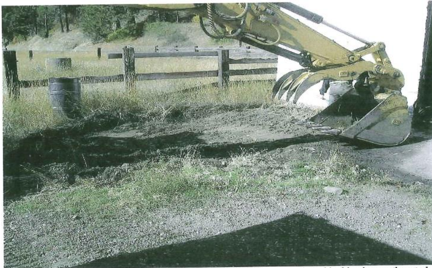
This picture shows the excavation at stained area #1. This picture was collected looking in a northwesterly direction.
