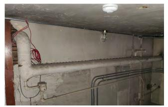
**Photo #11** View of a portion of potential asbestos containing materials (ACMs)
