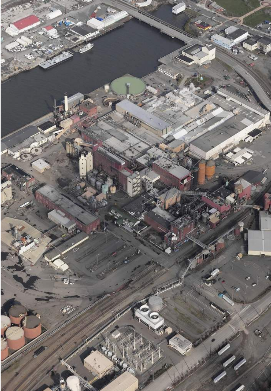
Figure 1.5: Old GP Mill Site
