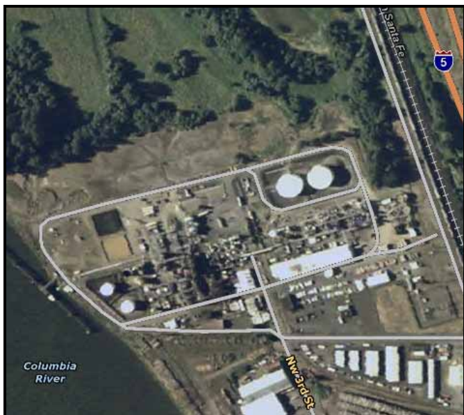
An aerial view of the Emerald Kalama plant
