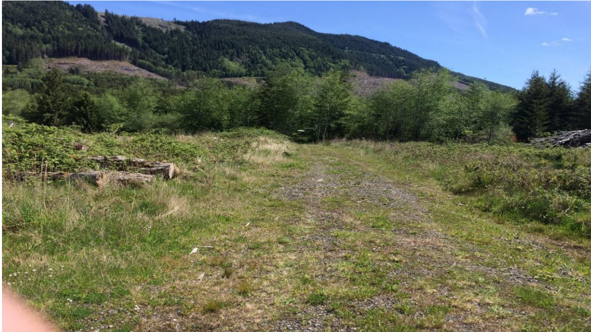
Photo 1. Dirt road to the Site and current general Site condition/overgrown wooded Area – from Southwest.
