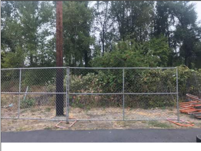
Picture Date: Friday 09/10/2021 Picture Taken By: Haley Provinsal Picture Location: Puyallup, Washington Project Name: USG Puyallup ISS Pilot Study Project Description: Temporary fence prior to be connected to original fence (middle of apple tree)
