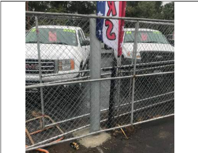
Picture Date: Friday 09/17/2021 Picture Taken By: Haley Provinsal Picture Location: Puyallup, Washington Project Name: USG Puyallup ISS Pilot Study Project Description: New post for new gate on eastern side of River Road entrance
