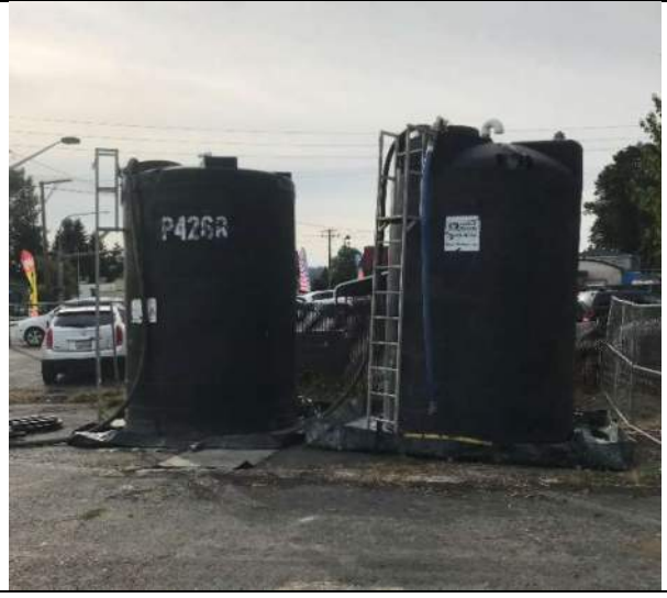
Picture Date: Thursday 09/16/2021 Picture Taken By: Haley Provinsal Picture Location: Puyallup, Washington Project Name: USG Puyallup ISS Pilot Study Project Description: Delivery of 2 water tanks and water
