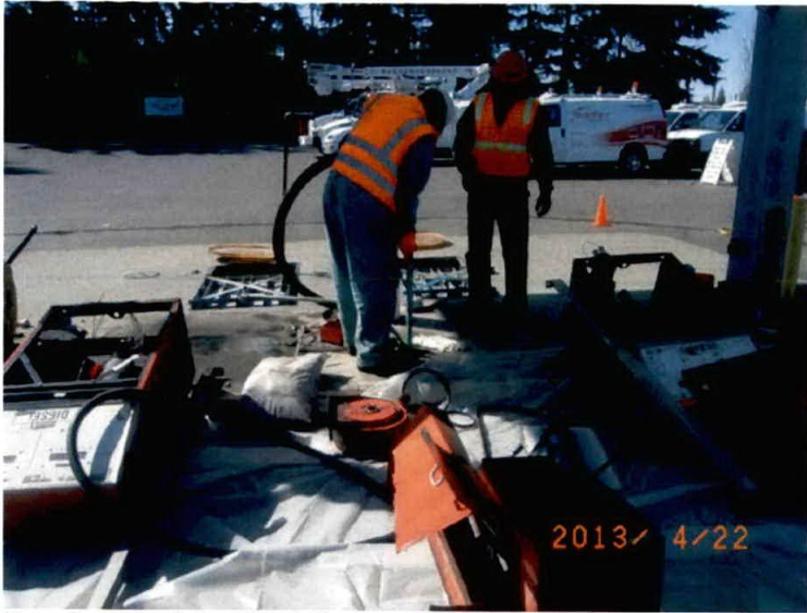
Pumping remaining fluids from tank
