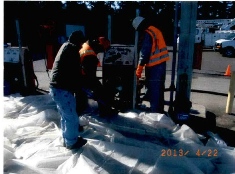
Draining product lines
