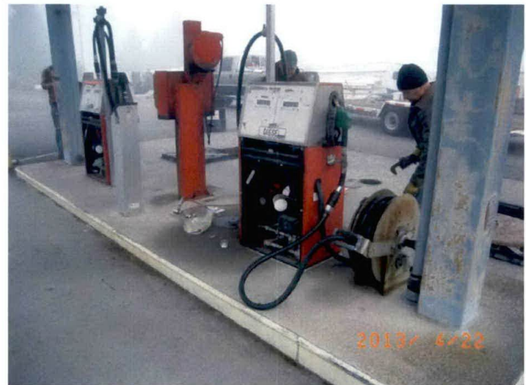
Beginning to dismantle dispensers
