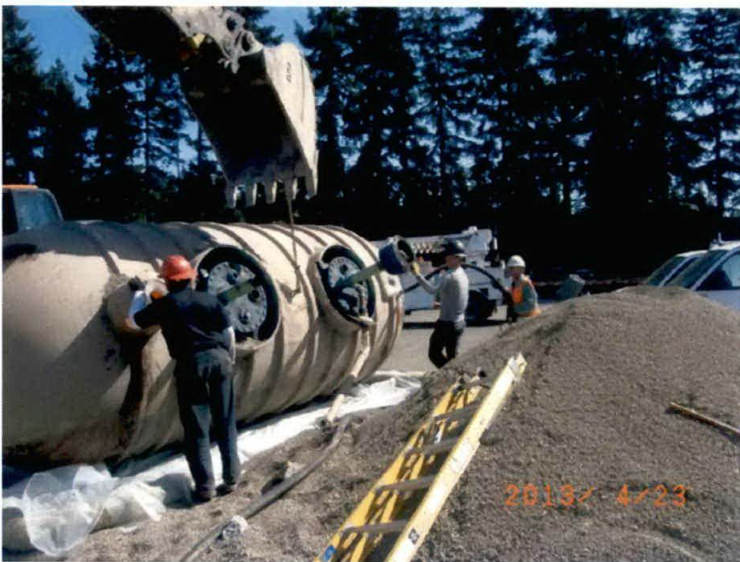
Removing interstitial fluids
