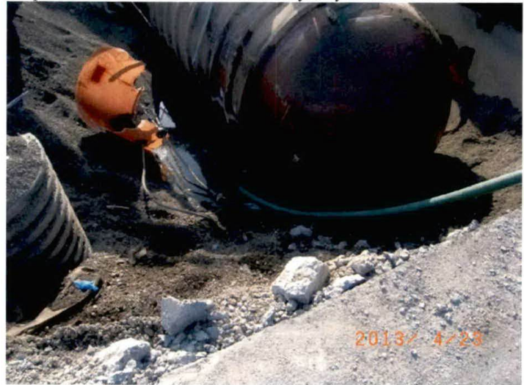
Pumping the excavation
