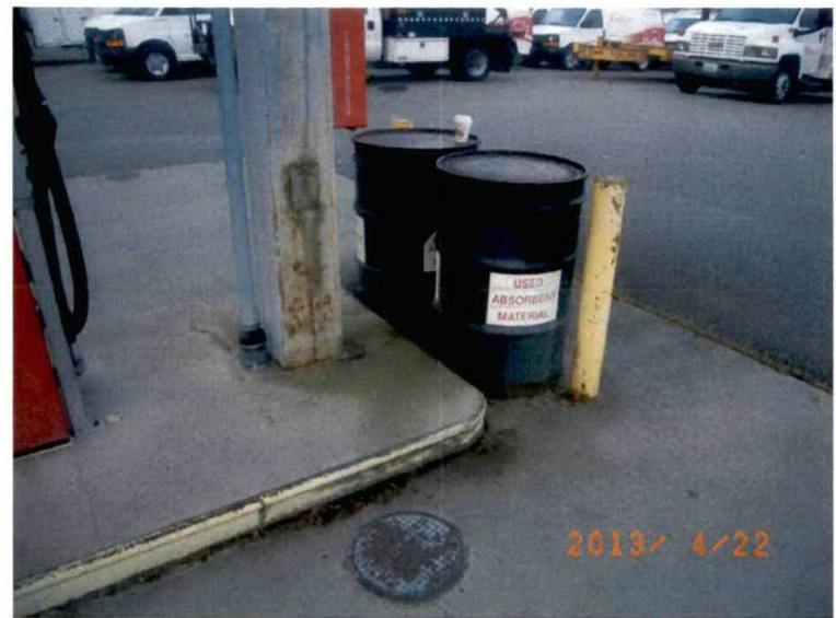
Vent pipe along canopy support
