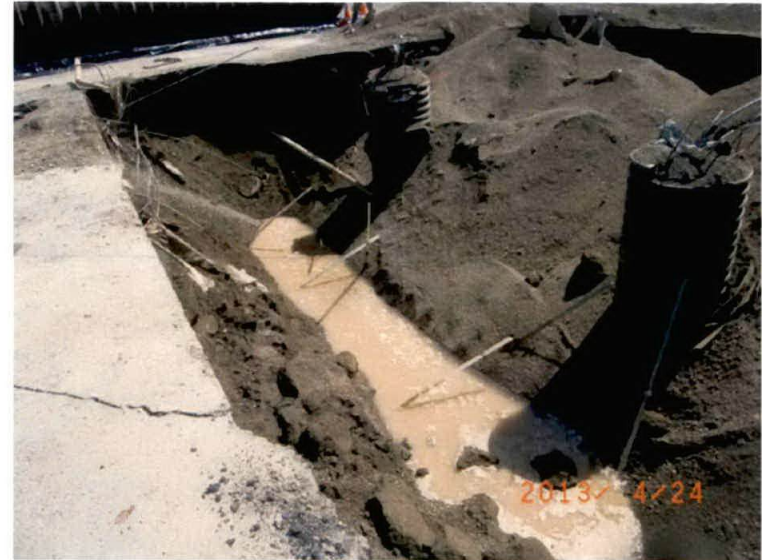
Reconnaissance ground water was sampled during decommissioning activities
