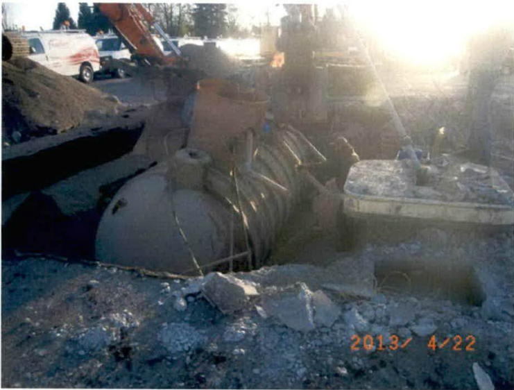
Tank being removed from excavation, assisted by buoyant forces
