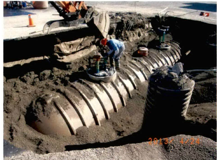
Preparing gasoline tank for removal
