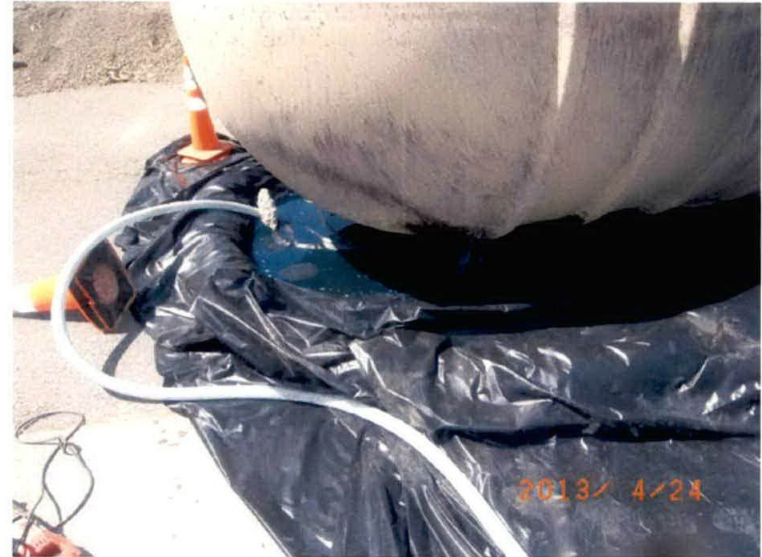
Removing interstitial fluids
