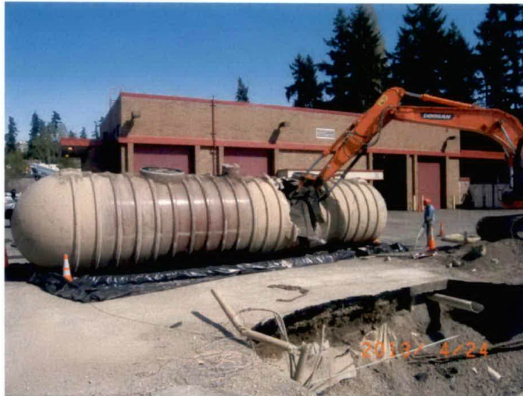
Ventilating the gasoline tank before removal from site to disposal facility
