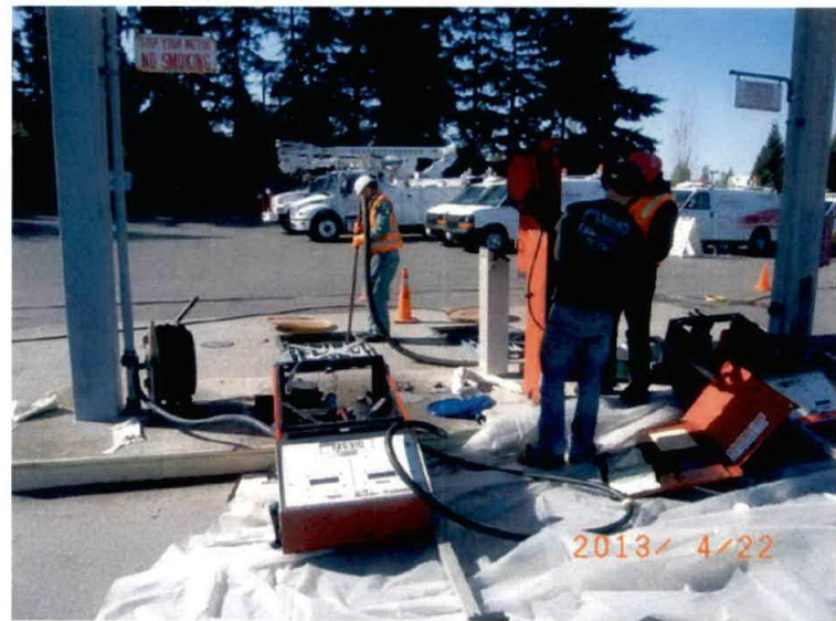
Dispensers removed from island
