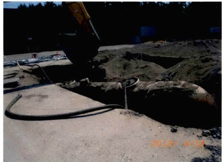
Preparing to lift gasoline tank
