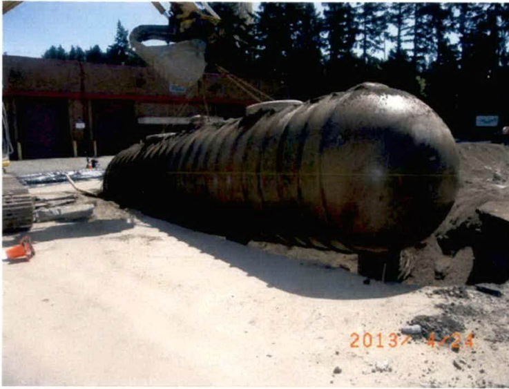
Lifting gasoline tank out of excavation
