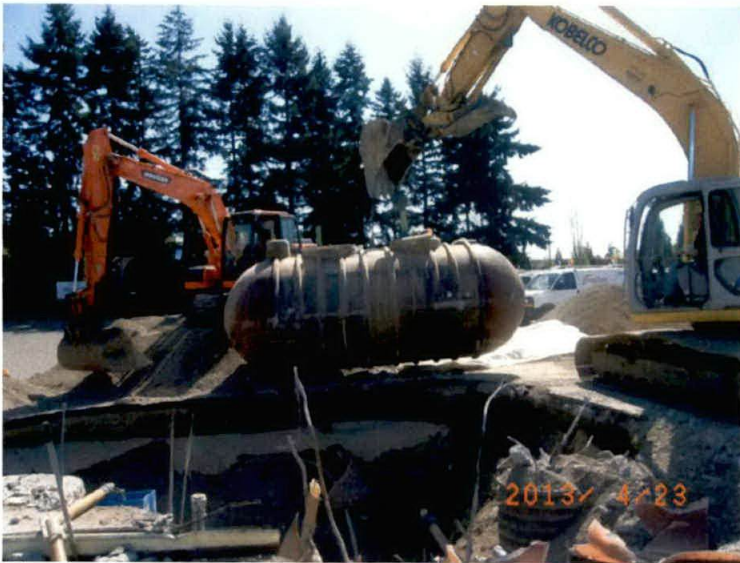
Diesel tank being removed from excavation
