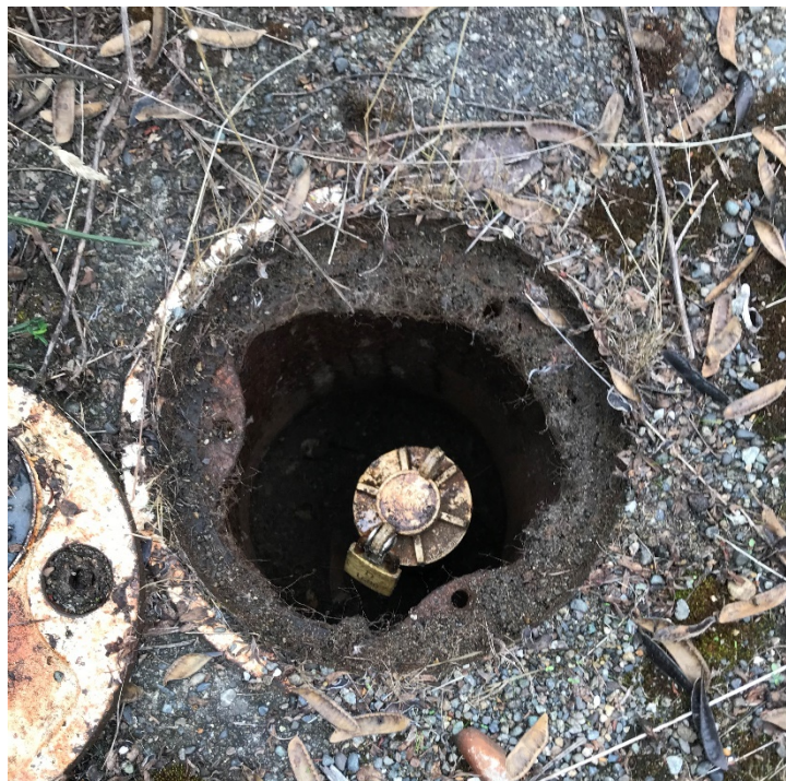
Photo 23: View of the monitoring well (MCW-2) with an inner cap.
