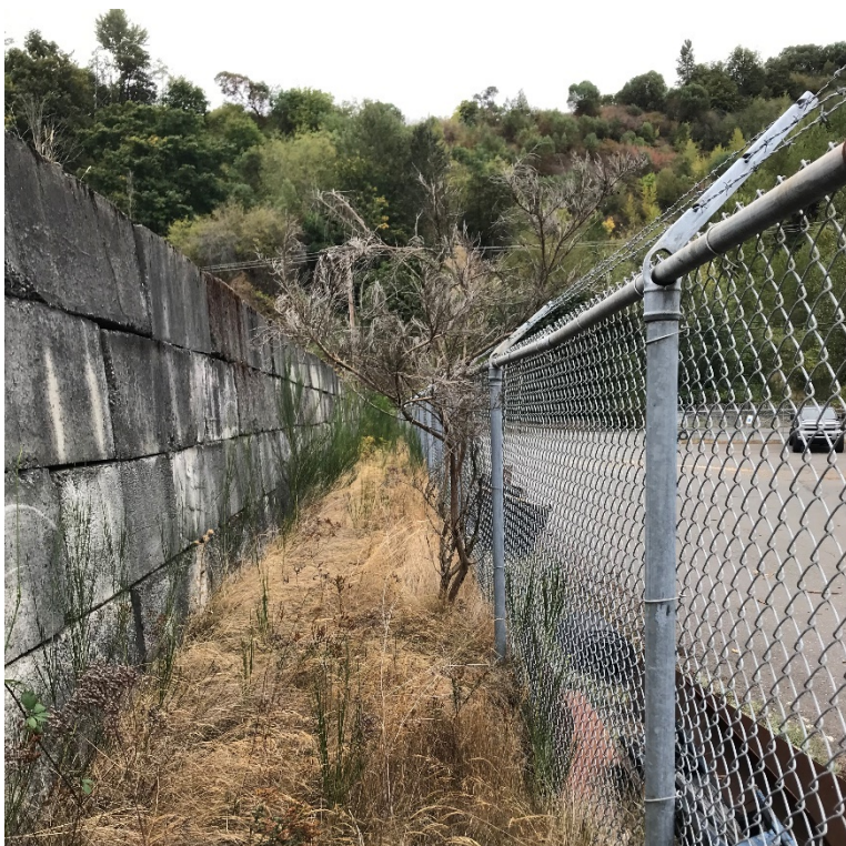
Photo 4: View of the walkway east of containment cell (facing north) with overgrowth of weeds and dead tree.
