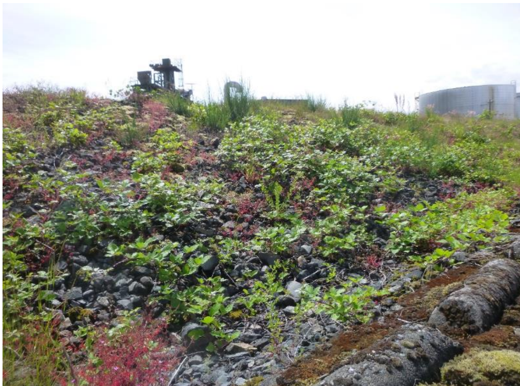
Photo 8: View of the center of containment cell cap with weed growth around a vent pipe (facing east).
