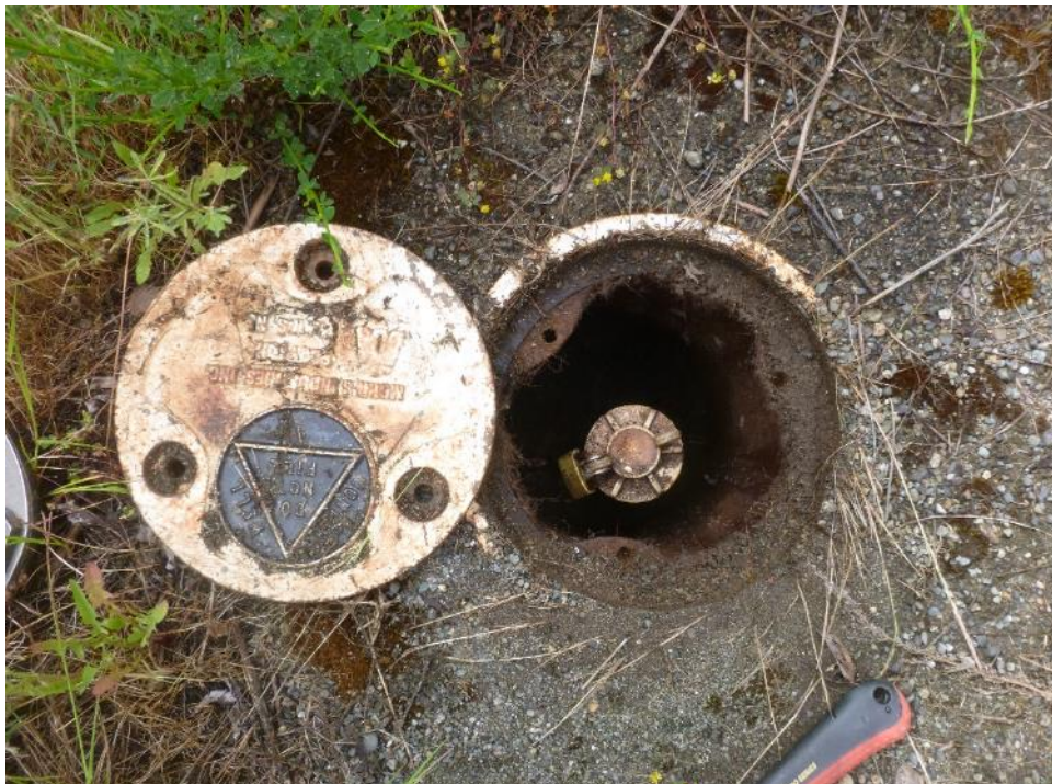
Photo 23: View of the monitoring well (MCW-2) with an inner cap.
