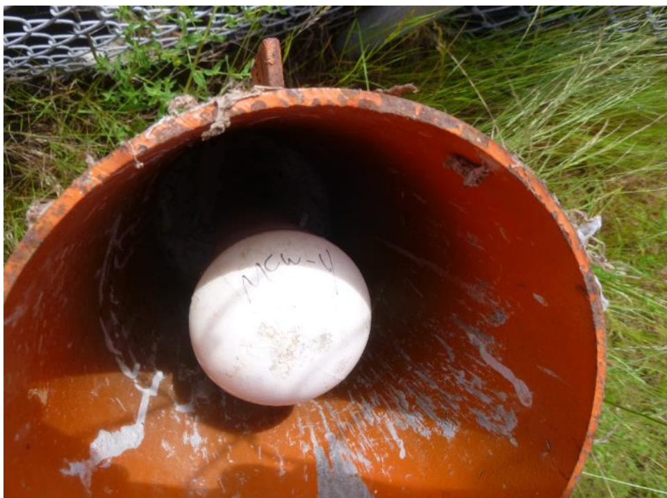
Photo 21: View of monitoring well (MCW-1) with an inner cap.
