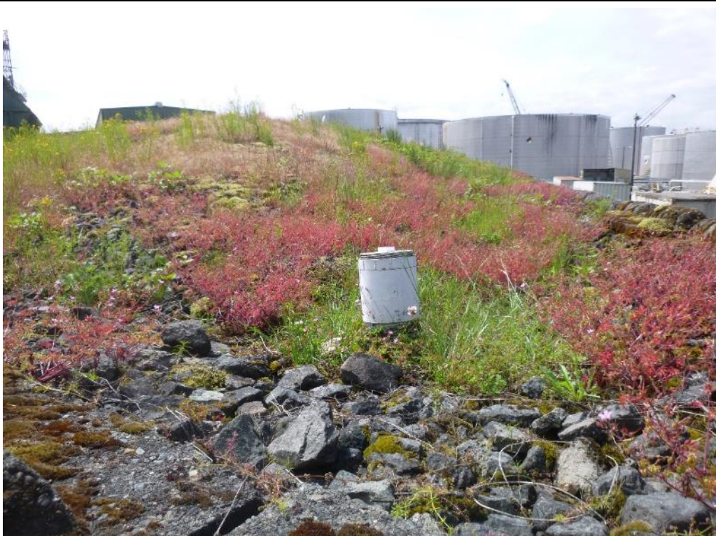
Photo 6: View of the northwest corner containment cell cap with a vent pipe (facing southeast)
