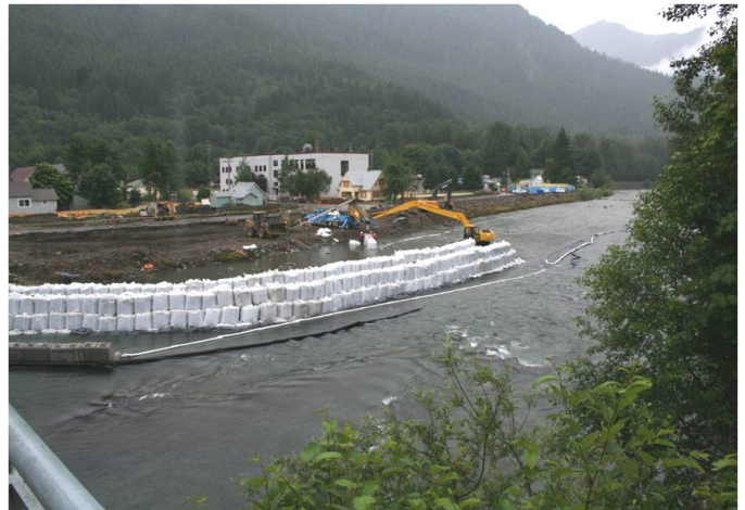
Skykomish River bank work, 2006
