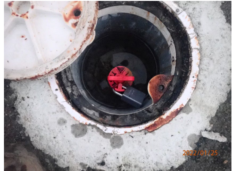
Well casings was fitted with a locking compression cap.
