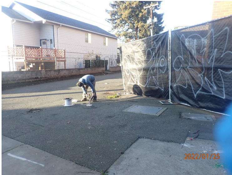
Gauging Well #2 with a depth to water meter.
