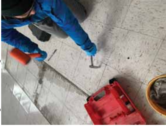
Installing a temporary Vapor Pin at SUB01.
