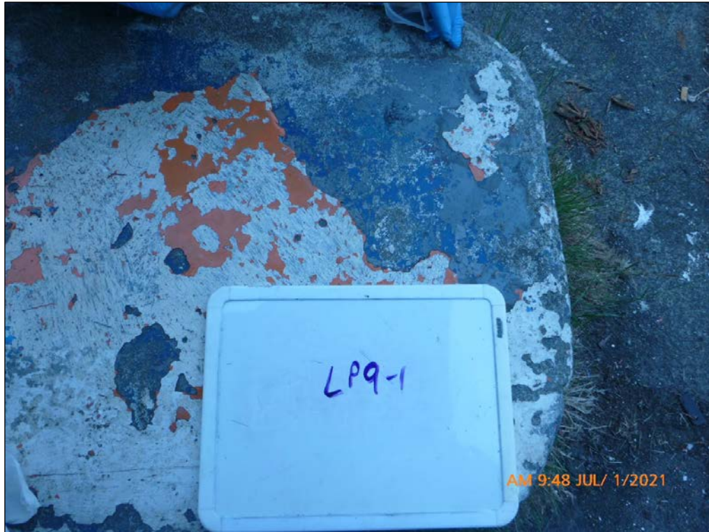
15. Lead paint sampling location LP9-1.
