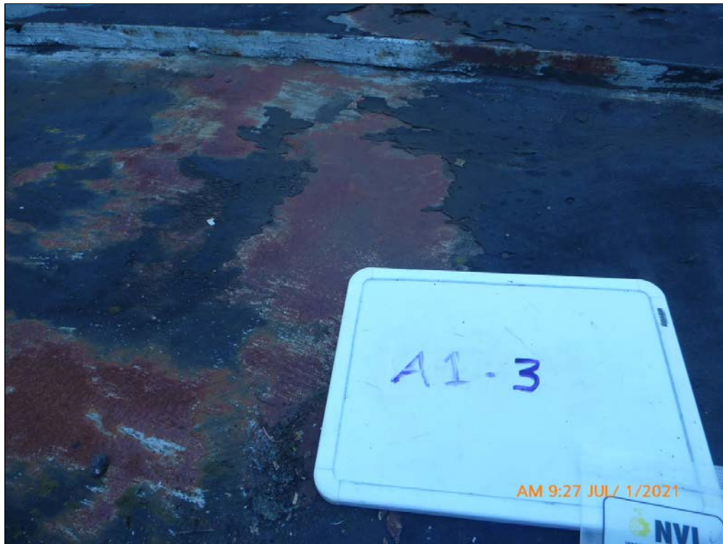
8. Asbestos sampling location A1-3.
