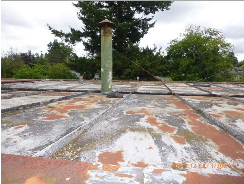
4. Building roof, looking east.
