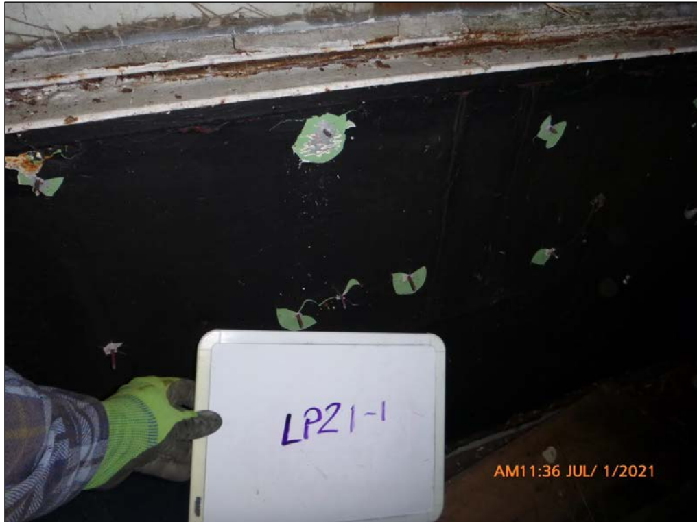
19. Lead paint sampling location LP21-1.
