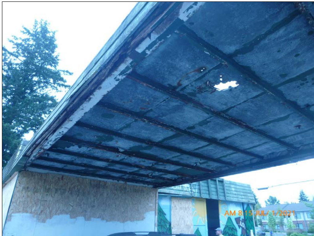
2. Building canopy, looking southeast.
