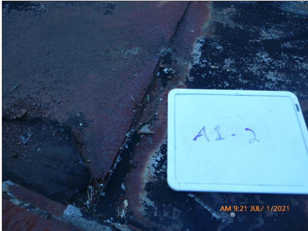
7. Asbestos sampling location A1-2.
