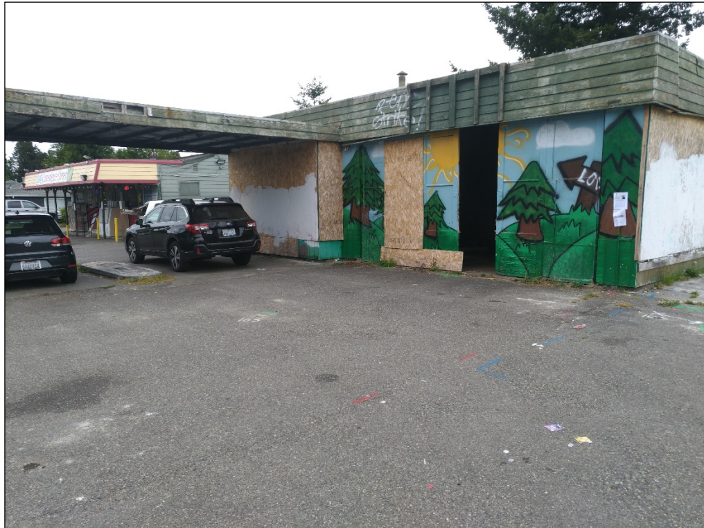
1. Building exterior, looking northeast.
