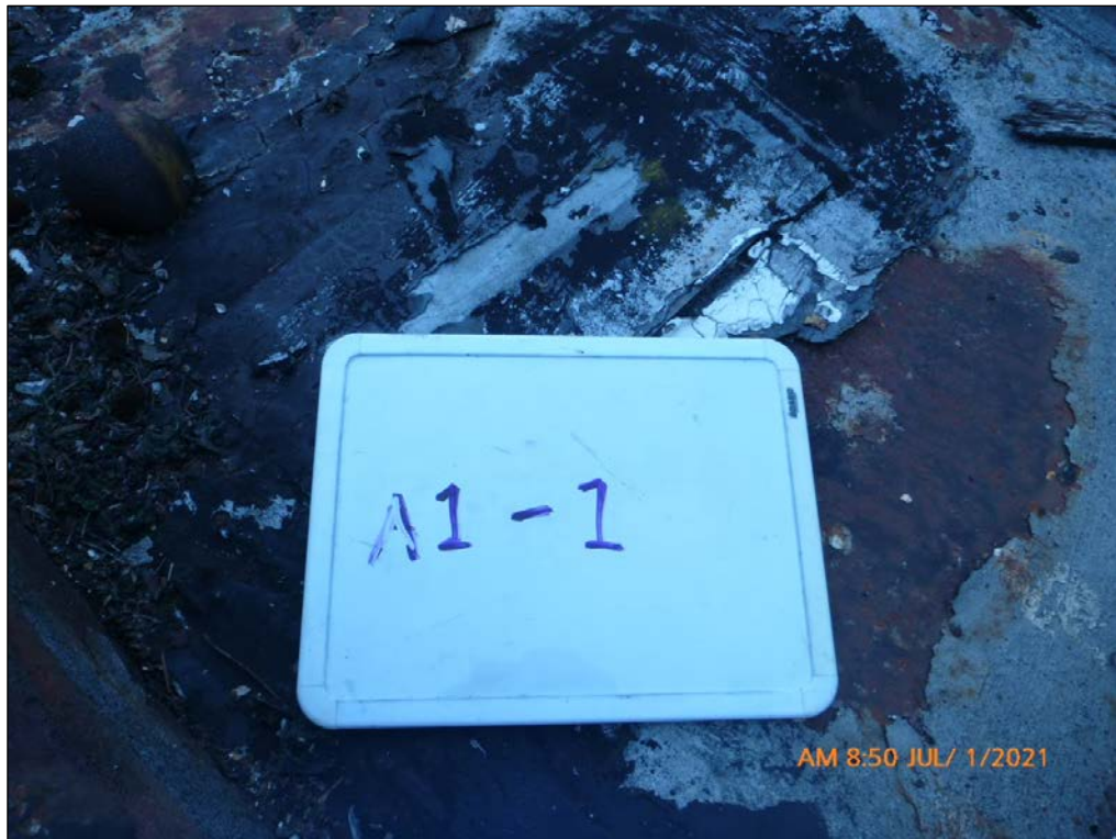
6. Asbestos sampling location A1-1.
