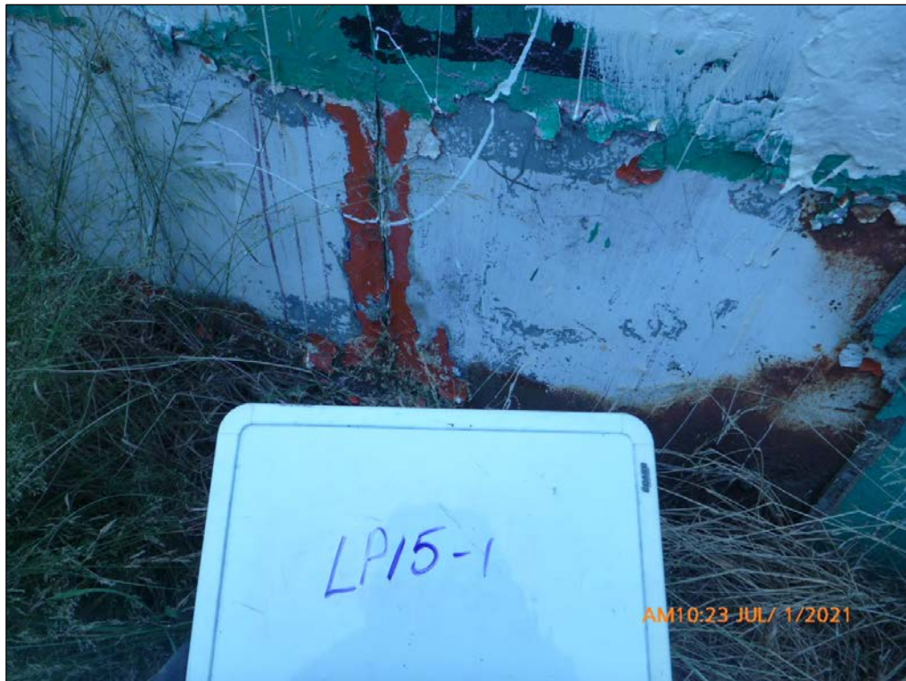
18. Lead paint sampling location LP15-1.
