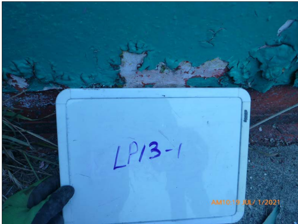
16. Lead paint sampling location LP13-1.
