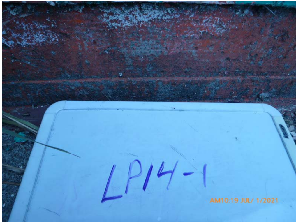
17. Lead paint sampling location LP14-1.
