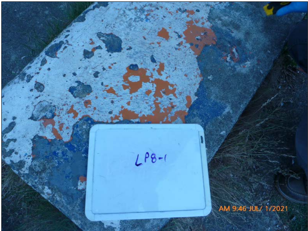
14. Lead paint sampling location LP8-1.
