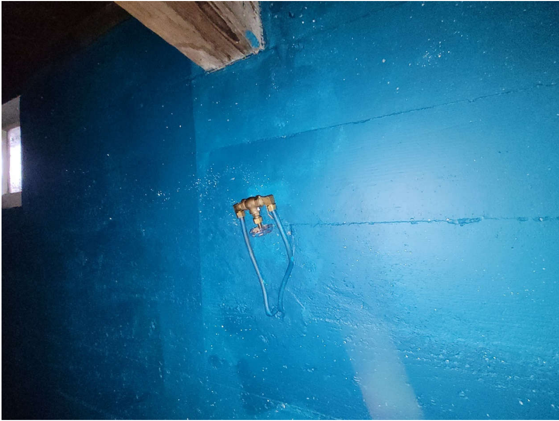
Photograph above of heating oil product lines in basement wall (residence at 7305 48 th St E) that appear to be capped off. Photograph below of electric furnace at same property.
