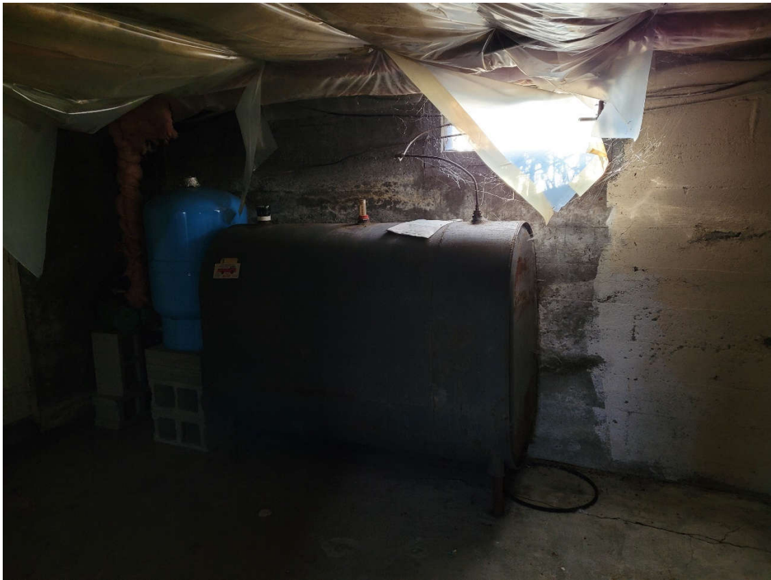
Photographs above and below of 275-gallon heating oil aboveground tank (AST) in basement of residence at 7111 48 th Street E.
