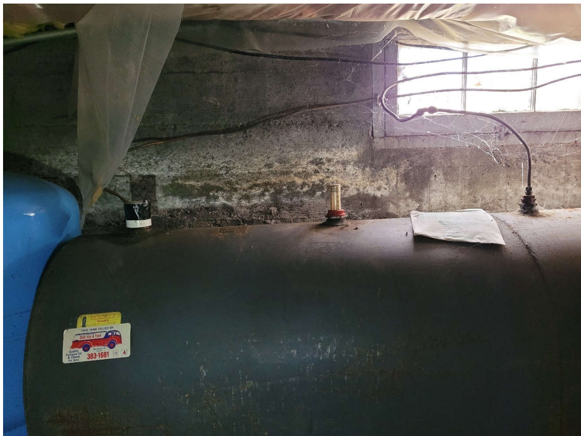
Photographs above and below of 275-gallon heating oil aboveground tank (AST) in basement of residence at 7111 48 th Street E.
