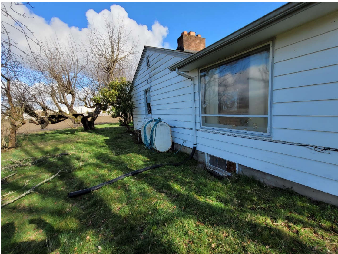
Photographs above and below of aboveground heating oil tank on west side of the residence at 7305 48 th Street E. Note in the photograph above, the vent pipe for a 675-gallon UST, to the left of the AST.
