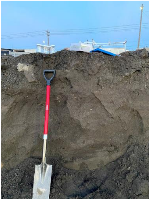
Photograph 17. 01/15/2021: SBG removed from sidewall. Limit of observed sand blast grit follows west side of original building footprint.
