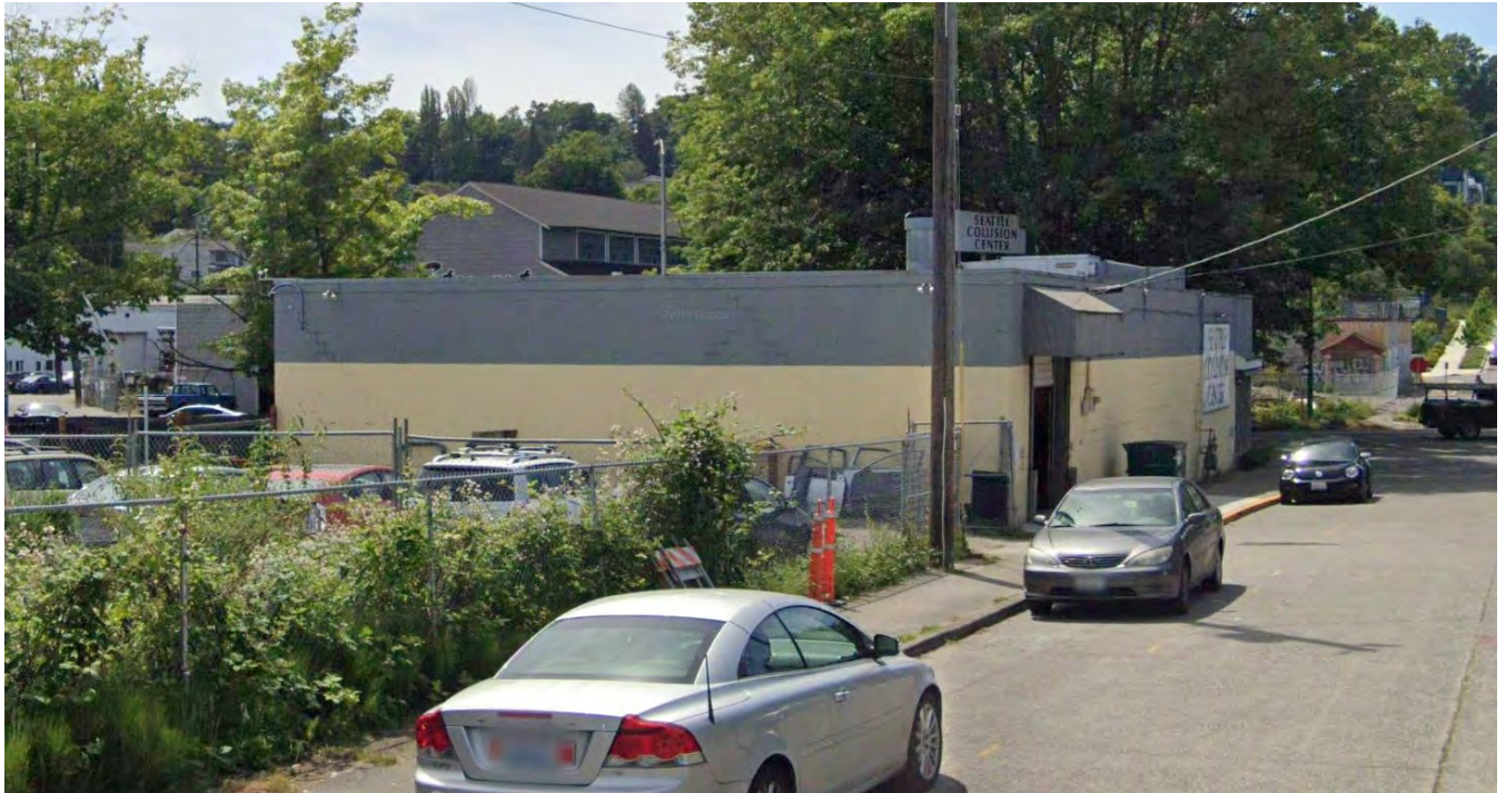
East façade of building, facing the parking lot.
