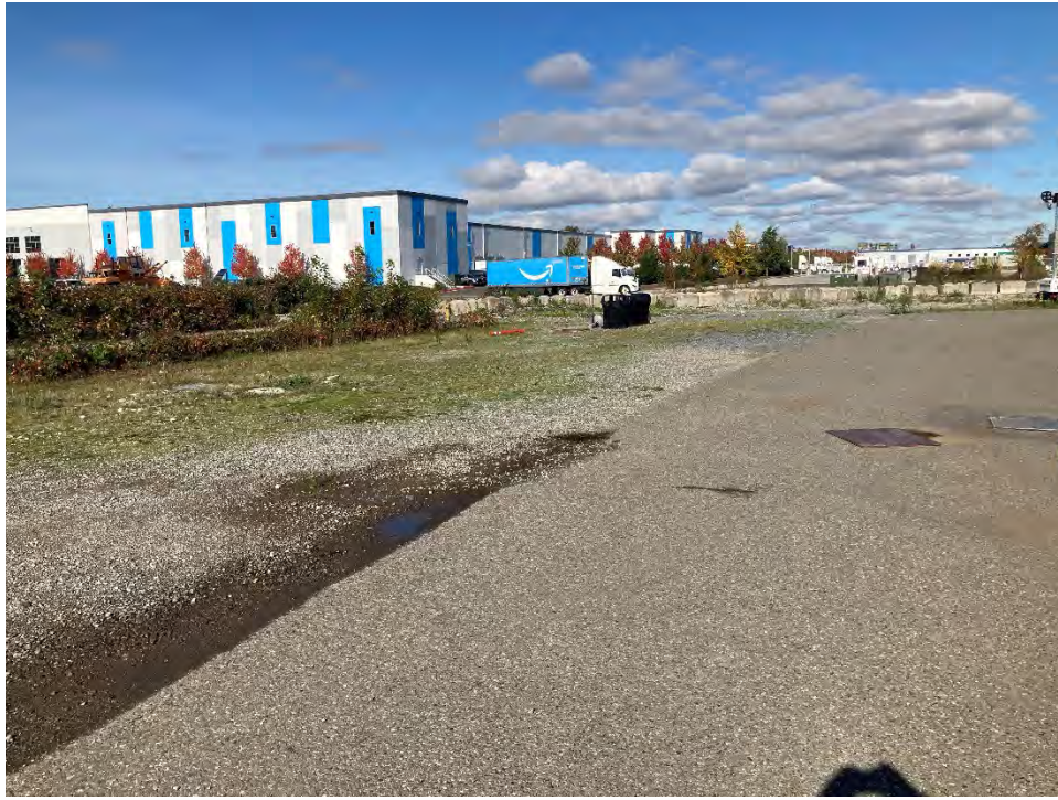
Photo 1. Looking north-northwest at the west portion of the asphalt cap.
