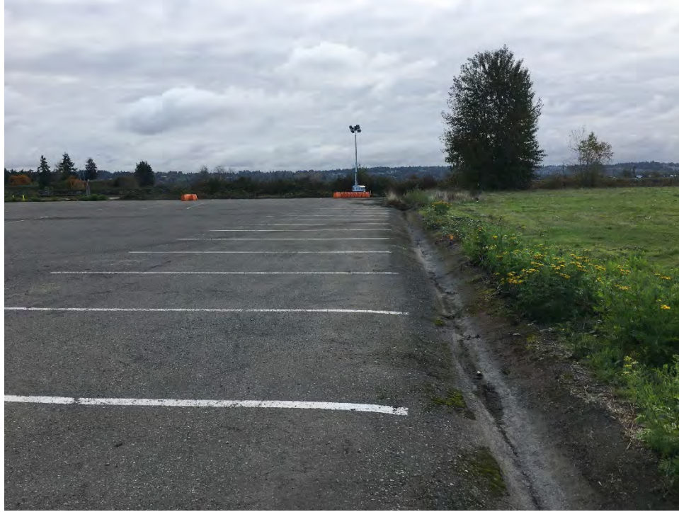
Photo 3. Looking east at the south drainage ditch. Less than 1 inch of accumulated sediment was observed.
