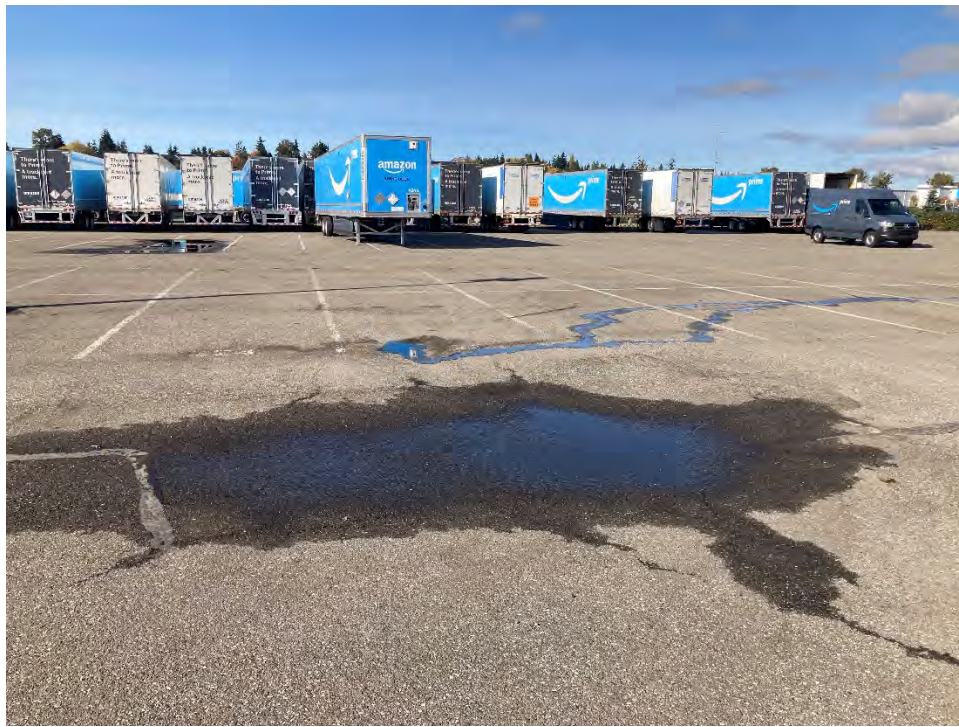
Photo 6. Observing the central portion of the asphalt cap.
