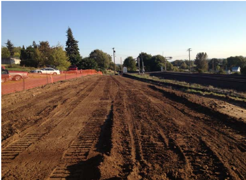
Photo 2: Reworking the subgrade at the Railroad Avenue Site.
