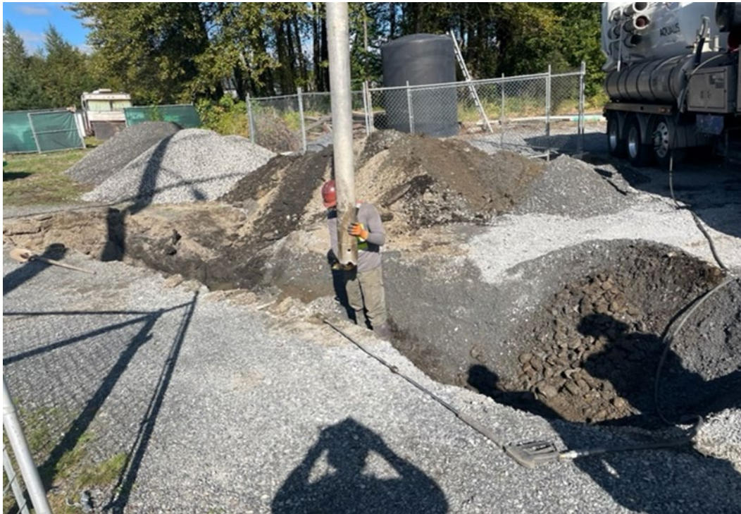
Photograph 10. Additional pothole investigation of active sewer line connections (facing north).
