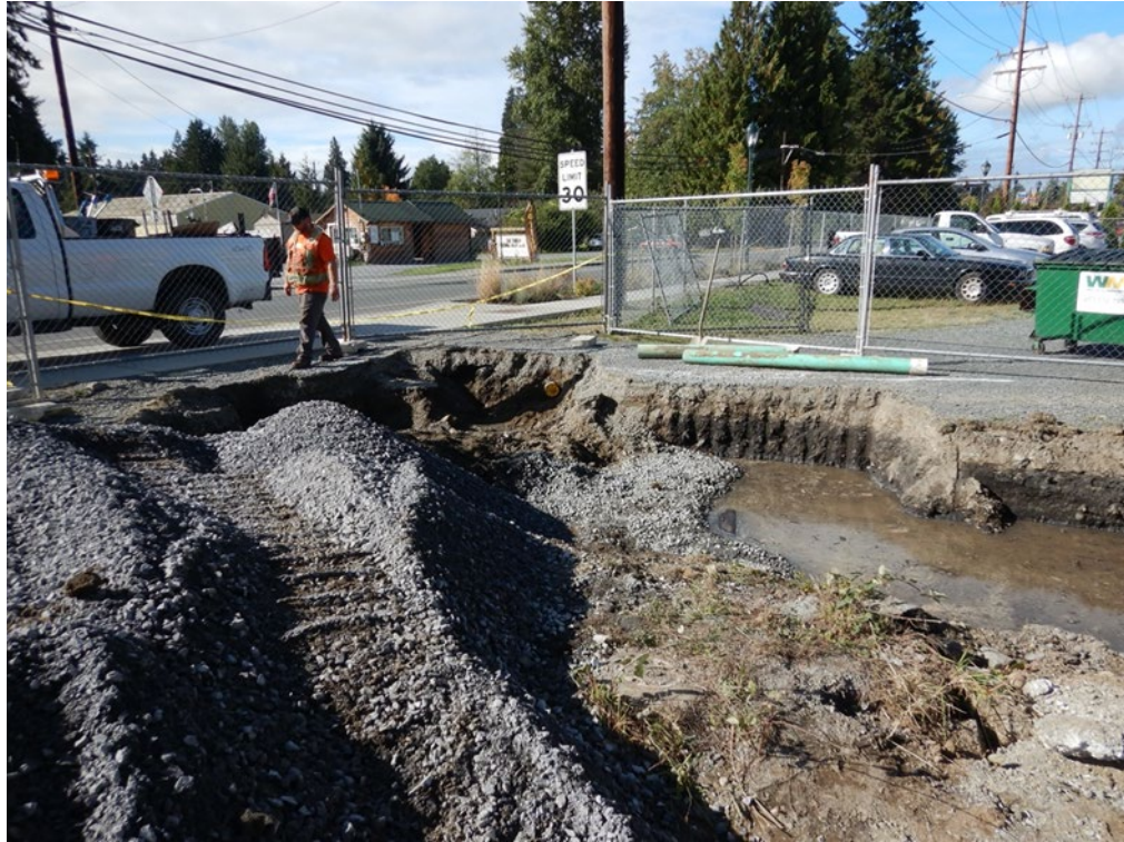
Photograph 7. Placement of backfill adjacent to City ROW (facing southwest).
