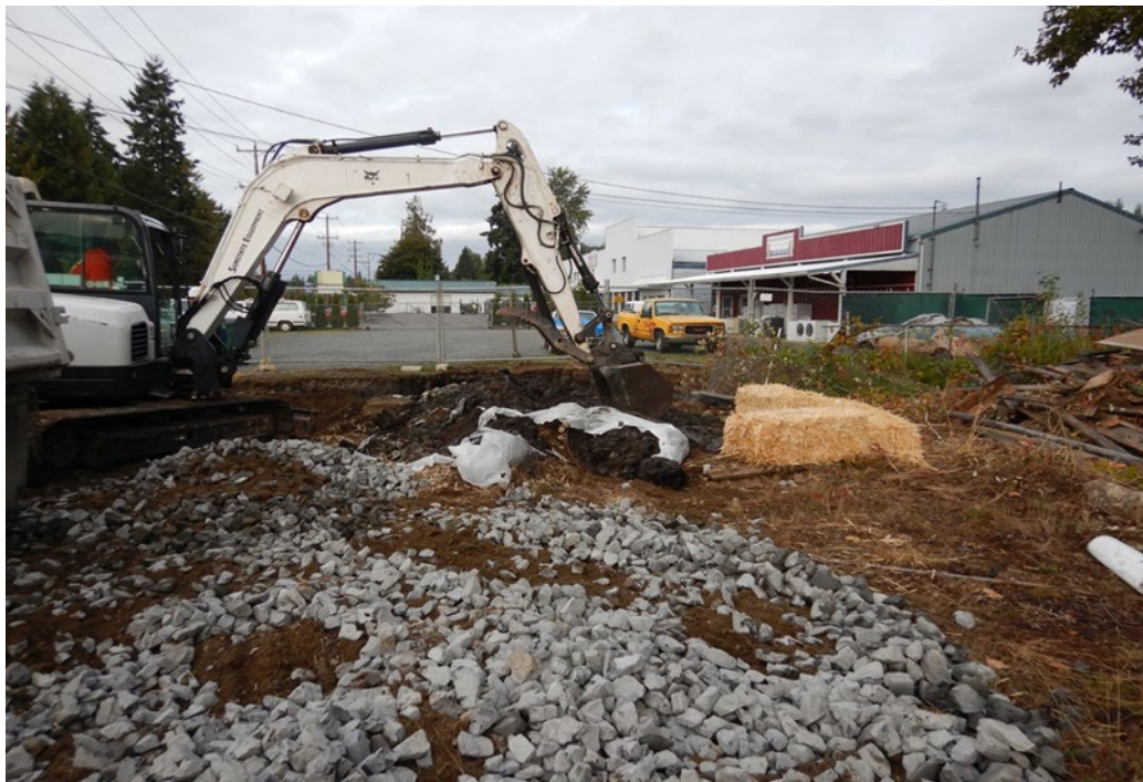
Photograph 6. Stabilized truck entrance and demolition of temporary stockpile (facing west).
