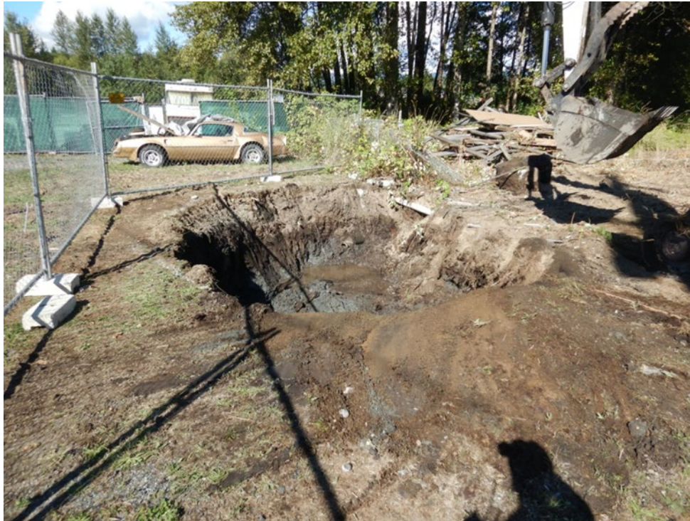
Photograph 3. Temporary fence and northwest corner of excavation area (facing north).
