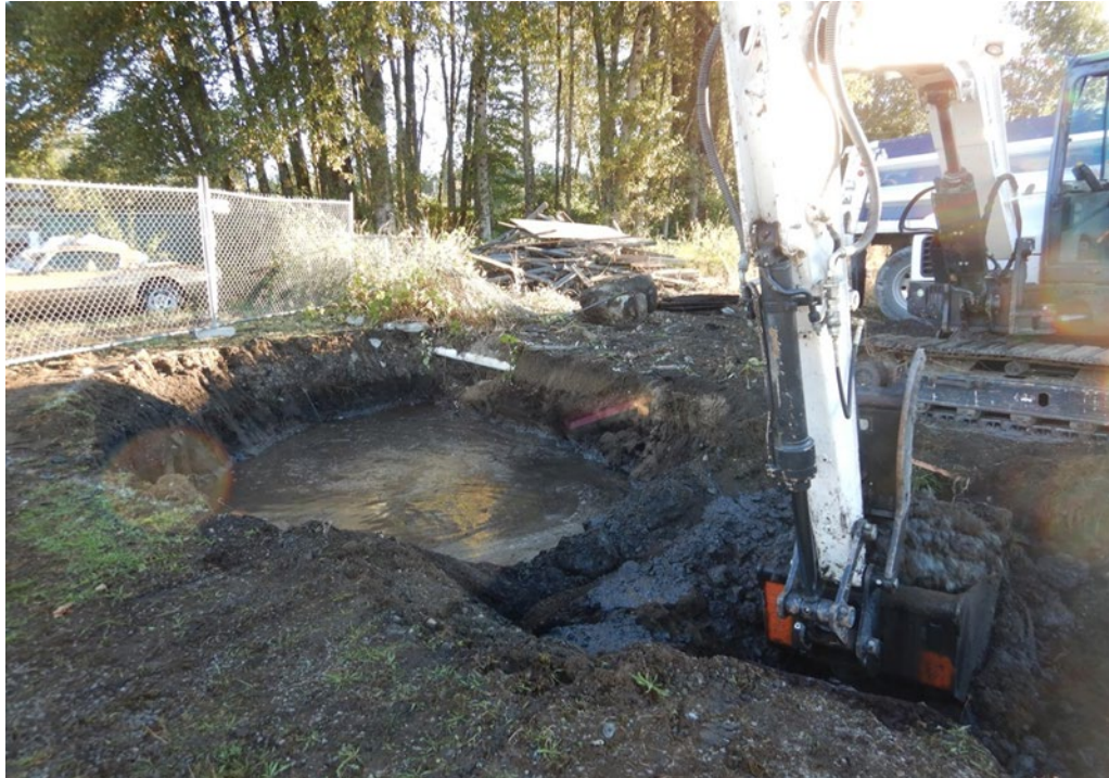
Photograph 5. Excavation with native soil buffer (facing east).
