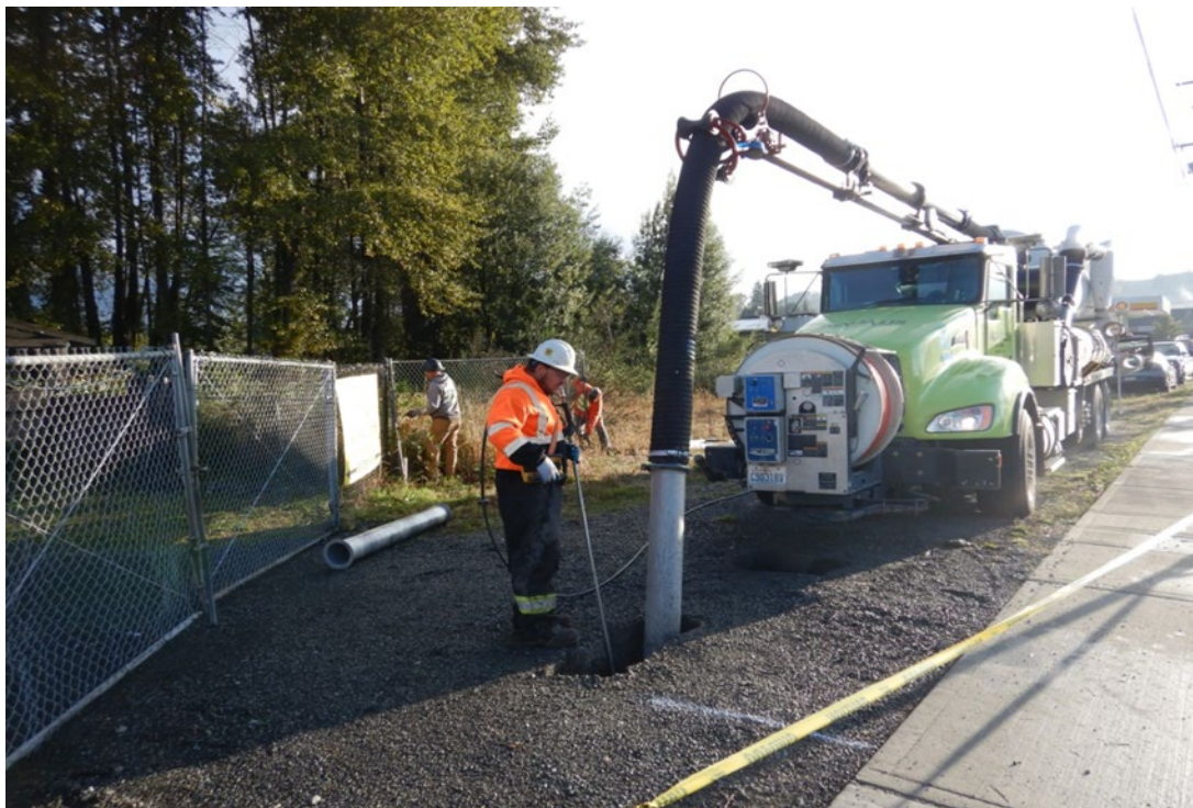
Photograph 1. Utility potholing for active water and sewer lines (facing northeast).
