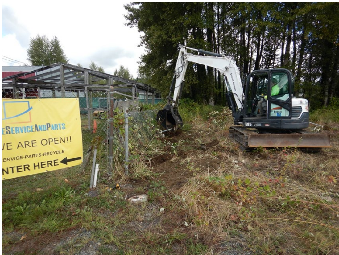
Photograph 2. Removal of property line fence (facing north).
