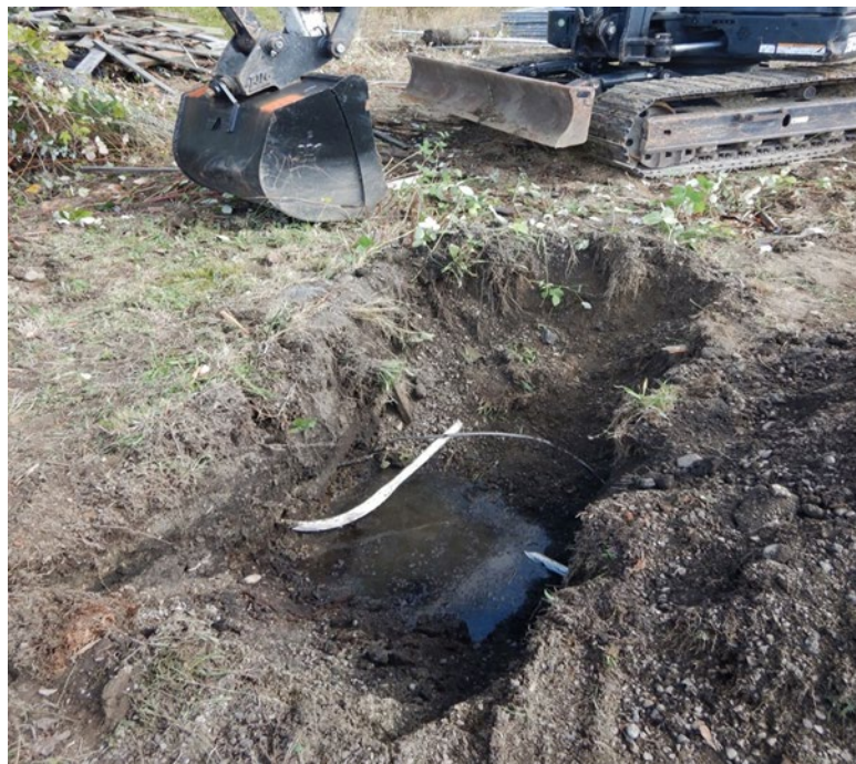
Photograph 4. Presumed 1.5-inch-diameter PVC water line and buried power (facing east).
