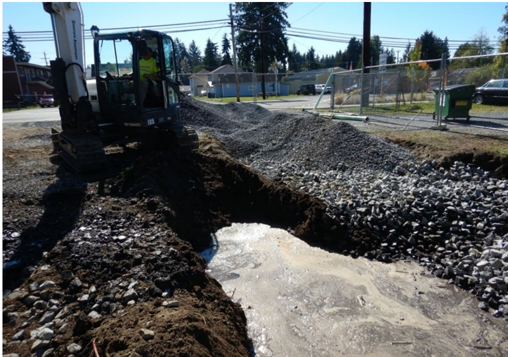
Photograph 8. Removal of native soil buffer during backfilling (facing south).
