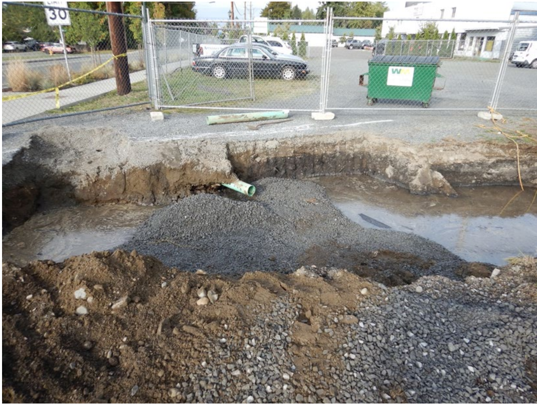
Photograph 9. Presumed 6-inch-diameter PVC drainage pipe (facing southwest).
