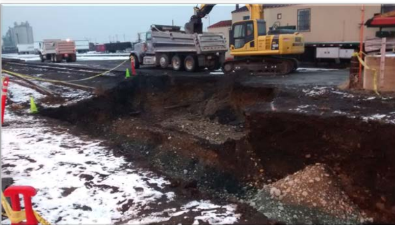
Photograph 4 – Soil excavation (west half excavation) - Looking to west.
