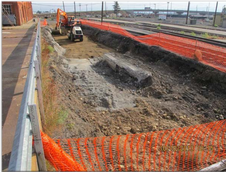
Photograph 3 – Soil excavation - Looking to northeast.
