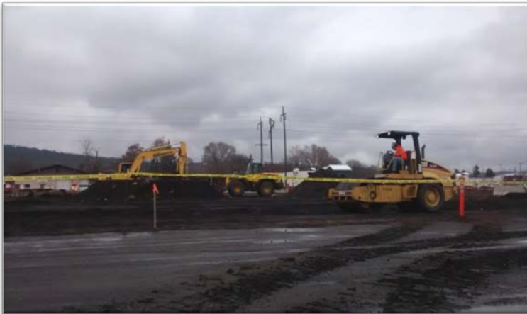
Photograph 7 – Initial grading activities - Looking to north.
