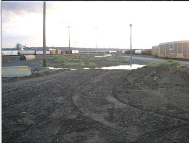
Photograph 2 –Preconstruction activities - Looking to west.
