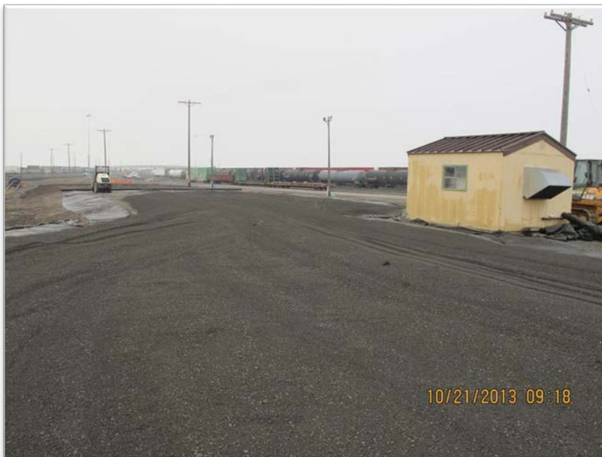
Photograph 6- Installing geo-textile fabric and cap material – Looking to west.
