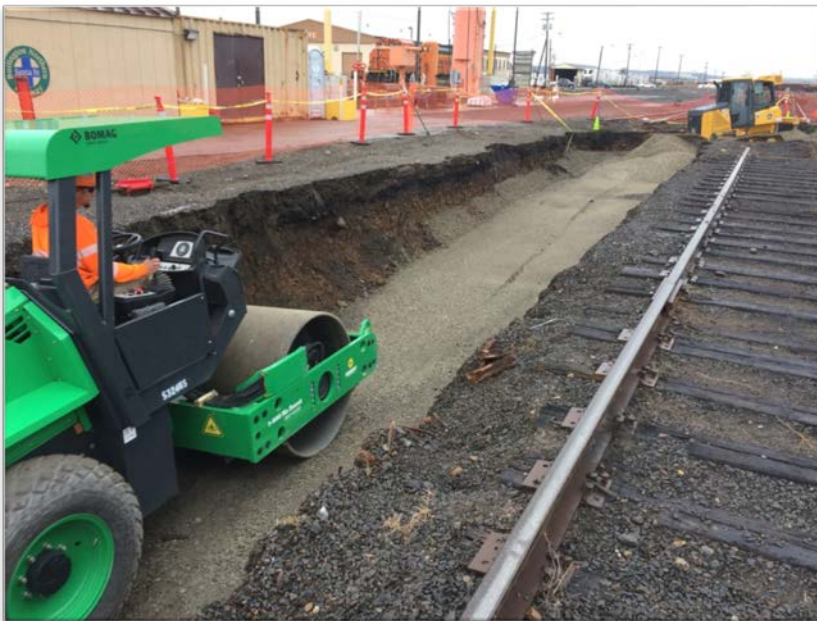
Photograph 5- Backfilling and compaction - Looking to southwest.
