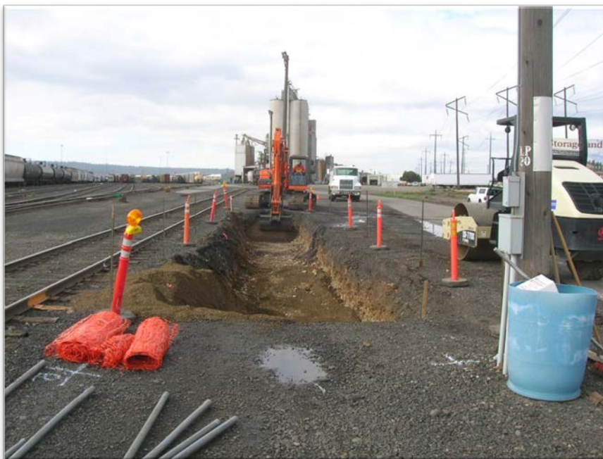
Photograph 8 – West excavation - Looking to west.
