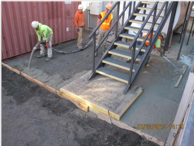
Photograph 5- Concrete placement (east end) - Looking to northeast.
