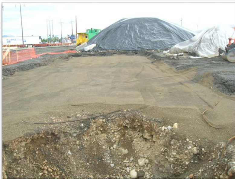
Photograph 4 – Backfilling soil excavation at GTP-48 & 50.
