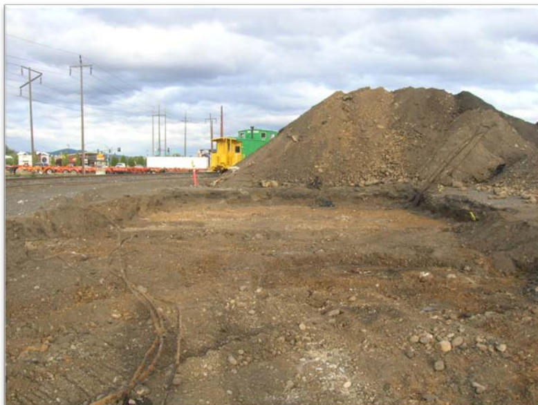
Photograph 3 – Soil excavation at GTP-48 & 50.
