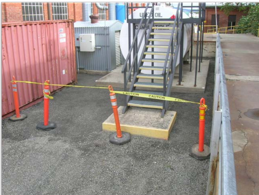
Photograph 2 – Preparing for concrete activities (east end) - Looking to northeast.
