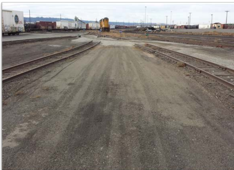
Photograph 6 –Backfill and capping- Looking to southwest.
