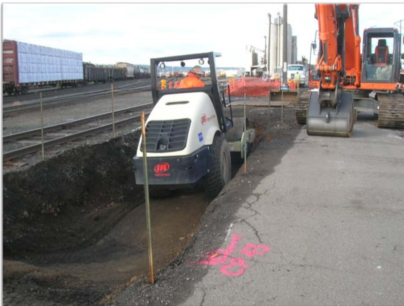
Photograph 6 – Backfilling and compaction of east excavation - Looking to west.
