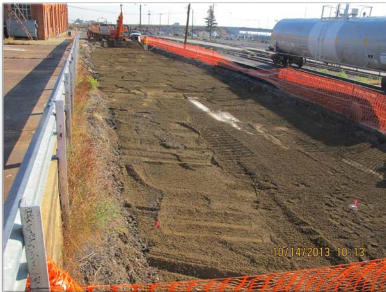
Photograph 4 – Backfill- Looking to northeast.
