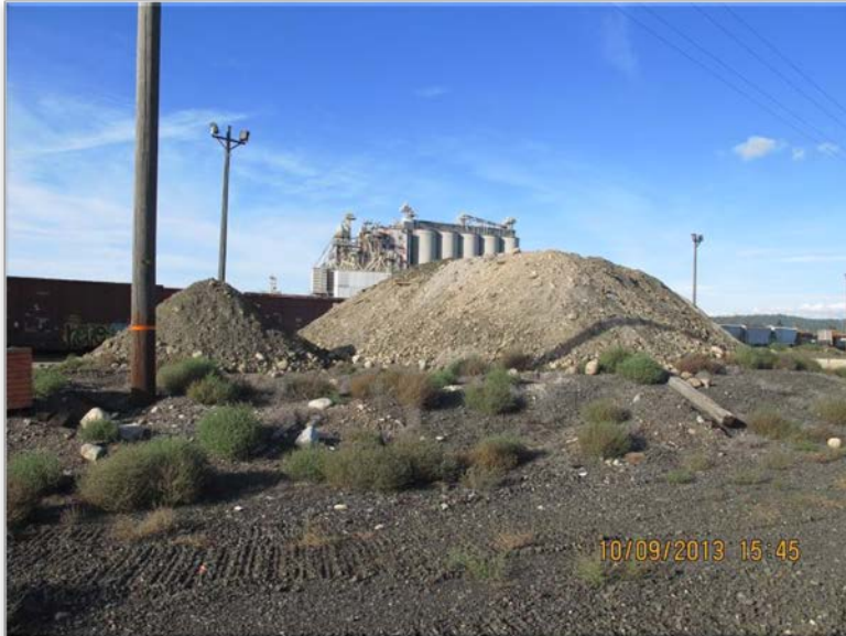
Photograph 3 – Materials storage building (east excavation) stockpile - Looking to north.
