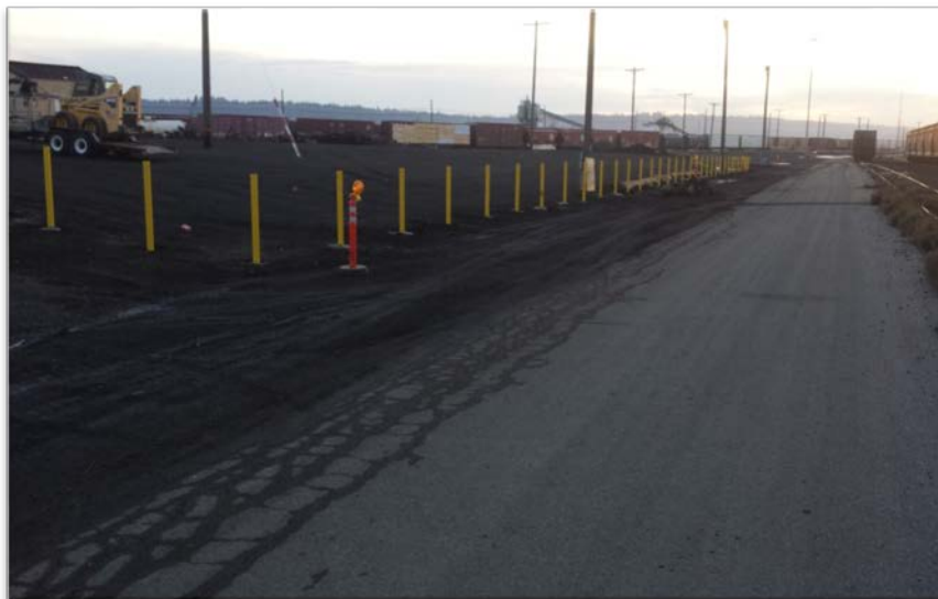
Photograph 10- Fencing – Looking to east.
