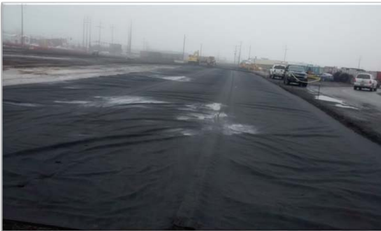
Photograph 8 – Geotextile placement activities – Looking to east.
