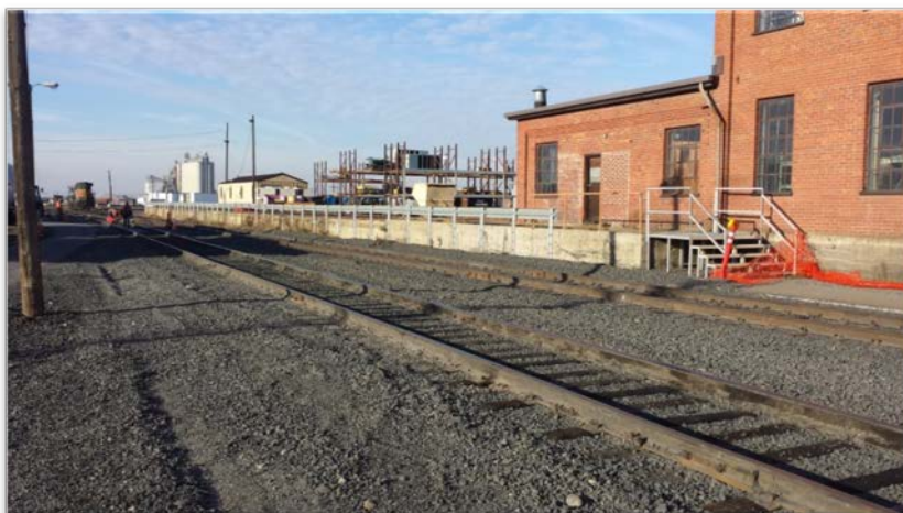
Photograph 5- Ballast and track replacement - Looking to west.
