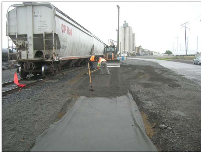
Photograph 10- Placement of geotextile and CSTC - Looking to west.
