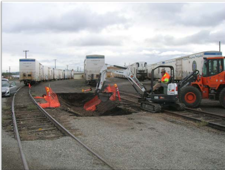
Photograph 4 – Over excavation - Looking to east.
