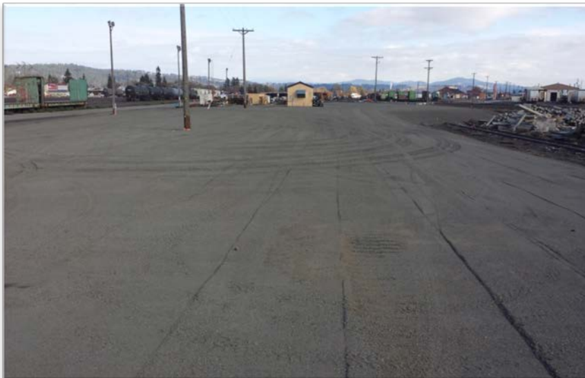
Photograph 8- Cap installed – Looking to east.
