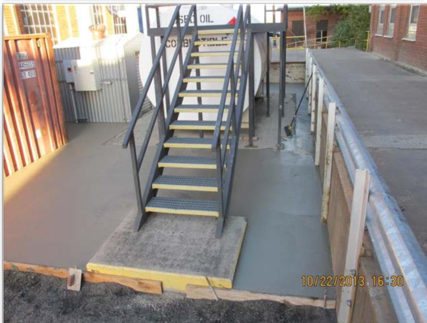
Photograph 6 – Concrete (east end) - Looking to northeast.
