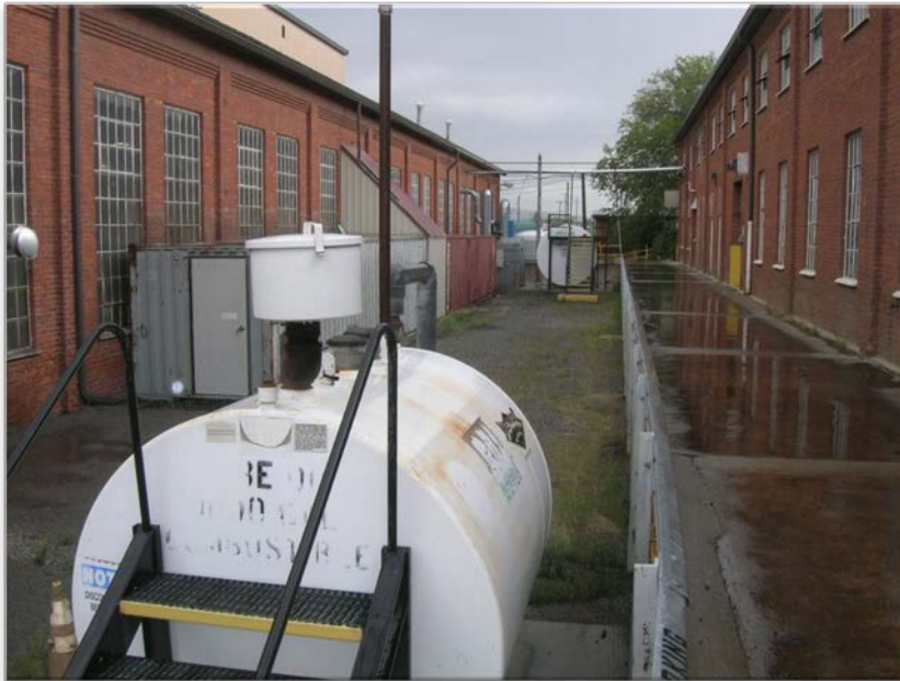
Photograph 1- Preconstruction activities - Looking to northeast.
