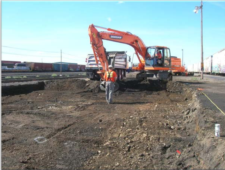
Photograph 1- Initial soil excavation - Looking to west.
