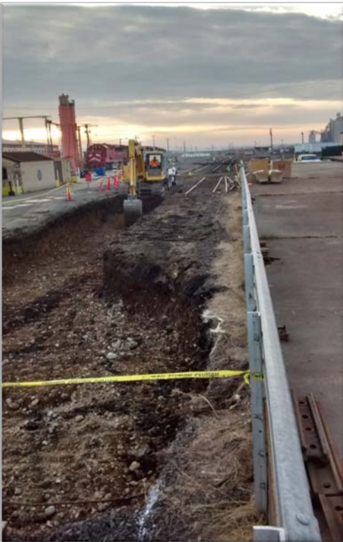
Photograph 3 – Soil excavation (west half excavation) - Looking to west.
