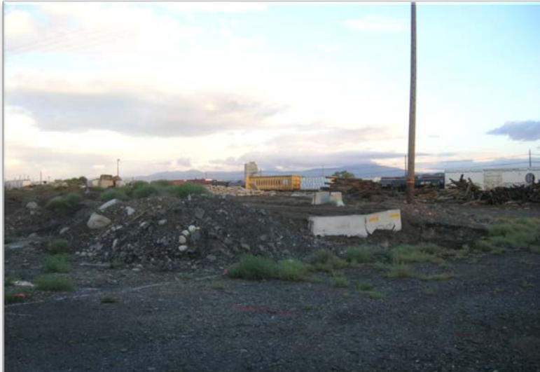
Photograph 1- Preconstruction activities - Looking to east.
