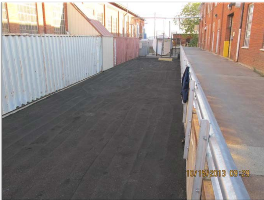
Photograph 4 – Grading and compacting structural backfill - Looking to northeast.
