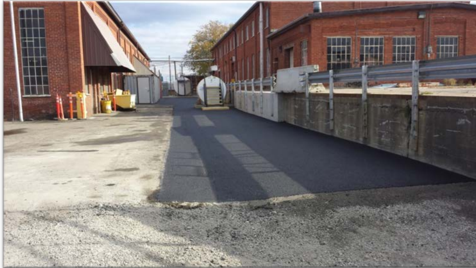
Photograph 8 – Asphalt - Looking to northeast.
