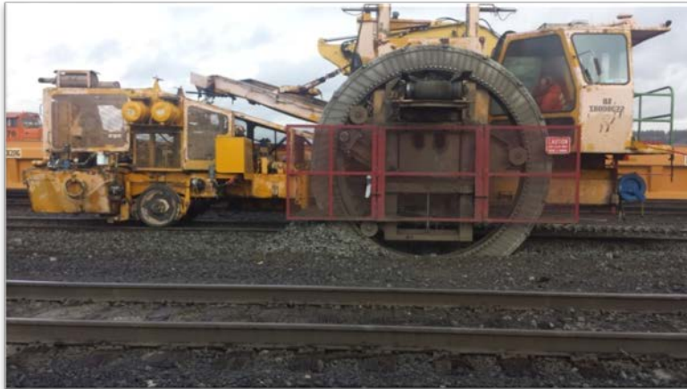
Photograph 1- Undercutter- Looking to north.
