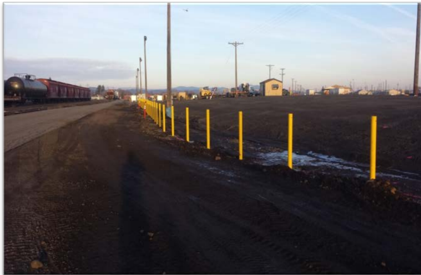
Photograph 9- Fencing – Looking to east.
