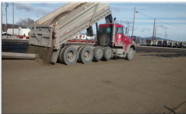
Photograph 9- Placement of CSTC cap - Looking to northeast.
