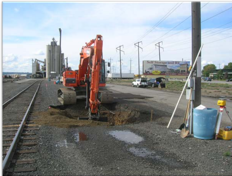
Photograph 2 – Soil excavation (east excavation) - Looking to west.
