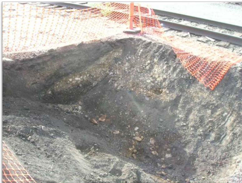
Photograph 2 – Initial soil excavation - Looking to west.
