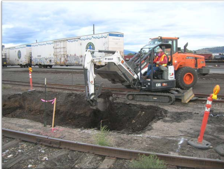
Photograph 3 – Over excavation- Looking to southeast.
