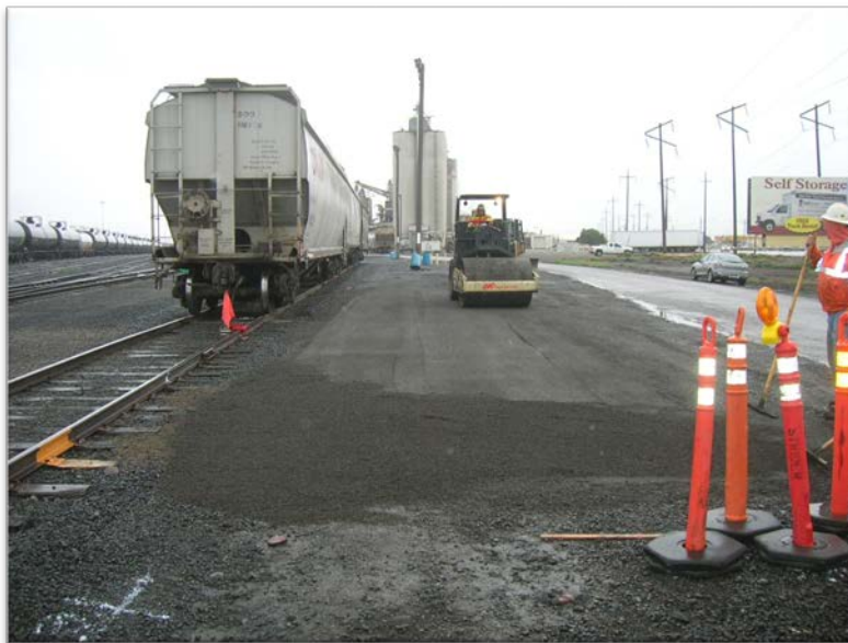
Photograph 12- Compacted CSTC (west excavation) - Looking to west.
