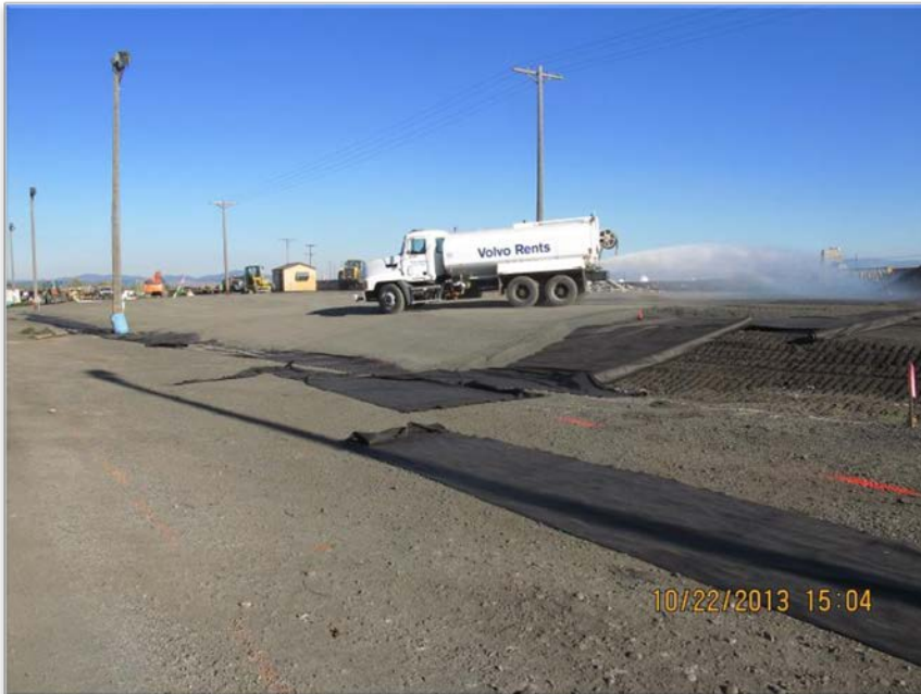
Photograph 7- Installing geo-textile fabric and cap material – Looking to west.
