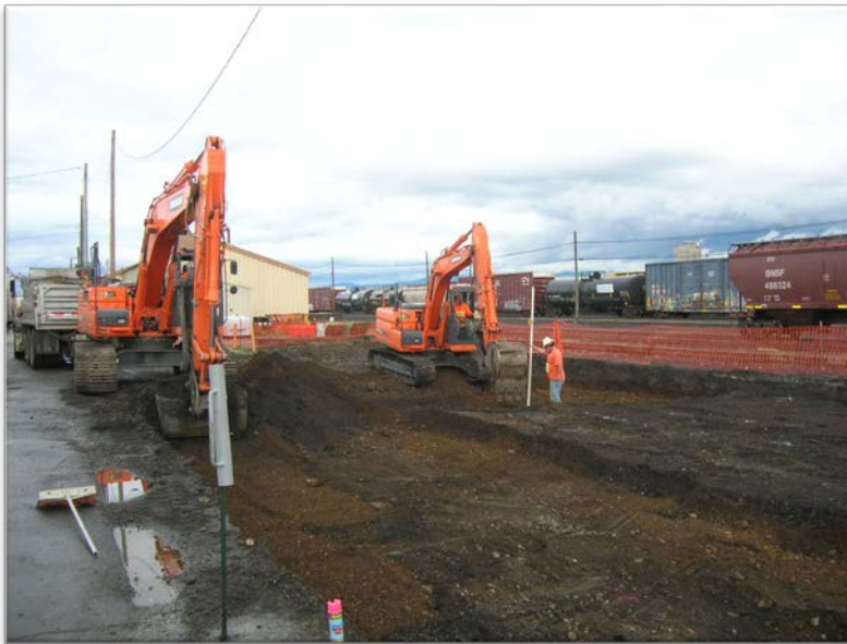
Photograph 4 – Over excavation - Looking to east.
