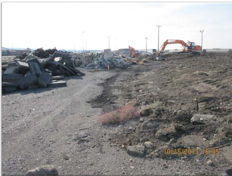
Photograph 4 –Rough grading and removal of large concrete debris.
