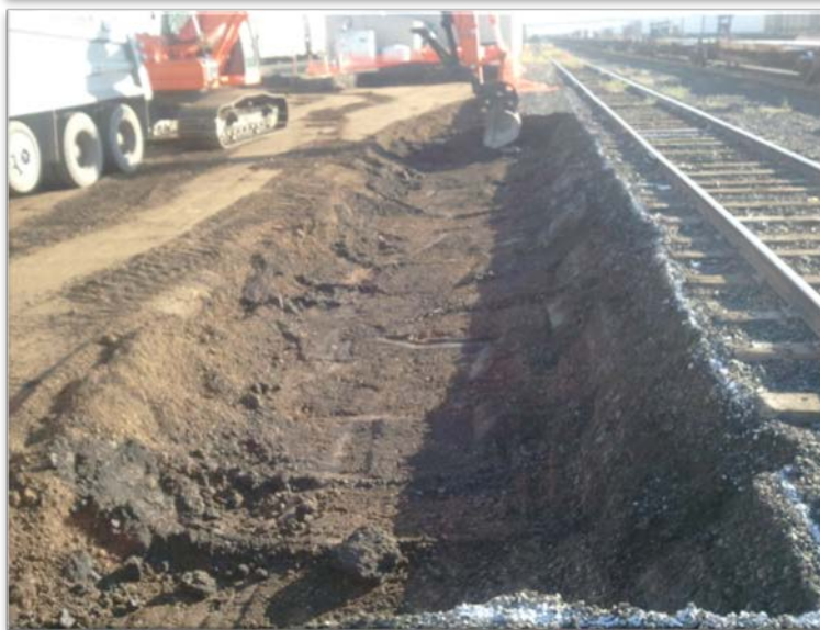
Photograph 8 – Over excavation on south side - Looking to east.
