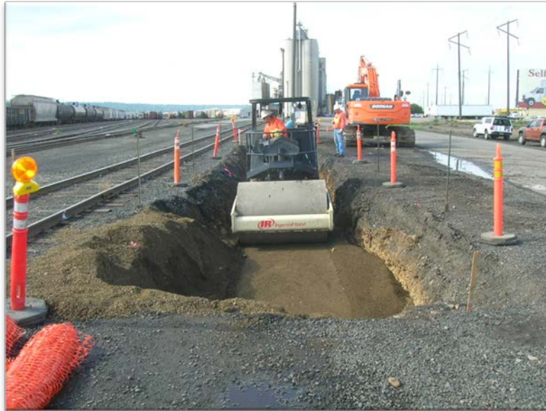
Photograph 9- Backfilling and compaction of west excavation - Looking to west.
