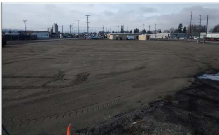
Photograph 10 – Completed cap – Looking to west.
