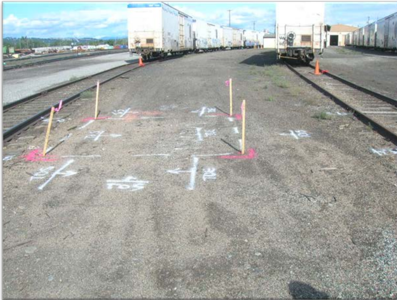
Photograph 1- Soil excavation control points - Looking to east.
