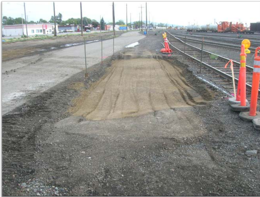
Photograph 7- Compaction of east excavation - Looking to east.
