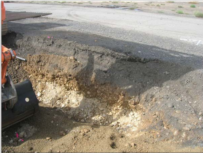
Photograph 3 – Soil excavation (east excavation) - Looking at north sidewall.
