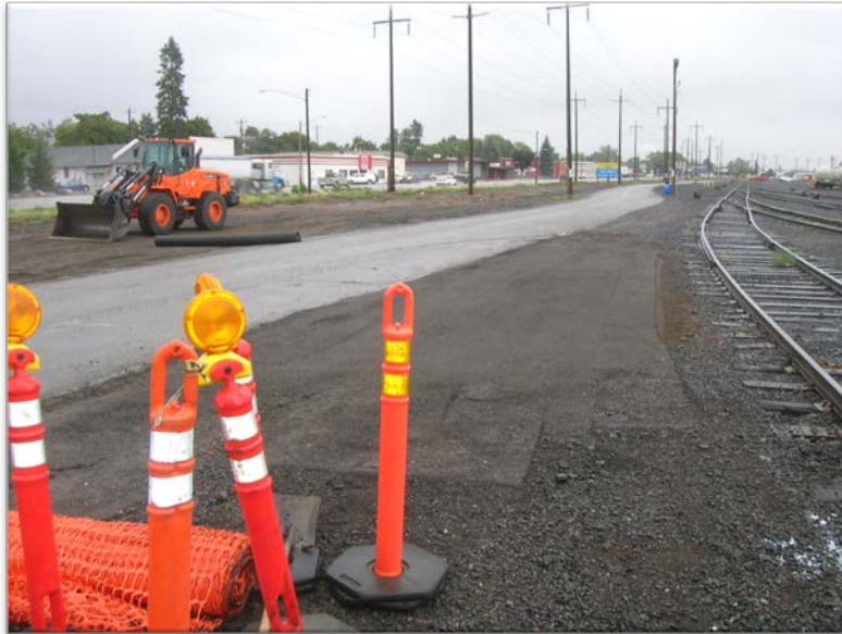
Photograph 11- Compacted CSTC (east excavation) - Looking to east.
