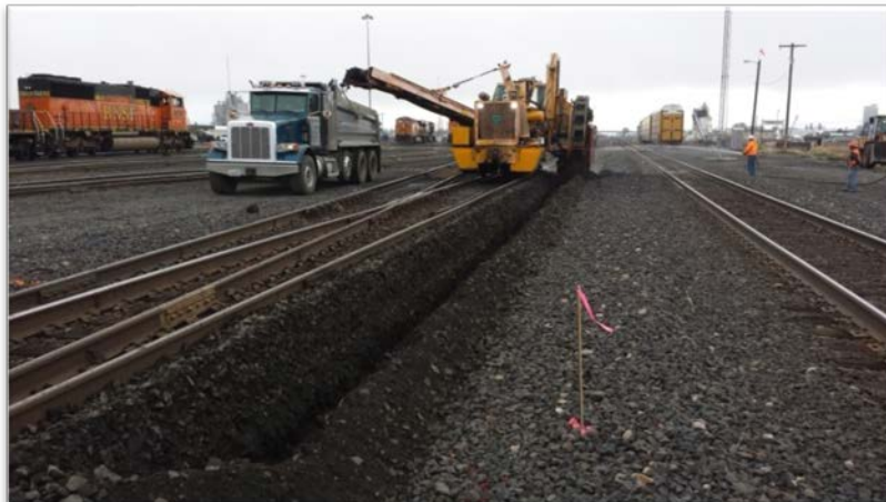
Photograph 4 – Undercutter - Looking to east.
