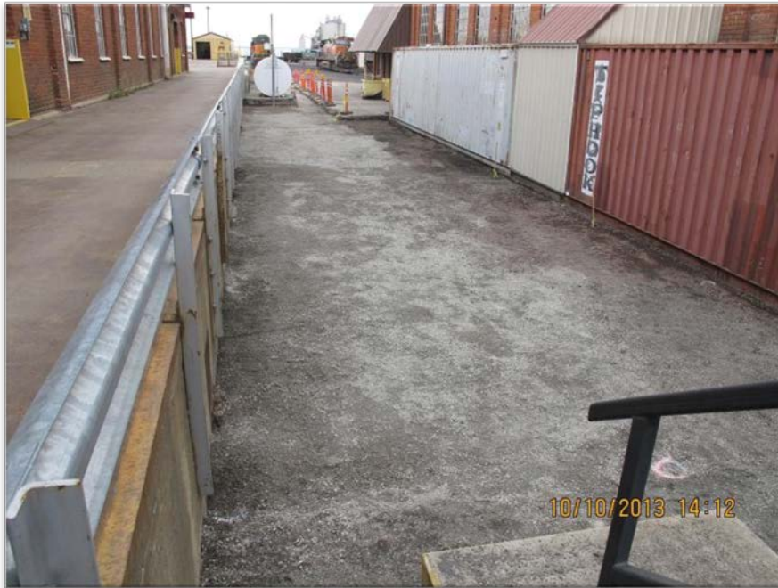
Photograph 3 – Subgrade - Looking to southwest.
