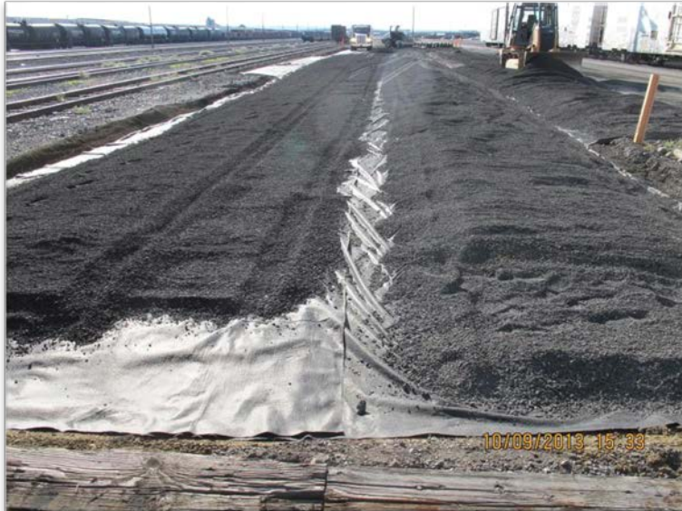
Photograph 9- Geotextile placement and CSTC cap - Looking to west.
