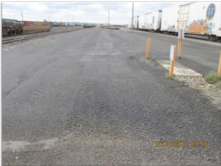
Photograph 10 – Compacted CSTC cap - Looking to west.
