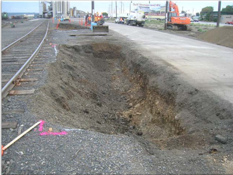
Photograph 5- Soil excavations - Looking to west.
