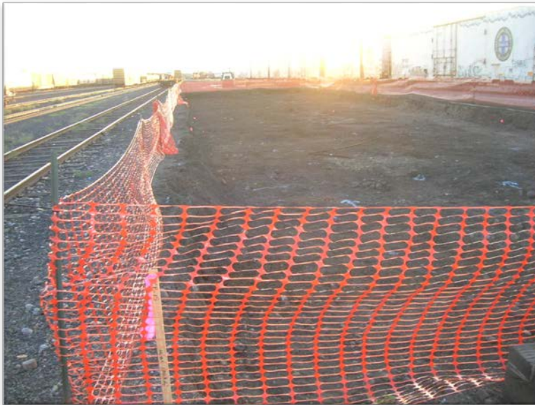
Photograph 2 – Initial soil excavation - Looking to west.
