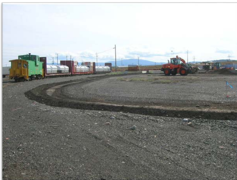
Photograph 2 – Berm construction for spoils stockpile.
