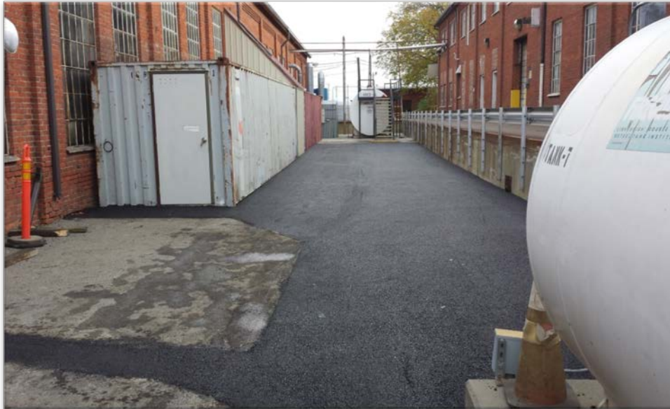
Photograph 7- Asphalt - Looking to northeast.
