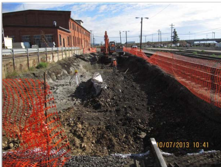
Photograph 2 – Soil excavation - Looking to northeast.
