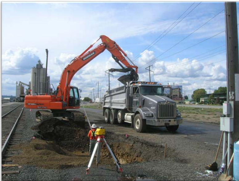
Photograph 4 – Soil excavation (east excavation) - Looking to west.
