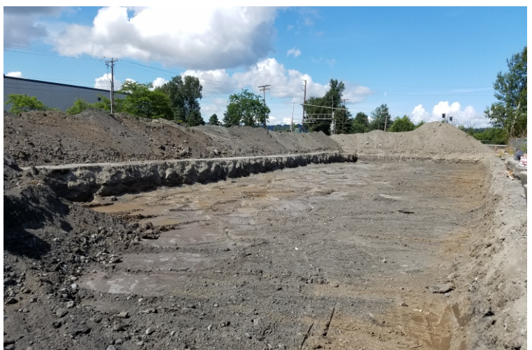
Photograph 06: Stormwater Vault Excavation
