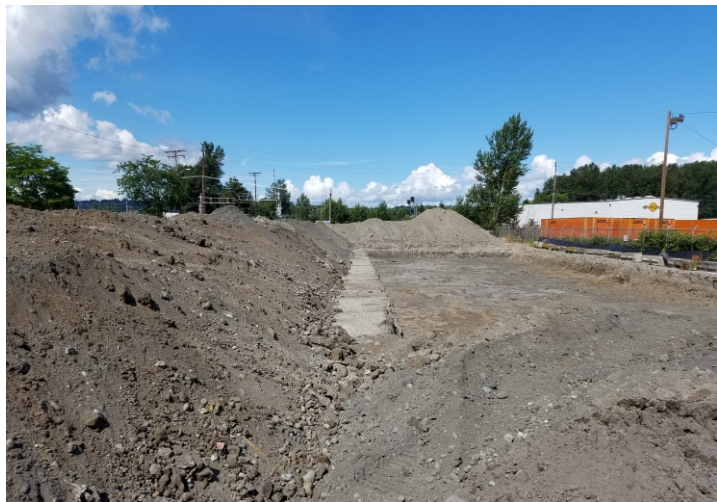
Photograph 05: Stormwater Vault Excavation
