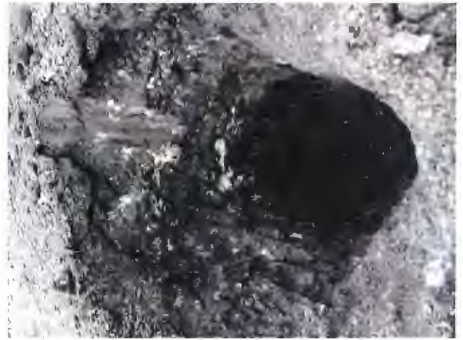
Example of Dross Material Near EX1
