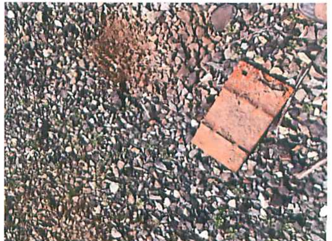
Rail joint near presumed MW3 location
