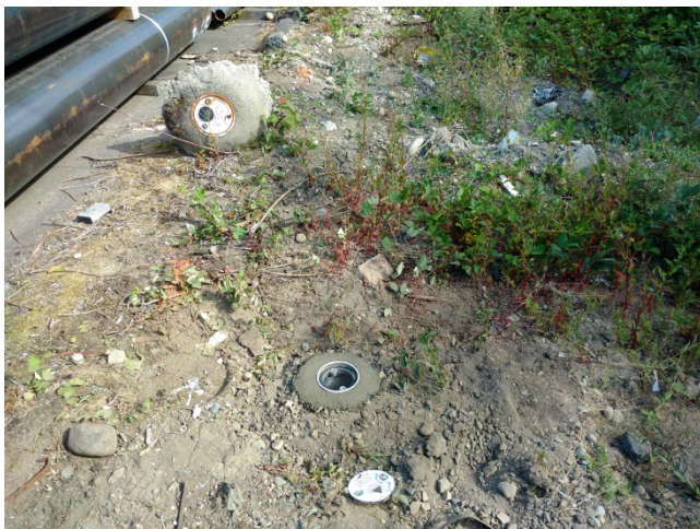
View of newly installed MW5A
