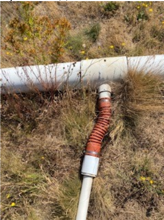
Repair at N-41 (1)
