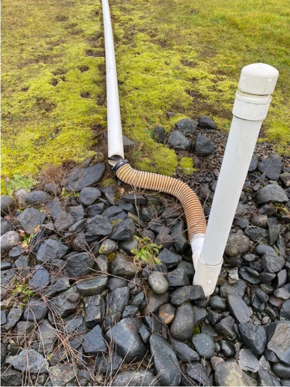
3" LFG Hose Replaced at N-57 (1)
