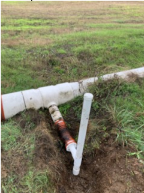
After repair at drain line near E-38
