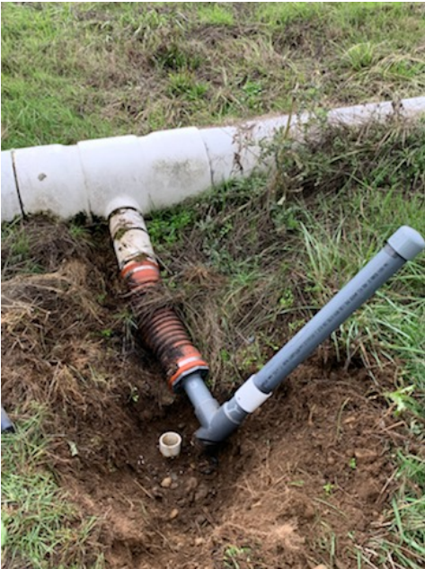
Before repair at drain line near E-38
