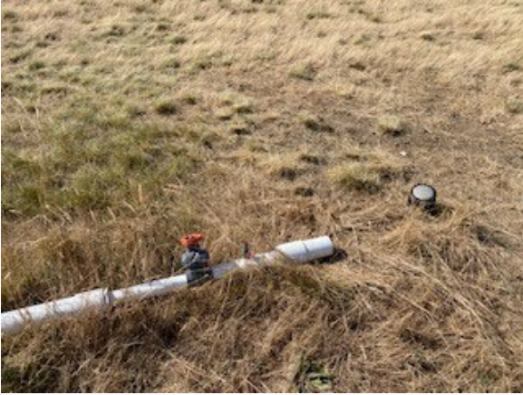
Repair at E-25 (1)
