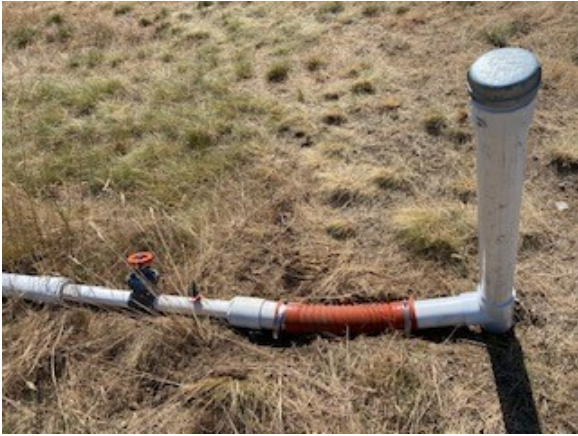
Repair at E-25 (2)
