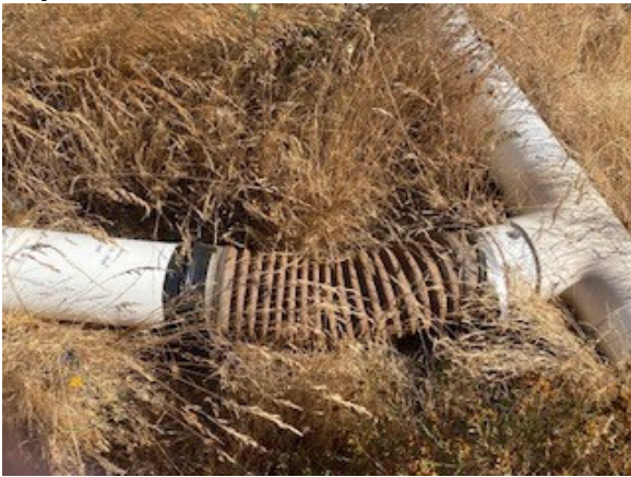
Repair at N-33 (2)
