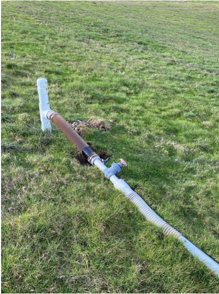
3" LFG Hose, 2" Valve Replaced at E-38 (1)
