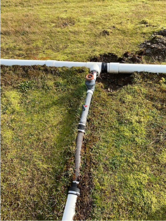
3" Tee and 3" LFG Hose Repaired at N-32 (1)
