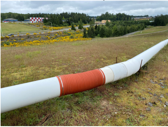
Installed 12"x3' Header Pipe at N-8 (1)
