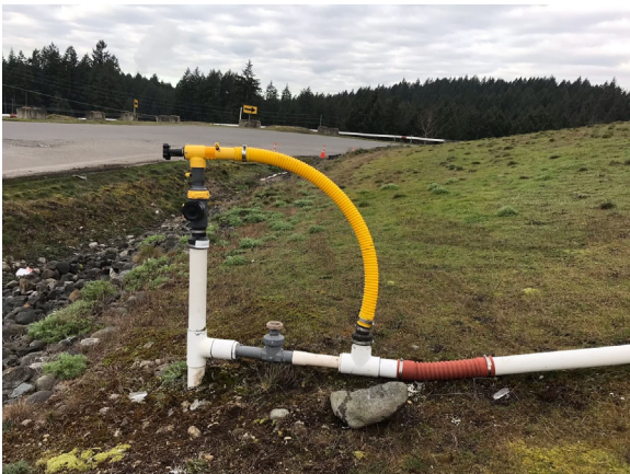
Replaced 3" LFG Hose at N -10 No figure available.
