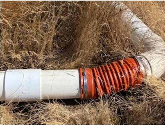
Repair at N-33 (1)
