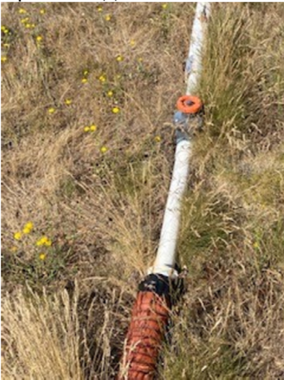
Repair at N-41 (2)
