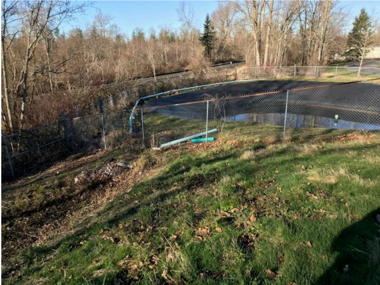
Photo 13: Leachate storage lagoon located on northwest corner of property
