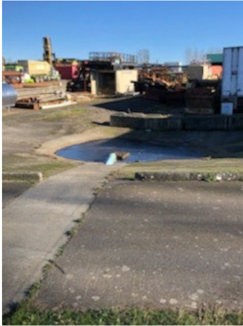
Photo 9: Stormwater collection basin on northern portion of closed ash landfill
