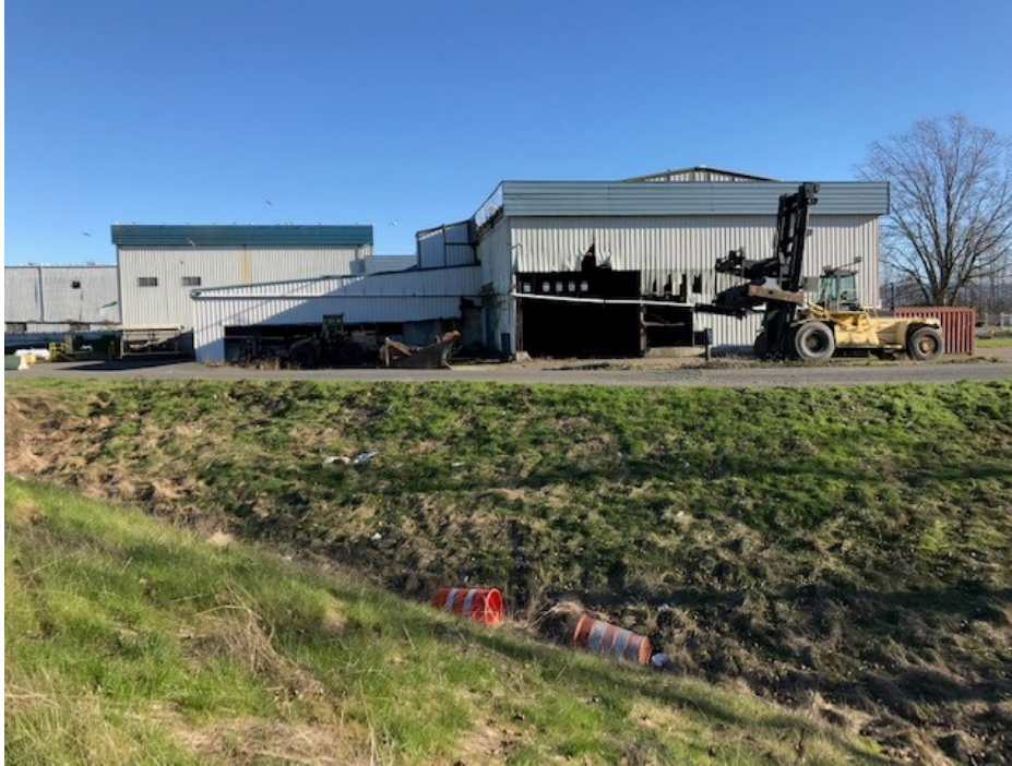
Photo 1: Waste transfer station located south of closed ash landfill, view to south
