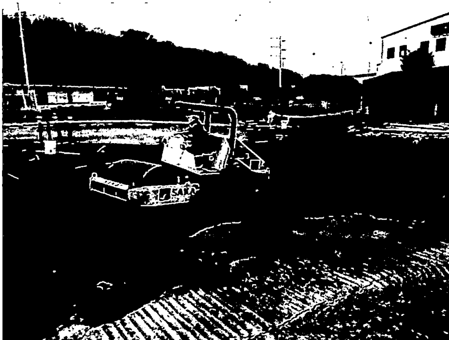
Photo 15: UST cavity being compacted (looking west)
