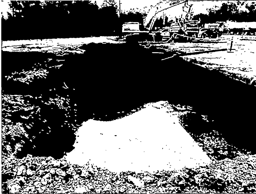
Photo 11: The site is tidally influenced, filling the UST cavity overnight after removal (looking south)
