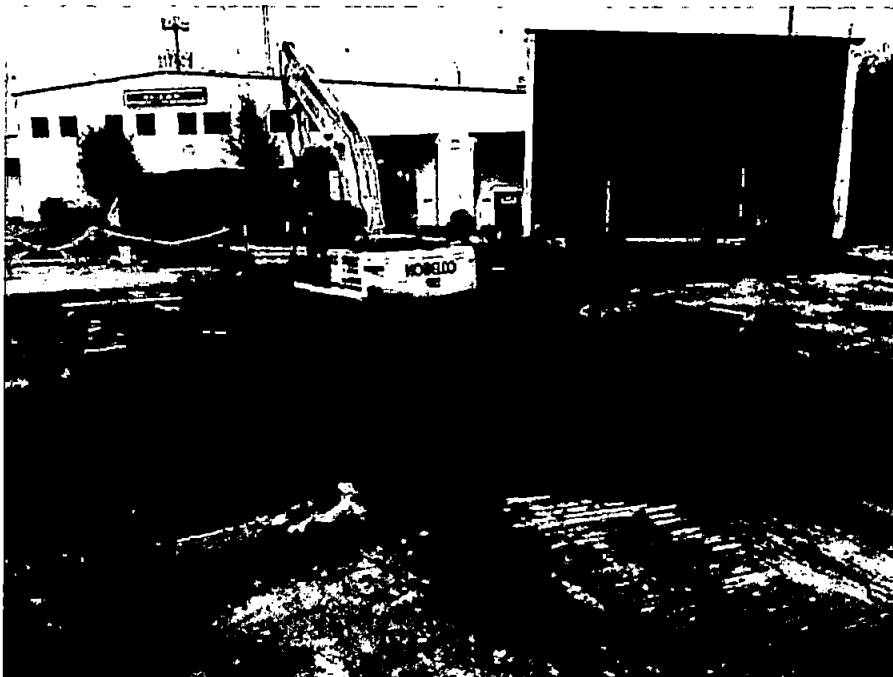
Photo 14: UST cavity being backfilled and compacted.
