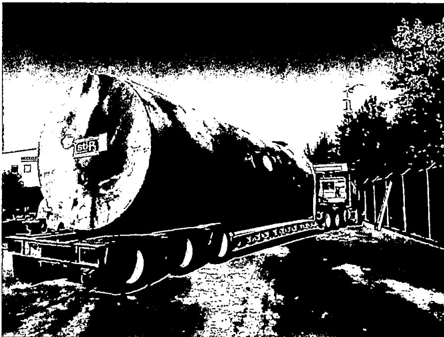
Photo 10: 20,000-gallon diesel UST loaded for transport to recycling yard.
