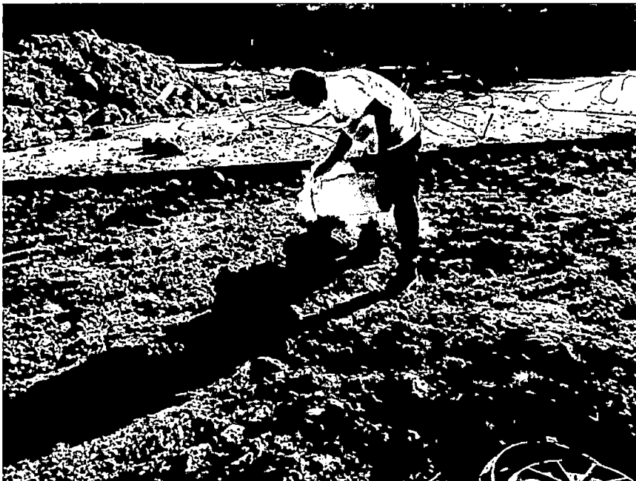
Photo 4: One day prior to removal, dry ice is added to the UST (Wyser).
