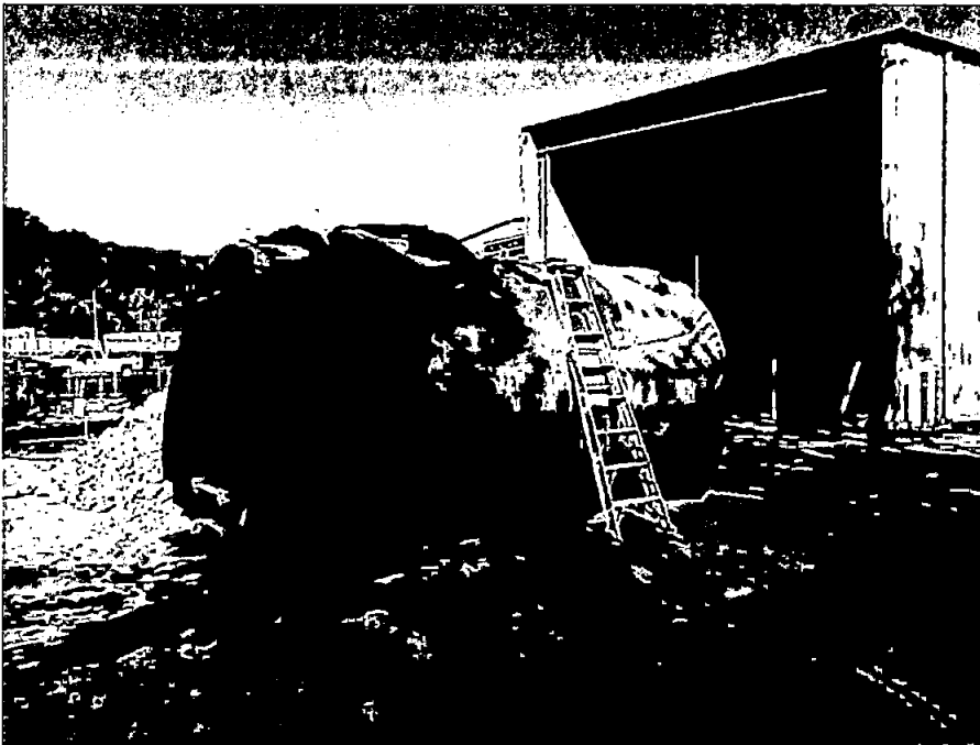
Photo 6: Gasoline UST after removal and being prepared for transport.
