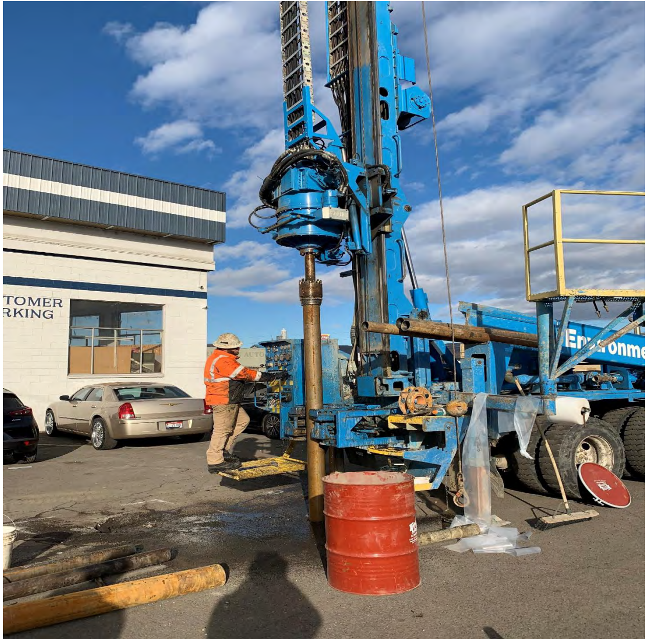
Photograph 11 – Drillers advancing sonic drilling rods at soil boring SB3 (facing northeast)
