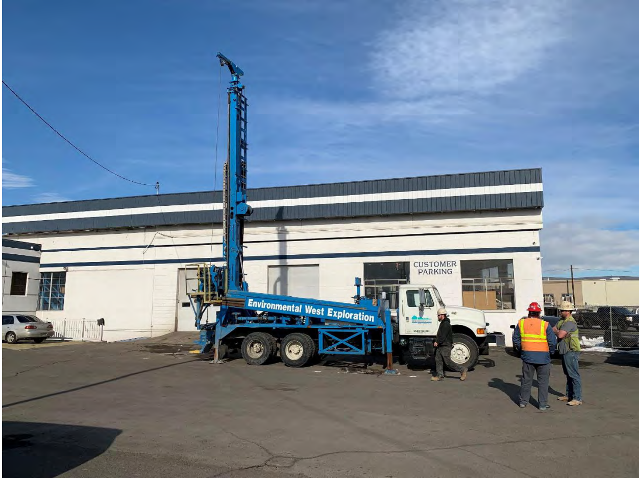
Photograph 7 – View of sonic drill rig prepared to begin drilling at soil boring SB1 on Tuesday, February 1, 2022 (facing north).
