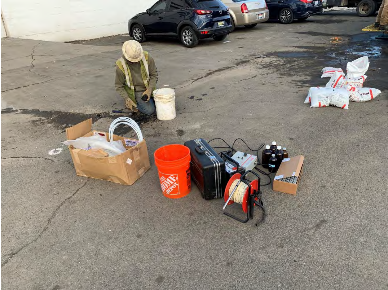
Photograph 13 – Driller’s helper replacing the asphalt patch at soil boring SB1.
