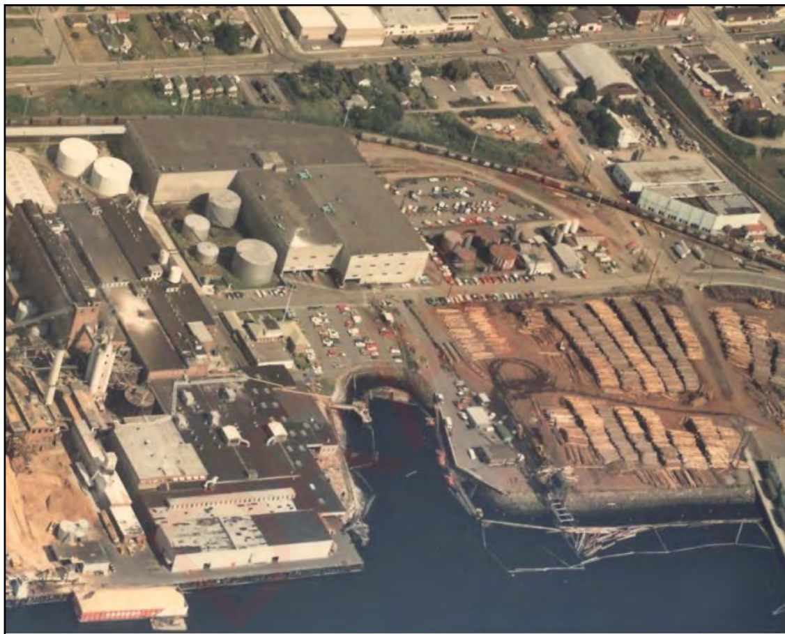
Figure 11. A 1977 aerial photograph of the project area (Washington Department of Ecology 2021).
