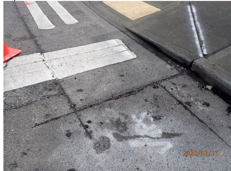
Following sampling activities, borings were backfilled and sealed at the surface.
