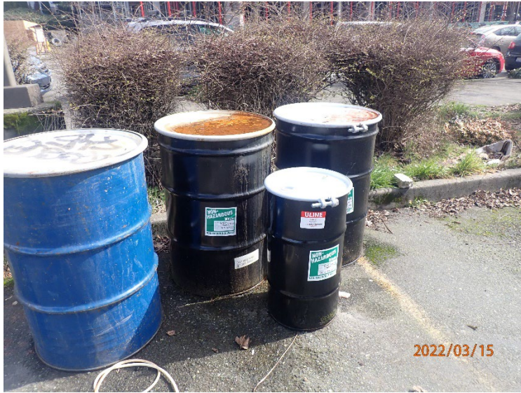
Investigation derived waste (soil and water) was placed in drums and left on site pending receipt of laboratory results.
