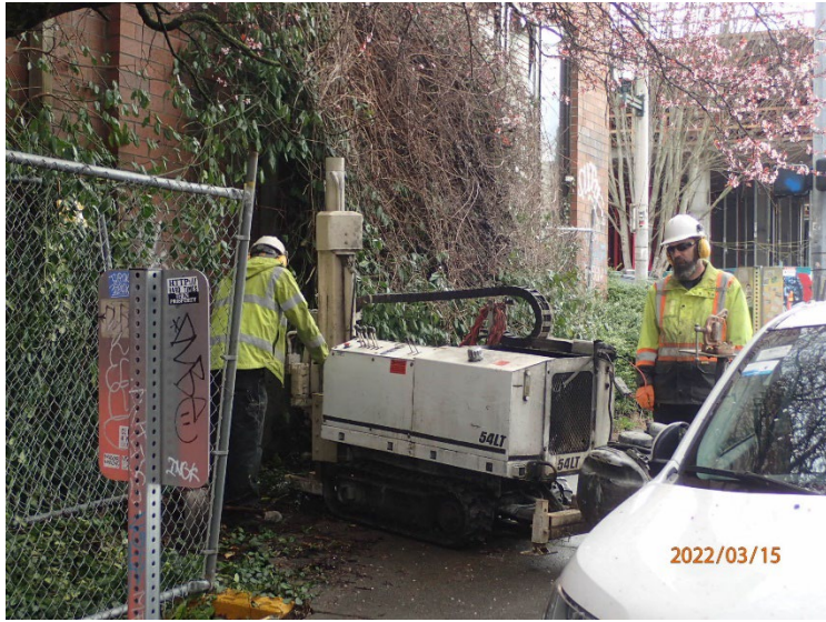
View east of drill rig set up on boring location EB01.
