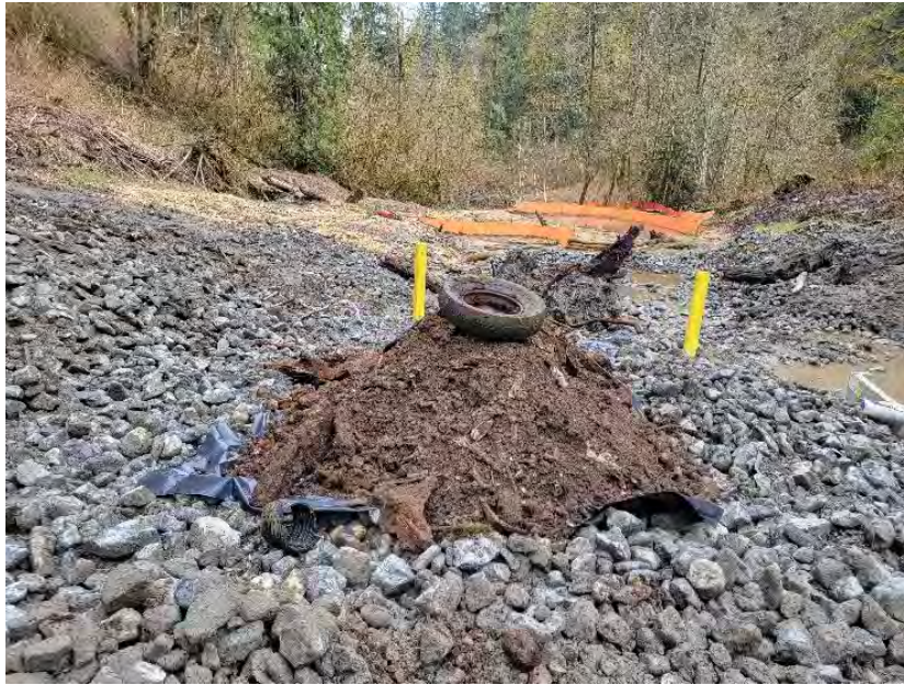
Photograph 13. Lined stockpile of excavated metal debris, soil, and other debris.
