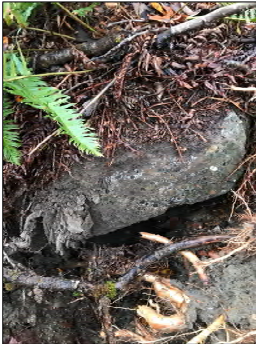
Photograph 4. One piece of concrete at ground surface.
