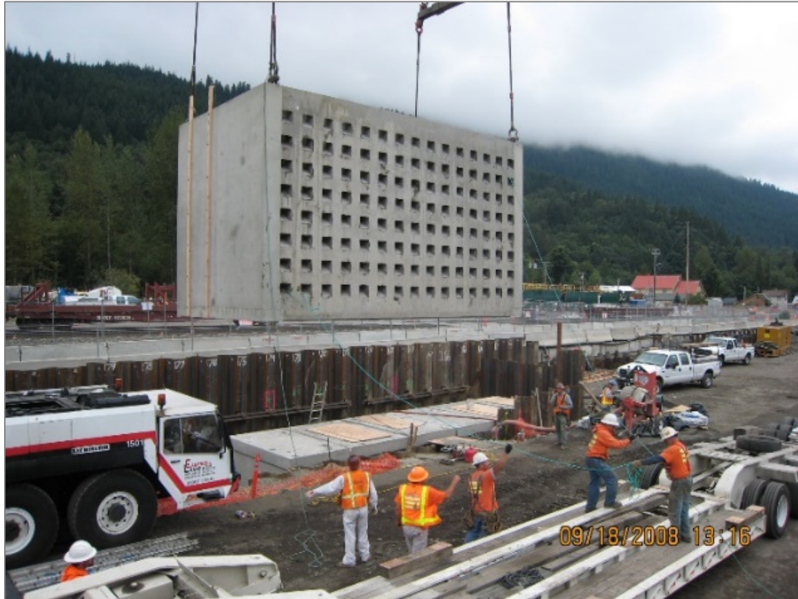
Installation of HCC treatment gate system, 2008
