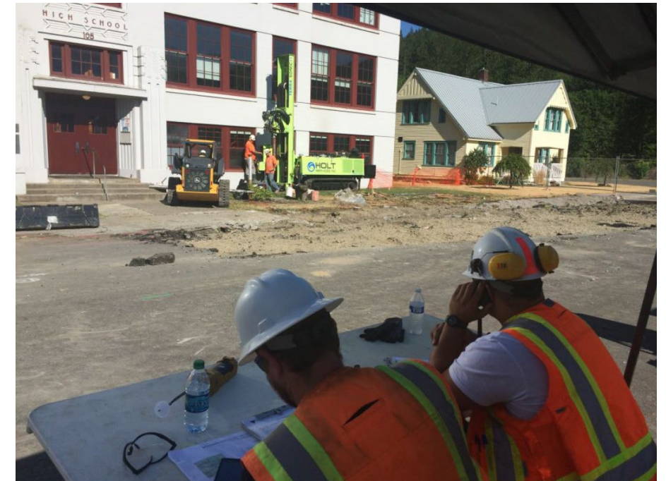
Hot water flushing system well installation, 2015
