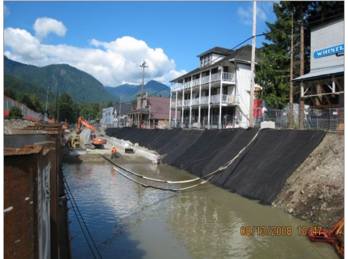
HCC System construction on Railroad Avenue, 2008
