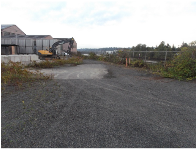
Photograph 1. Overview of the SB3/SB4 Upland Interim Action area. Photo viewing south.
