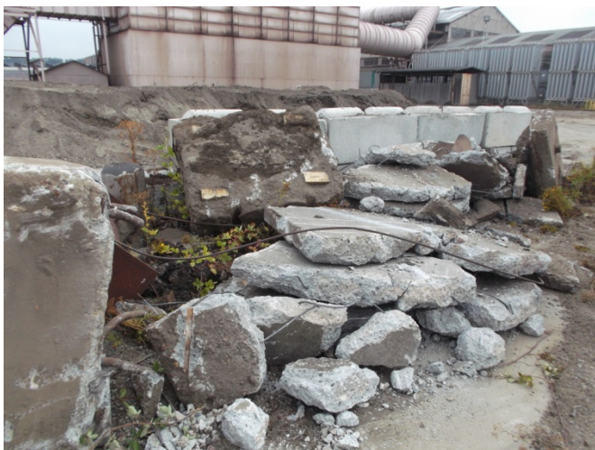
Photograph 5. Example of concrete rubble removed from SB3/SB4 excavation. Photo viewing southeast.
