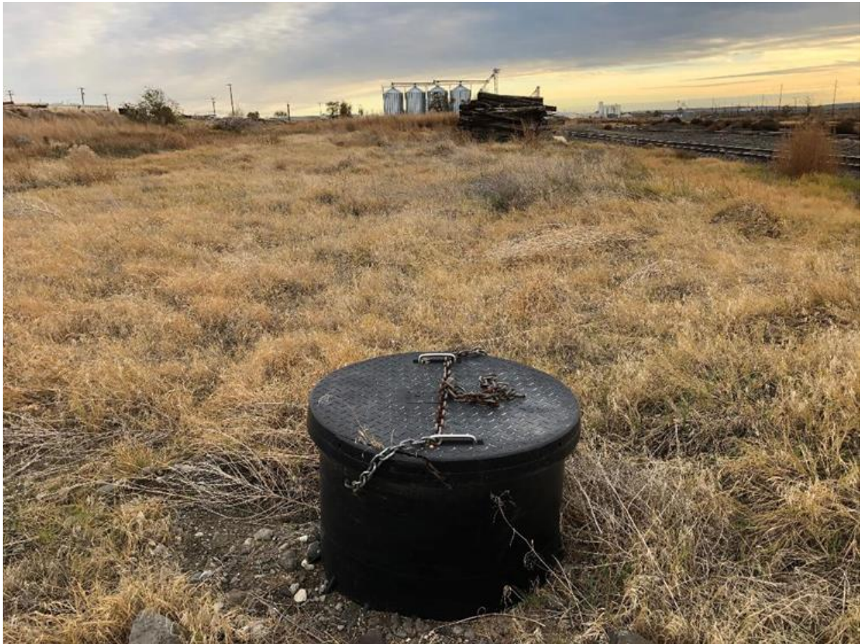
Photo 2: Former dewatering sump and vicinity of barrier wall – from the north
