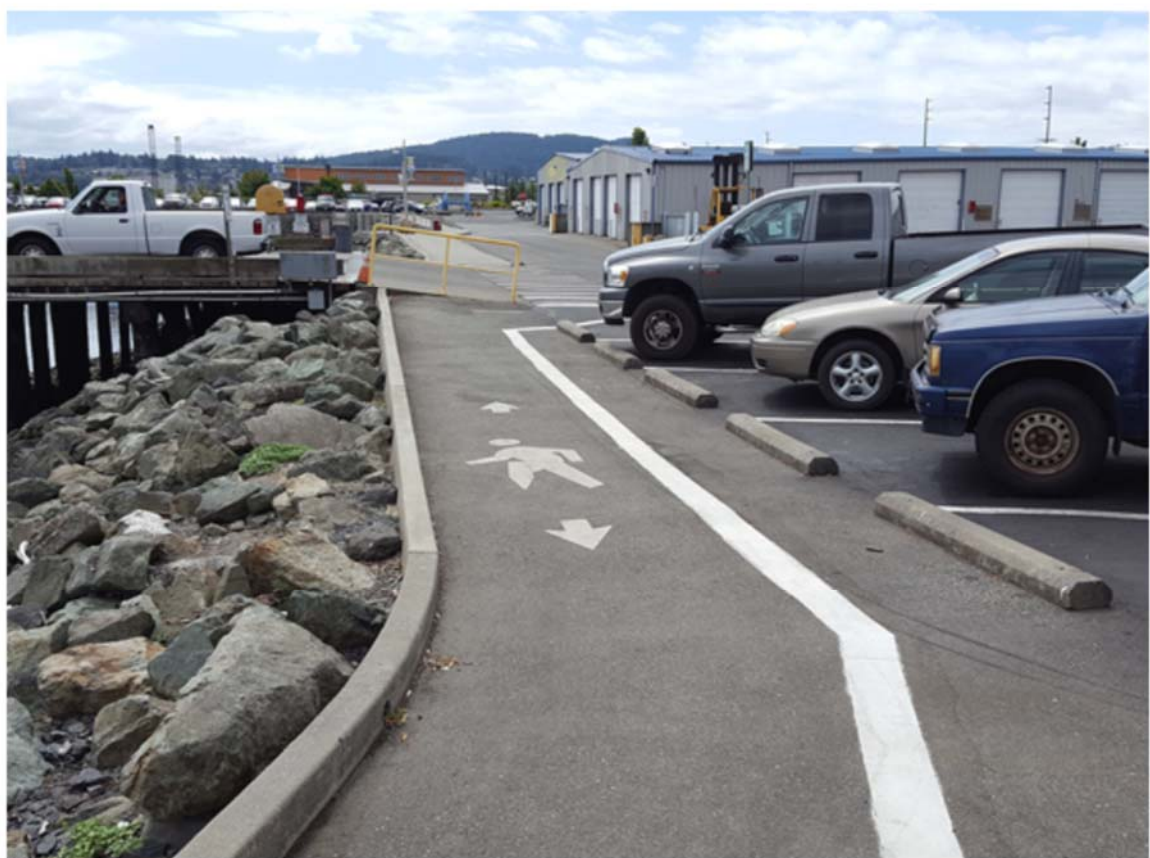
Photo A8: Protective asphalt barrier east of the utilities looking south (see Figure 1).
