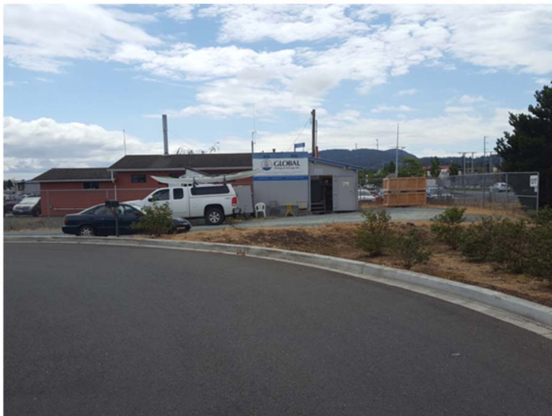
Photo B8: Protective crush gravel and topsoil barriers with fenced enclosure north of the office building (see Figure 2)
