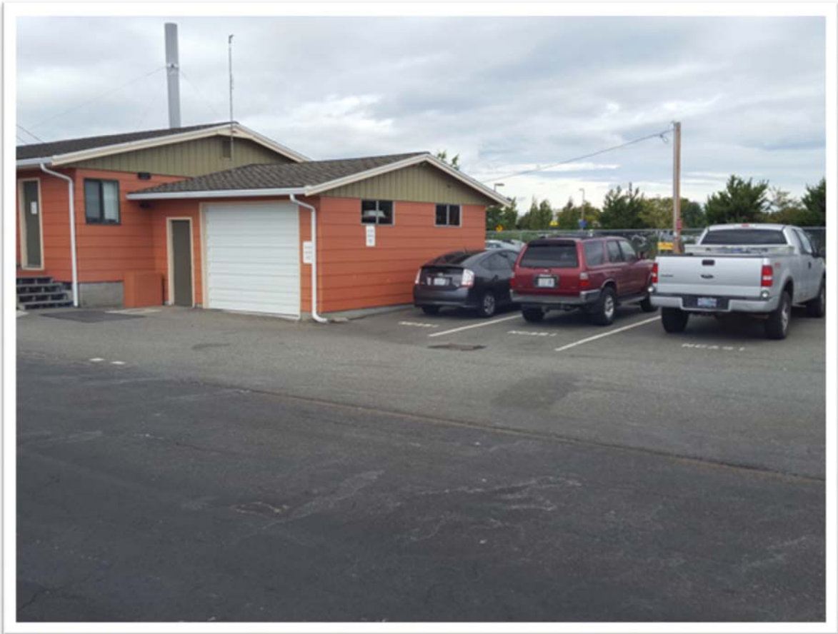
Photo B5: Protective asphalt barrier looking northwest from Control Point B1 (see Figure 2)
