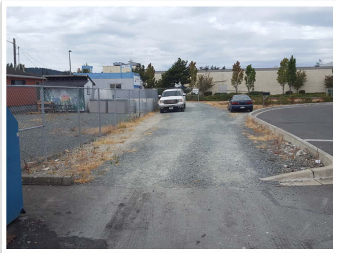
Photo B6: Protective crush gravel and topsoil barriers with fenced enclosure north of the office building (see Figure 2)
