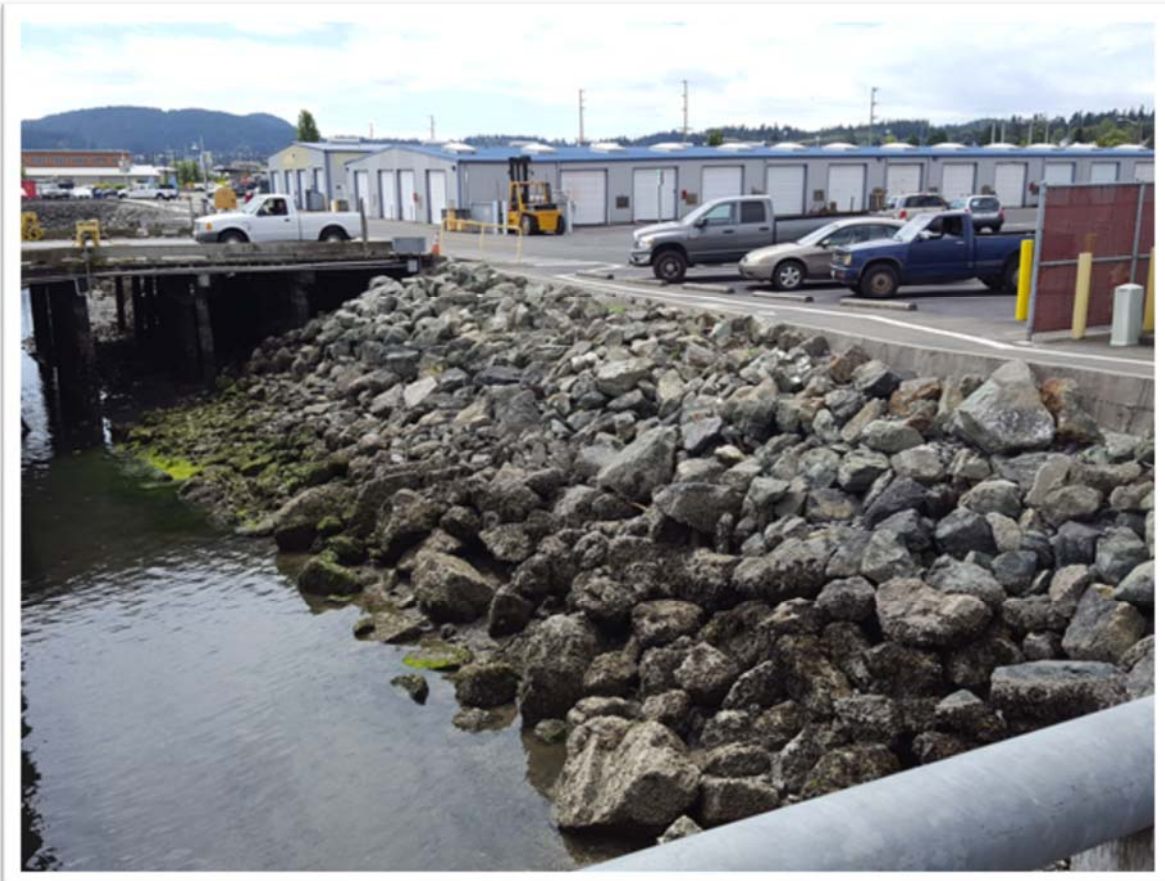
Photo A5: Protective stone revetment barrier looking southwest (see Figure 1).
