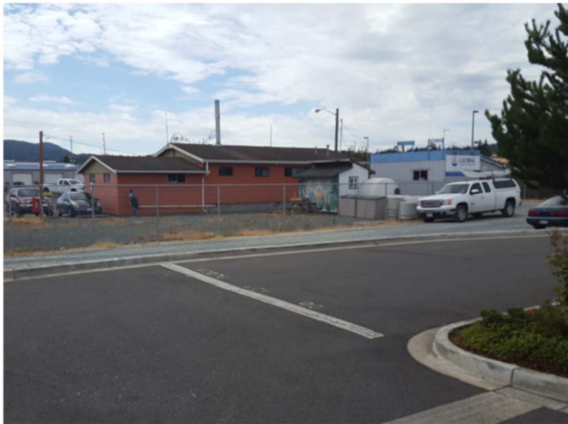
Photo B7: Protective crush gravel, topsoil and asphalt barriers north of the office building (see Figure 2)
