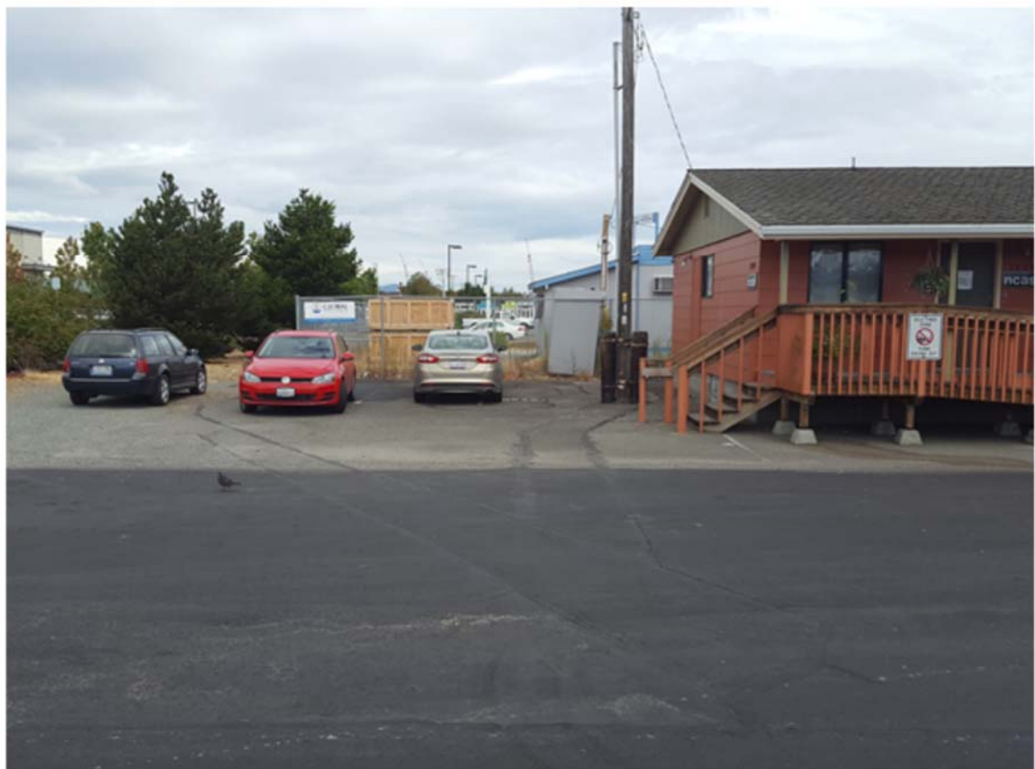
Photo B4: Protective asphalt barrier south of the office building (see Figure 2)
