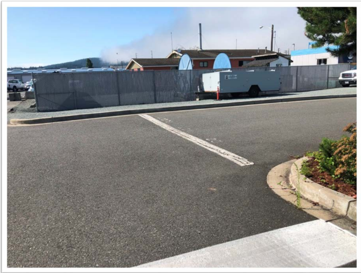
Photo B7: Protective crush gravel, topsoil and asphalt barriers north of the office building (see Figure 2)
