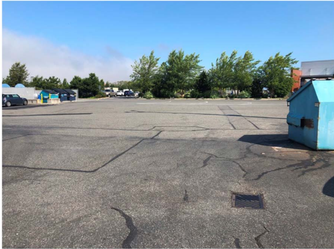
Photo A3: Protective asphalt barrier looking north (see Figure 1).
