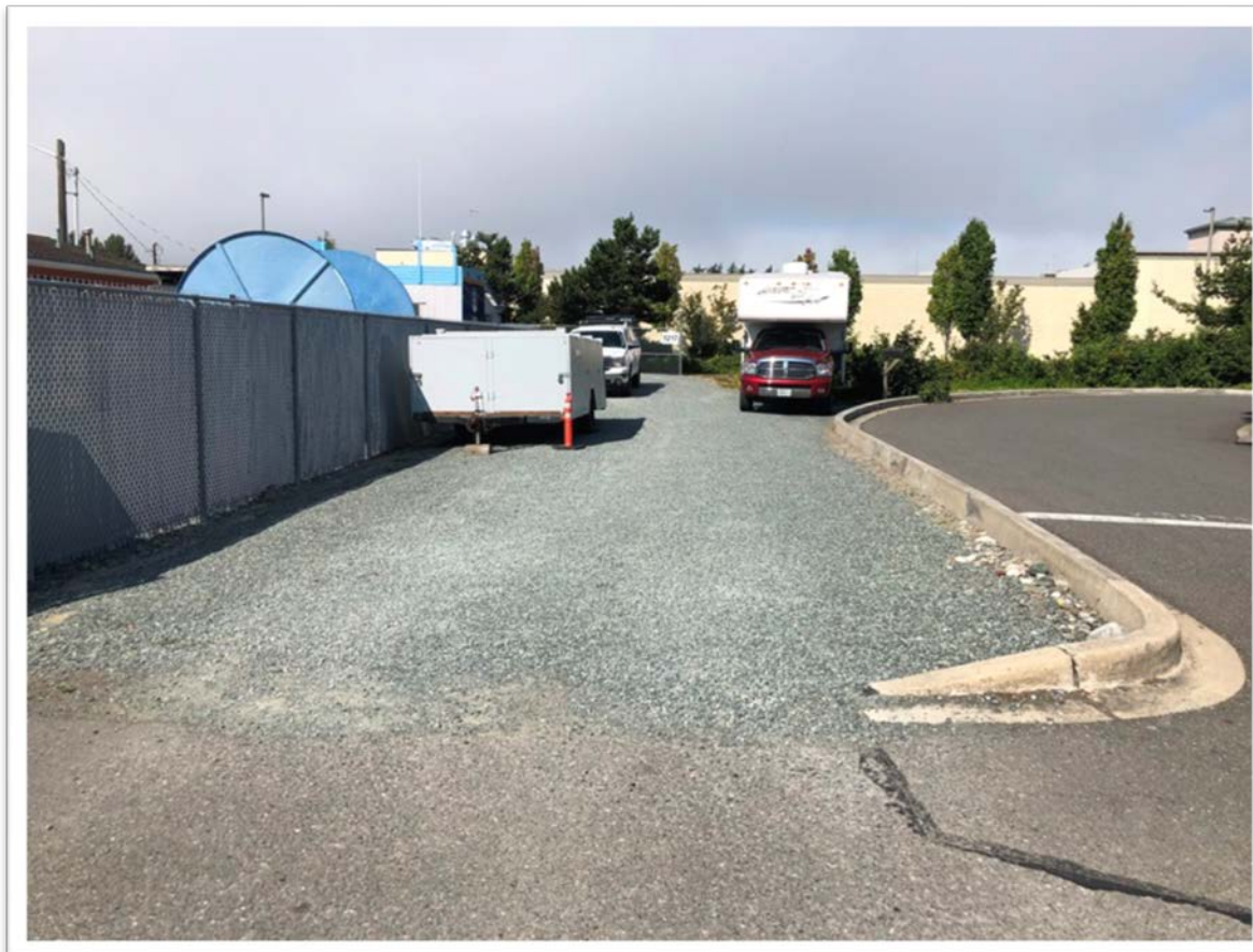
Photo B6: Protective crush gravel and topsoil barriers with fenced enclosure north of the office building (see Figure 2)
