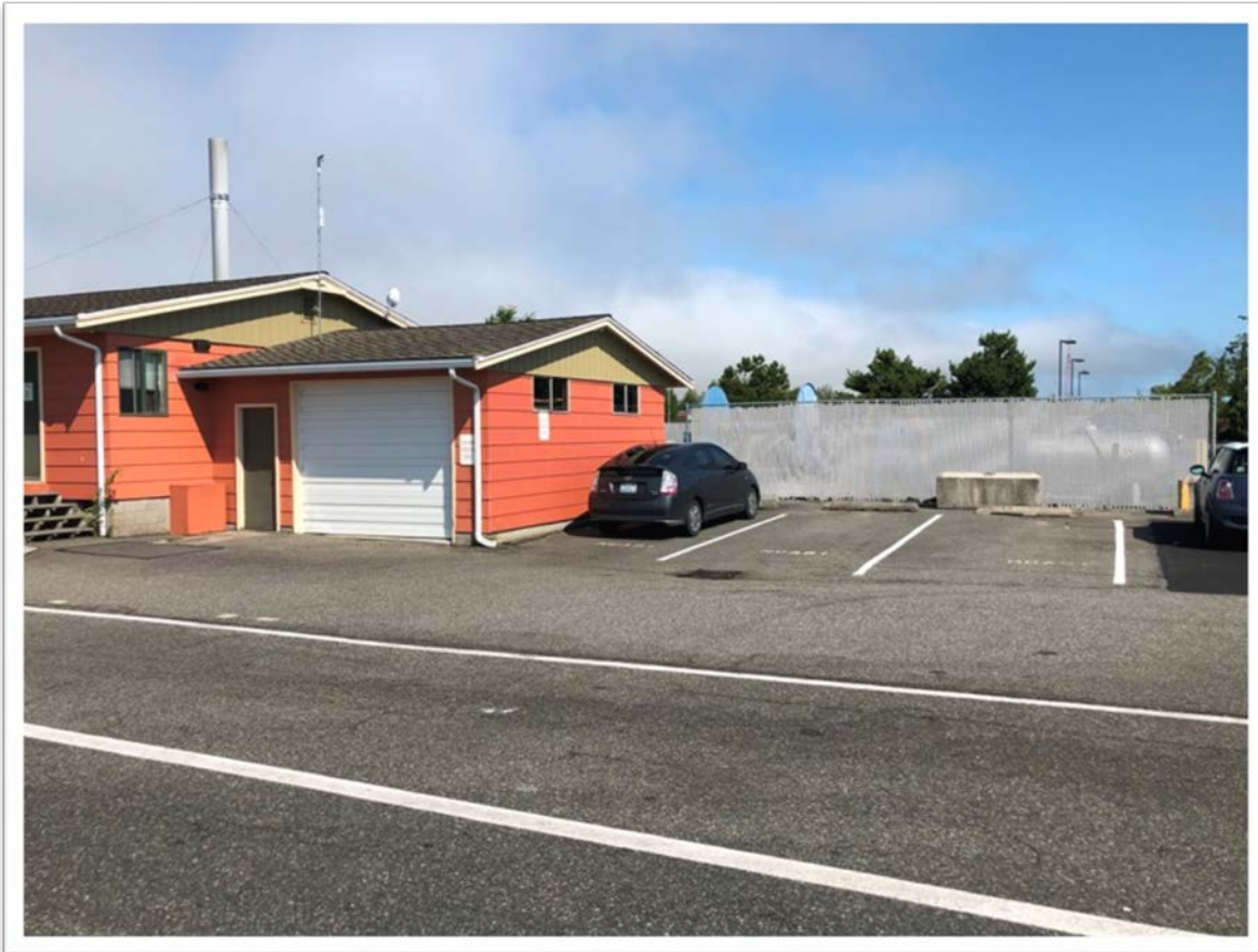
Photo B5: Protective asphalt barrier looking northwest from Control Point B1 (see Figure 2)
