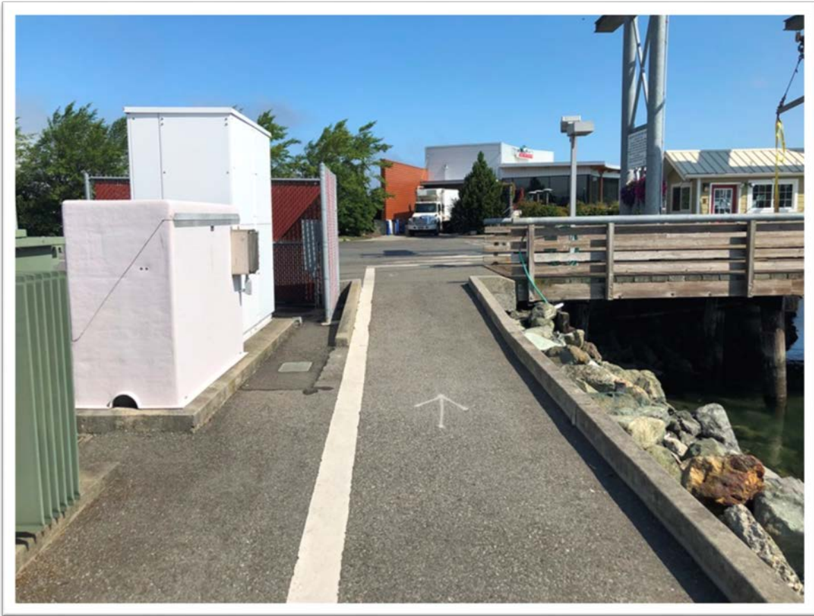
Photo A7: Protective asphalt barrier east of the utilities looking north (see Figure 1).
