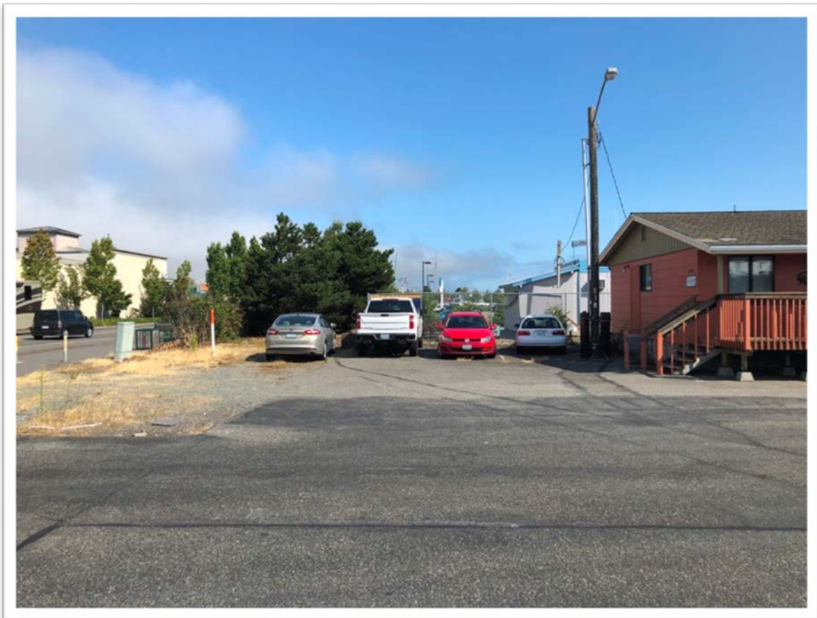
Photo B4: Protective asphalt barrier south of the office building (see Figure 2)
