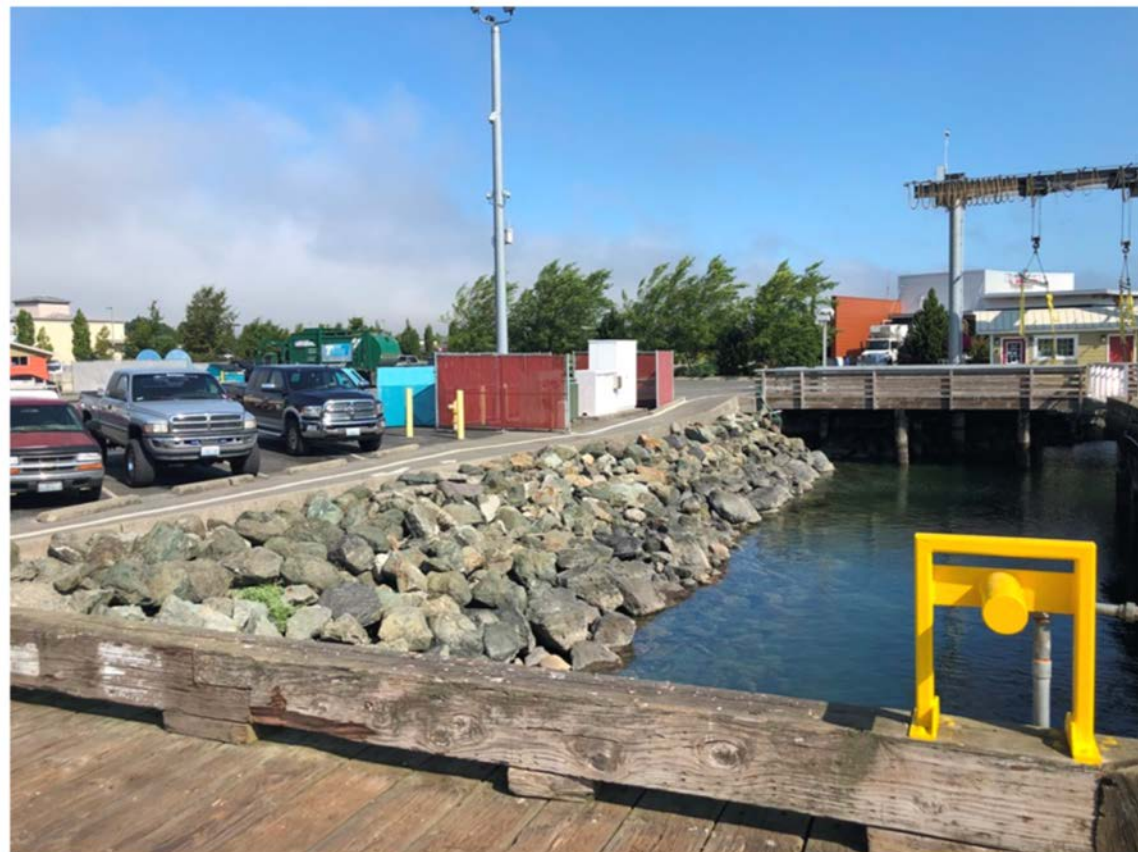
Photo A4: Protective stone revetment barrier looking northwest (see Figure 1).
