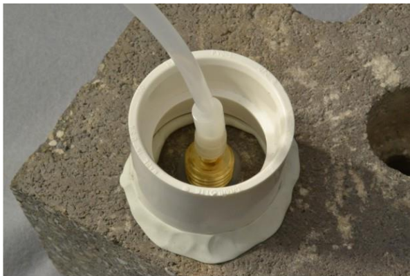
Figure 6. Water dam used for leak detection
