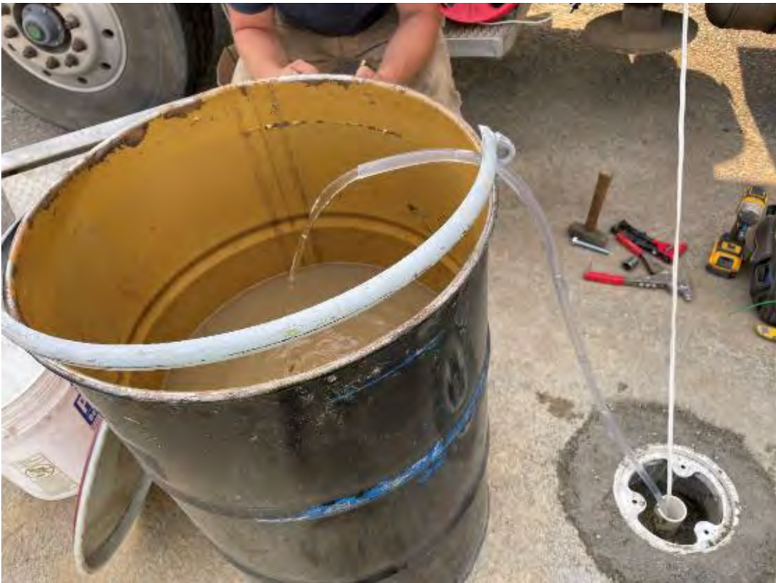
Photo 8. Developing MW-7D.
