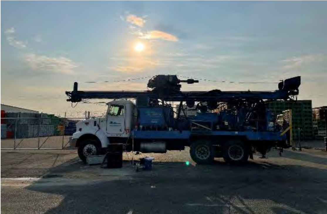
Photo 7. Environmental West sonic drill rig – developing MW-6D
