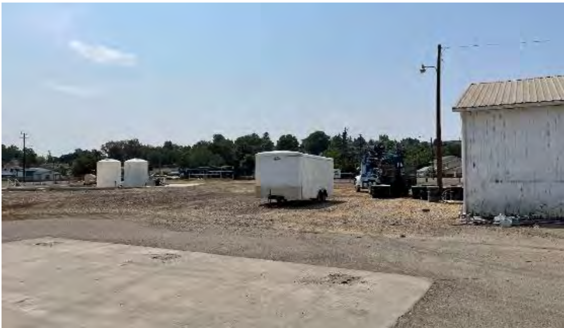
Photo 2. Temporary onsite storage of product water from monitoring well installations – south-east of storage building.
