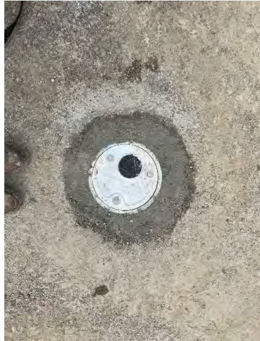
Photo 6. Monitoring wells completed flush to grade.
