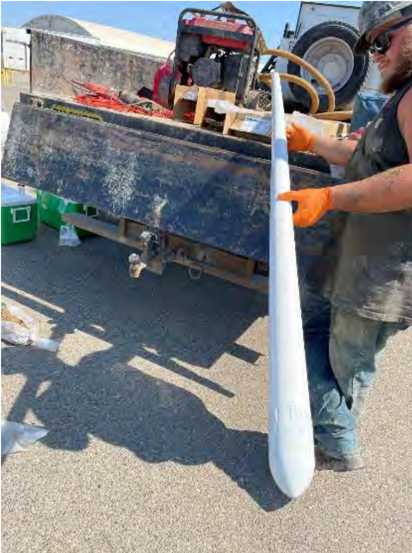
Photo 3. Well screen: 10-ft interval, 2-inch diameter, 0.010-inch slot Schedule 40 PVC with flush threaded bottom caps.
