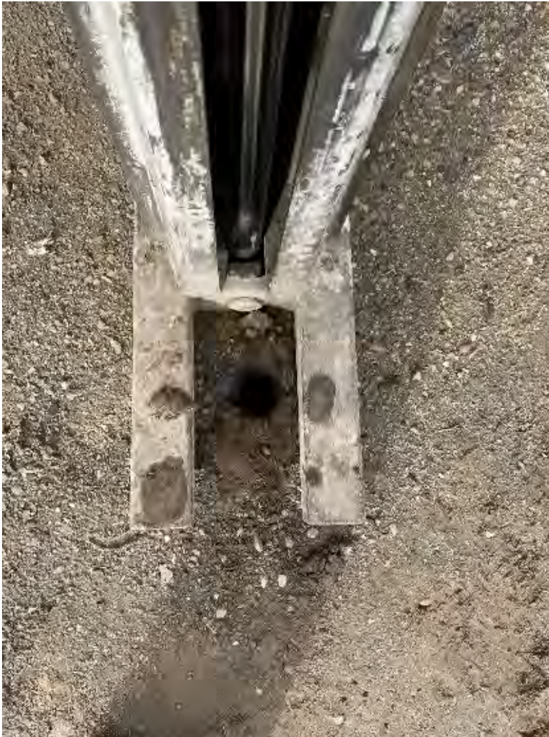
Photo 9. GeoProbe borehole, prior to backfilling.
