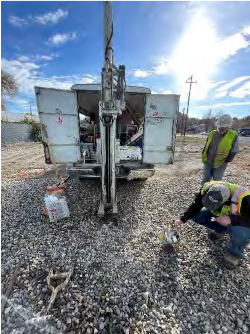
Photo 15. Collecting soil vapor intrusion sample VI2.5-02 (sample collected at 4-ft below ground surface).
