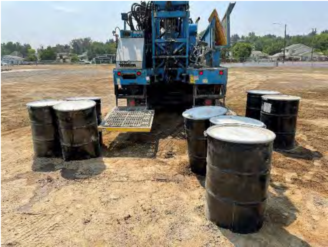
Photo 1. Temporary onsite storage of product water from monitoring well installations.
