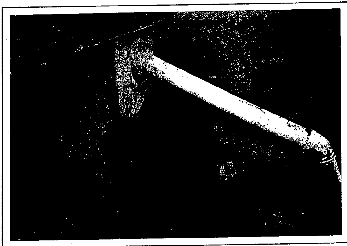
Plate 2. Patch Repair on Discharge Pipe Below O/W Separator:
