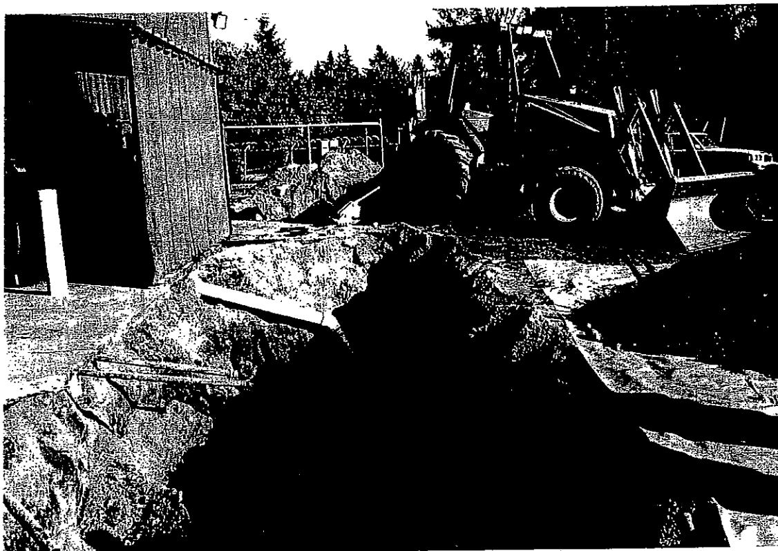
Plate 3. Excavation 2, after Removing (2)-2,000-g Gasoline USTs. O/W Discharge Pipe at NE End of Excavation. (View to NE).
