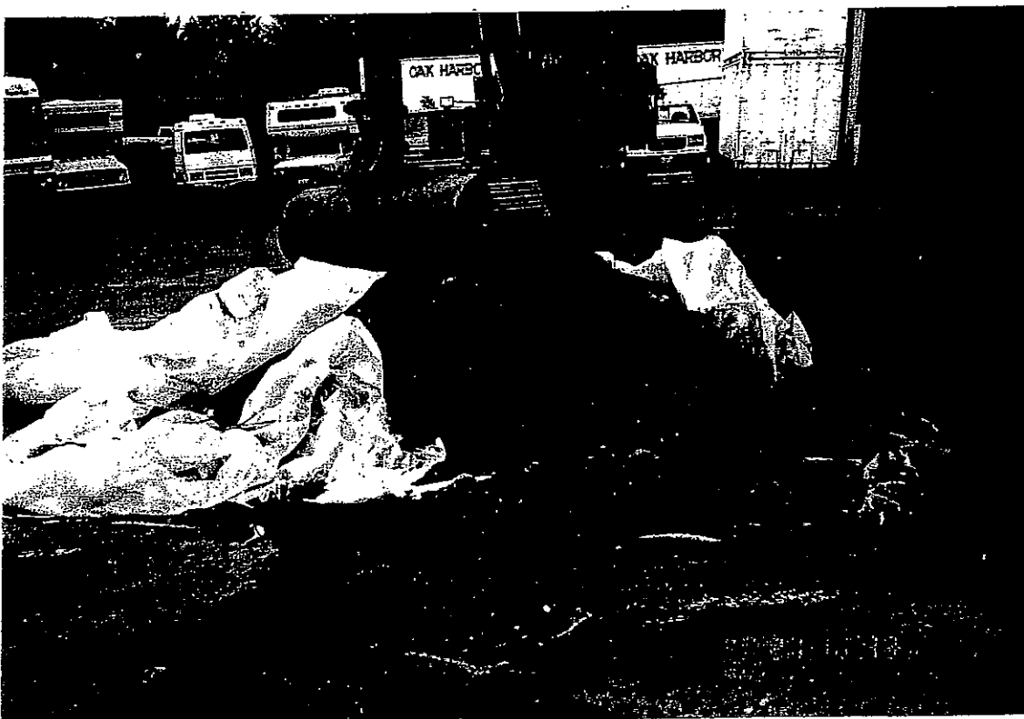
Plate 4. Contaminated Soil from Below the O/W Separator. Note 1,000-g Waste Oil Tank in Background.
