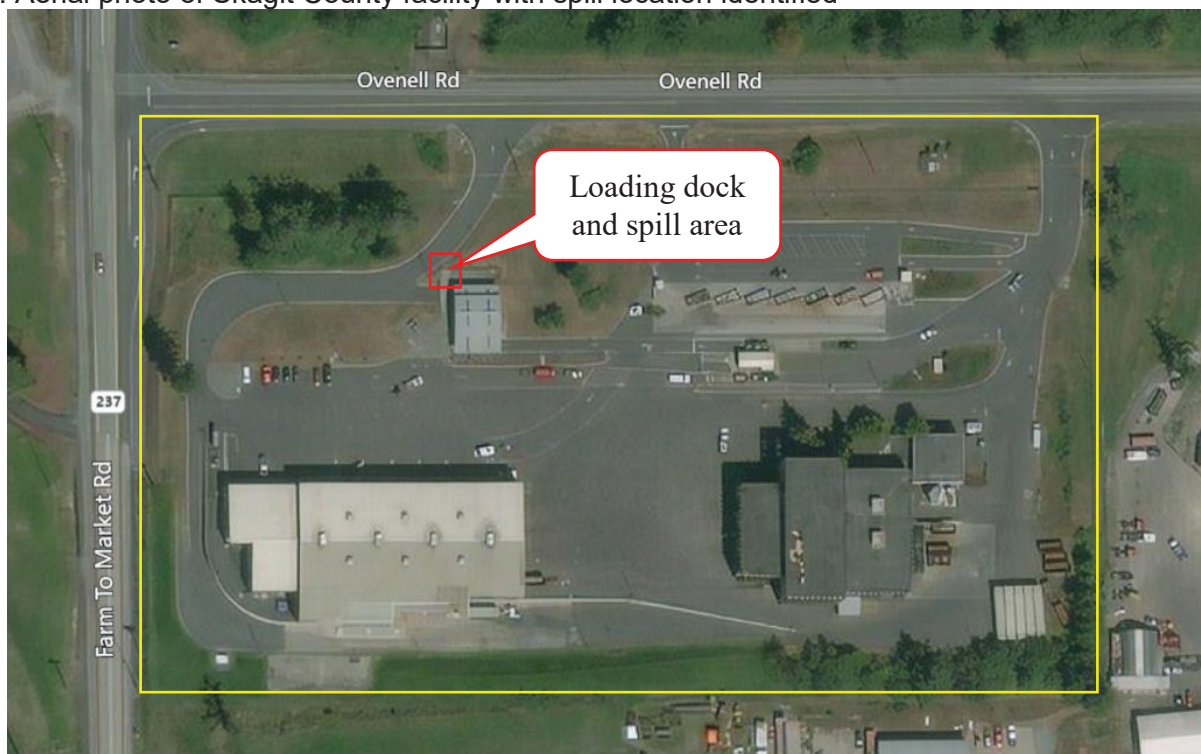
Figure 1: Aerial photo of Skagit County facility with spill location identified
