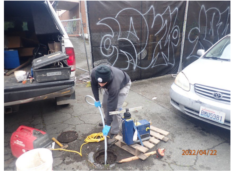
Well MW-8 being re-developed.
